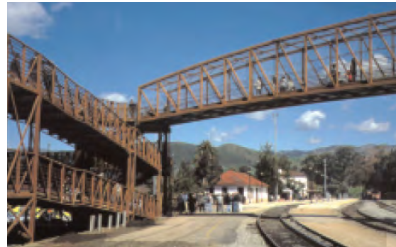
Trail-Rail Overcrossing, San Luis Obispo, CA
