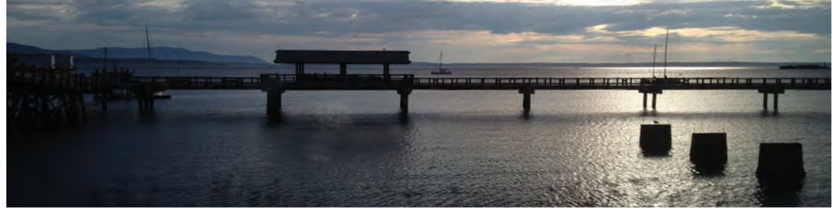
Interurban Trail, Overwater Section: Taylor Dock. Bellingham, WA.
