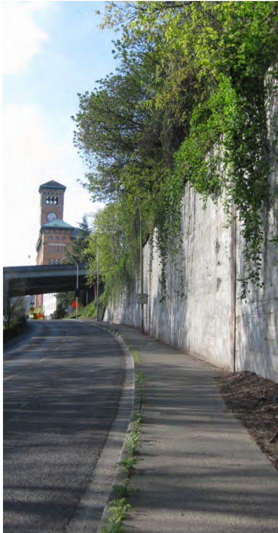
Existing Stadium Way Wall.
