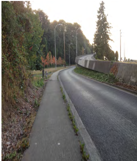
Schuster Parkway, Existing Approach to Garfield Gulch and Ruston Way Overpass.
