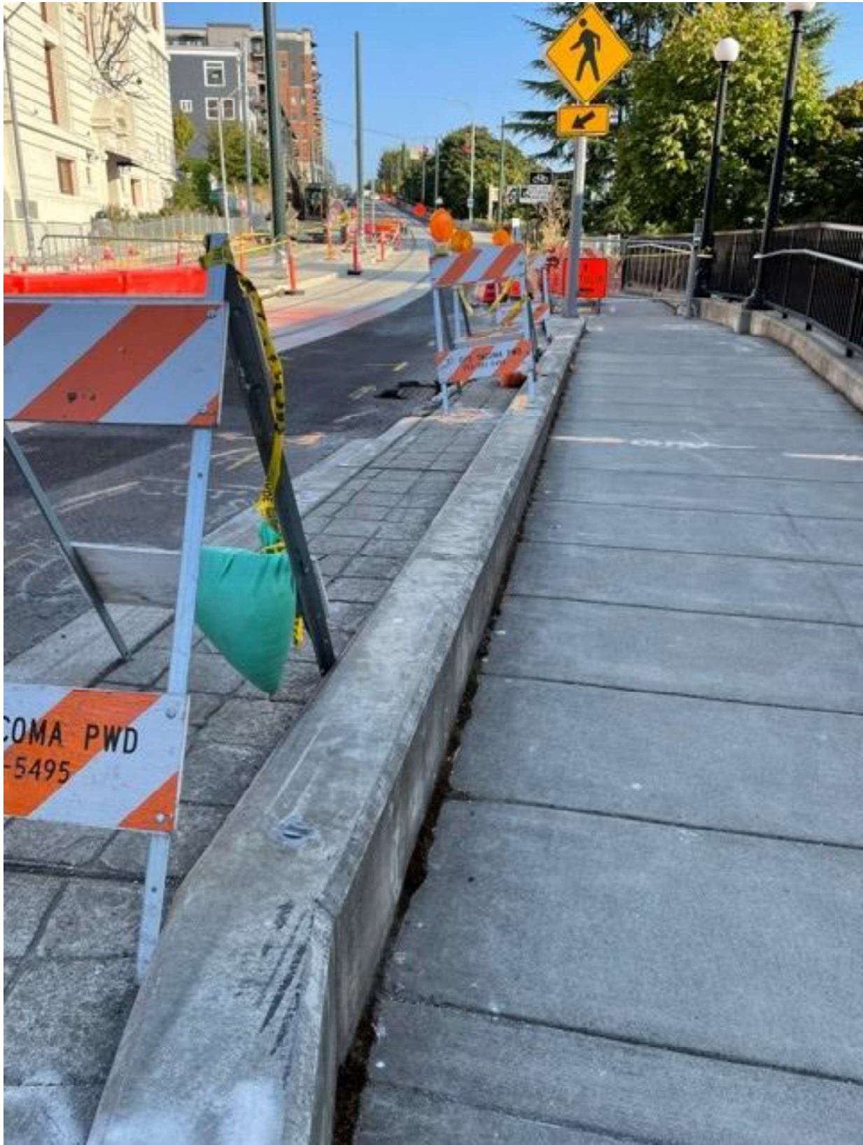
Curb on which new railing will be installed (via surface mount).
