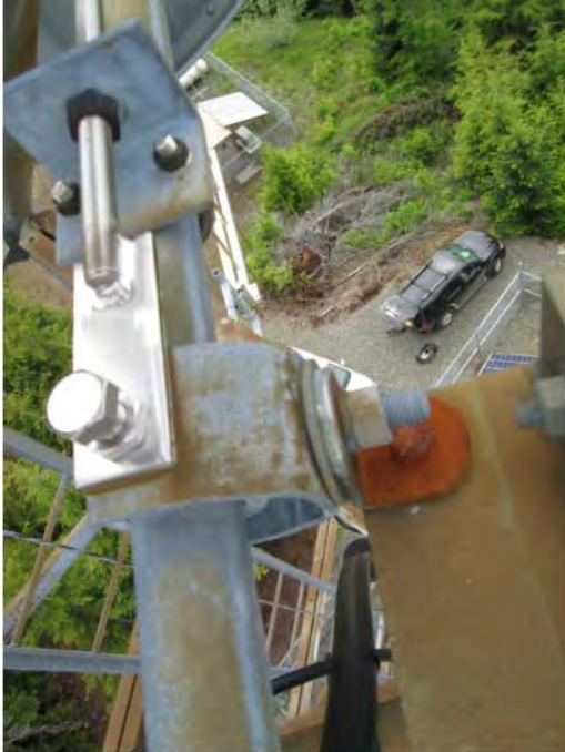
141 Weatherwax Hardware Corrosion
