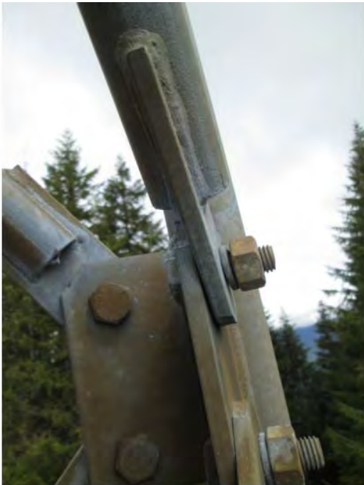
097 Weatherwax Loose Diagonal Bolt 46' N Leg
