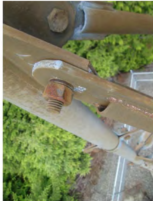
094 Weatherwax Corrosion
