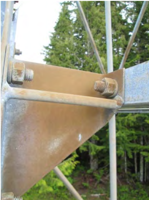
077 Weatherwax Corrosion
