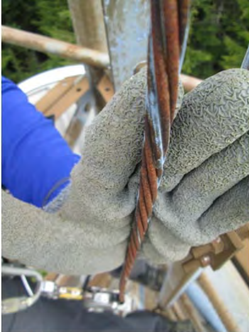
137 Weatherwax Corrosion Safety Climb
