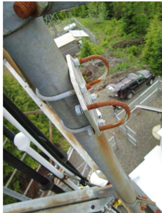
100 Weatherwax Abandoned Mount Hardware
