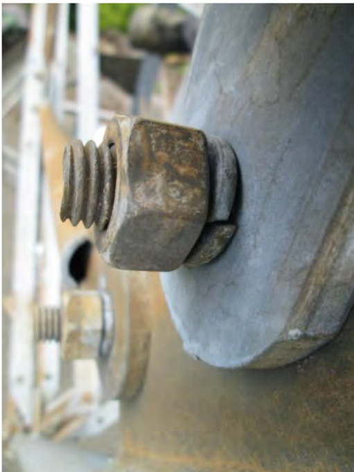
099 Weatherwax Loose Diagonal Bolt 46' N Leg
