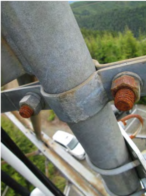
101 Weatherwax Hardware Corrosion
