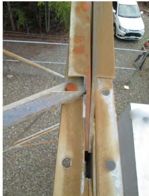
072 Weatherwax Corrosion
