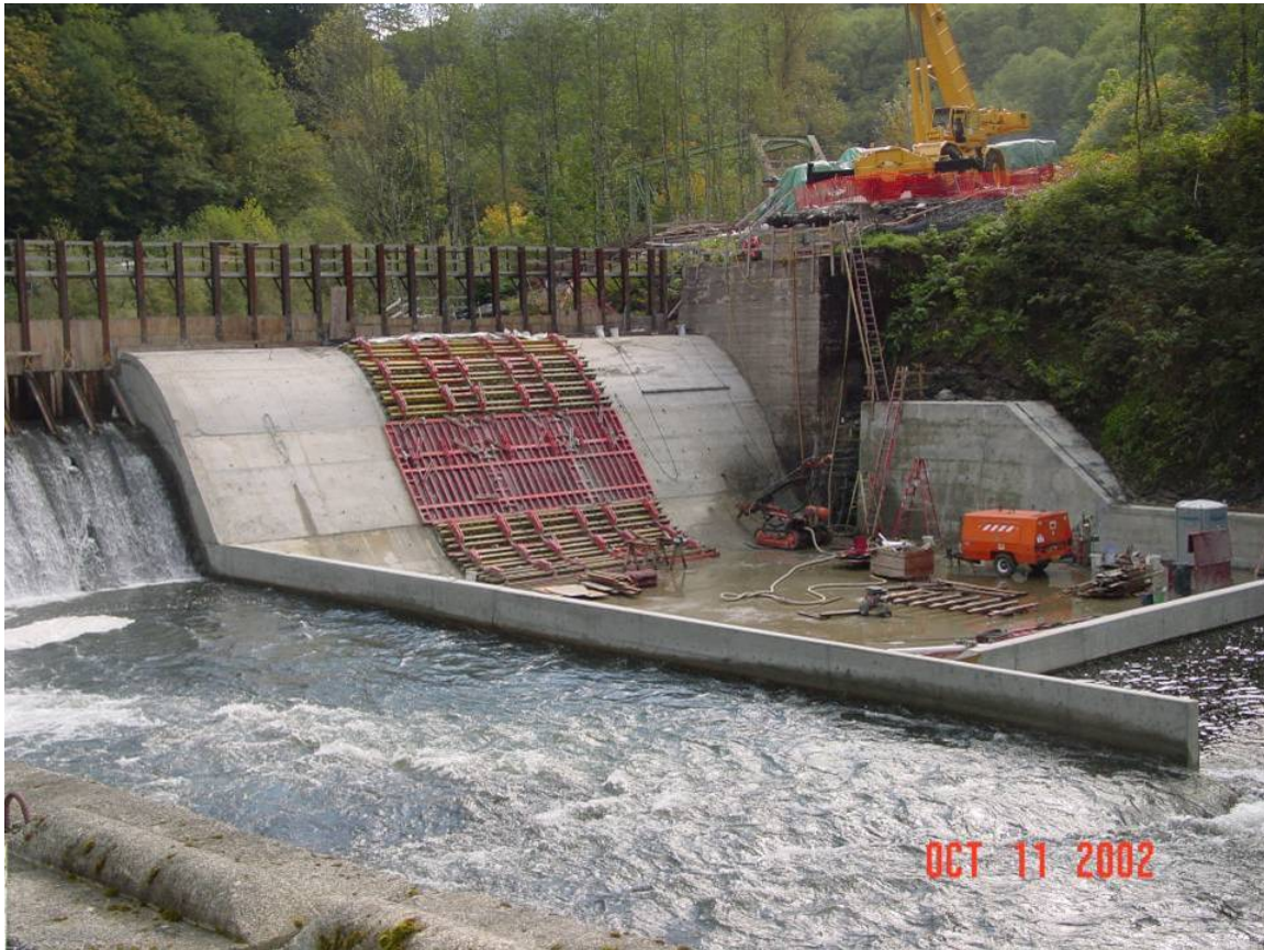
Figure 2. Headworks Dam during construction of the dam raising project showing the increased dam height, sinusoidal spillway, and pool retention sill.
