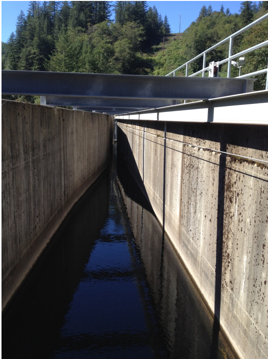
Photo 21 Flow In Front of the Screens and Baffles (Fish Screen Basin), Final Configuration (Q = 210 cfs)
