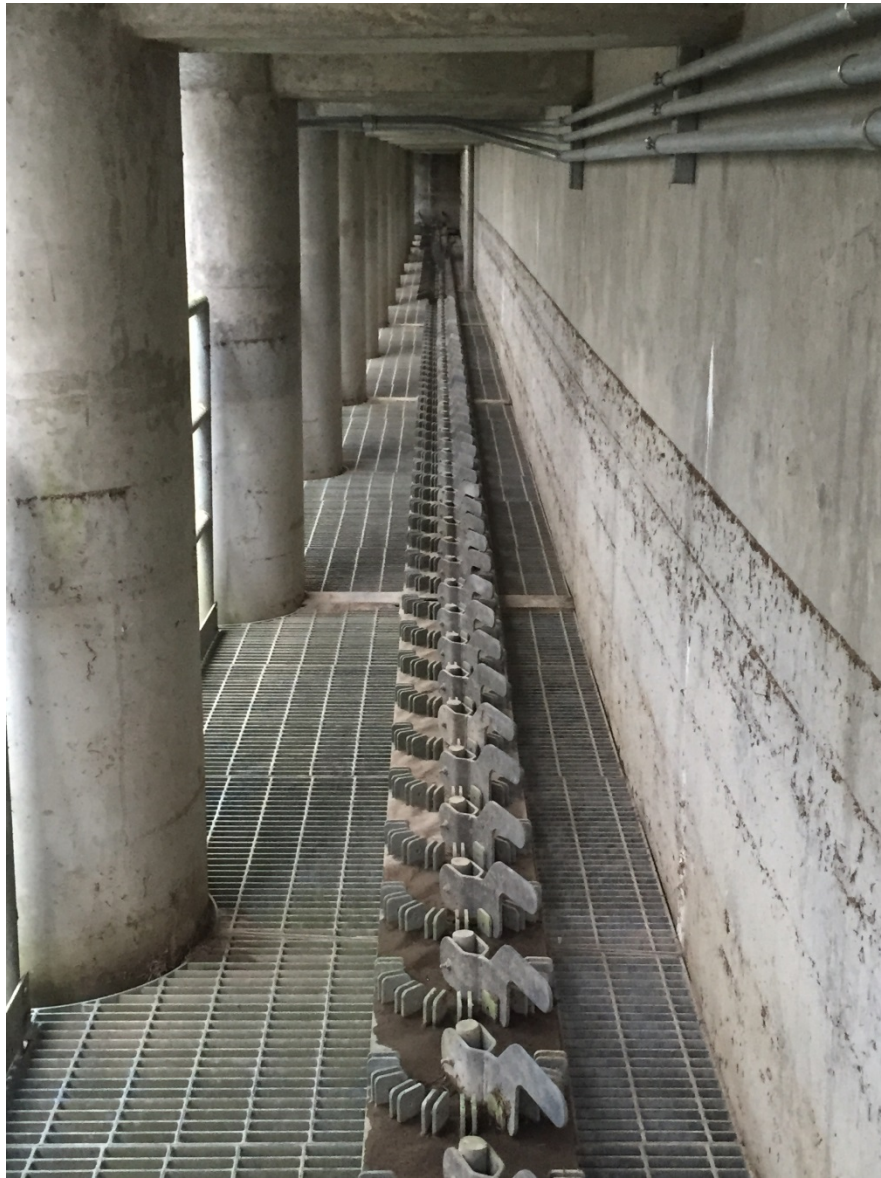
Photo 16 Final Baffle Configuration (Looking Upstream)
