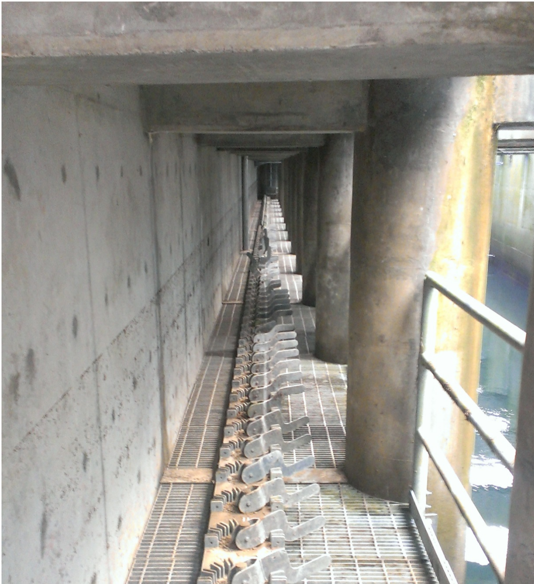
Photo 17 Final Baffle Configuration (Looking Downstream)
