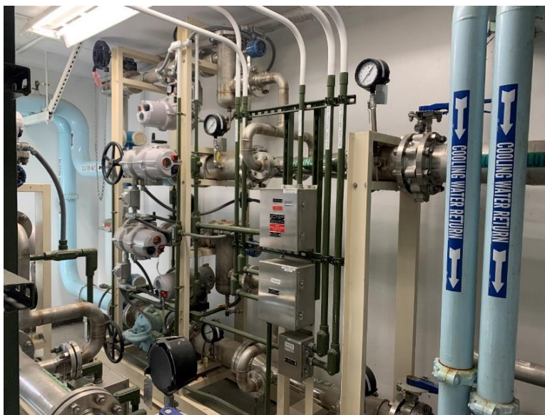
Figure 3.6. Existing Reactor 5 Sidestream Injection System
