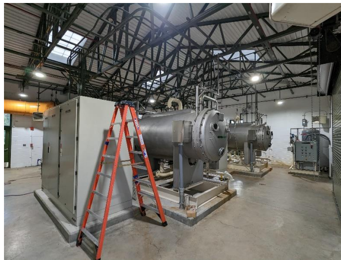
Figure 3.2. Ozone Generator and PSU
