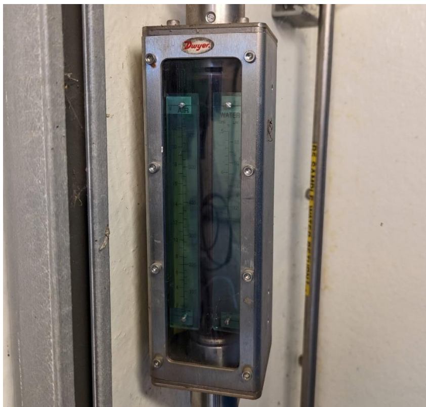
Figure 3.10. Existing Rotameter in Ozone Sample Station (Reactor 5, Sample Station 2)
