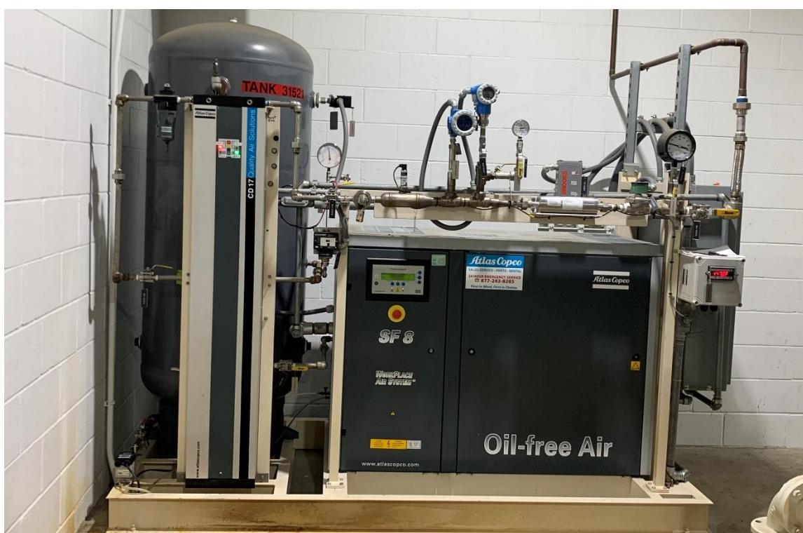
Figure 3.4. Existing Nitrogen Boost Skid
