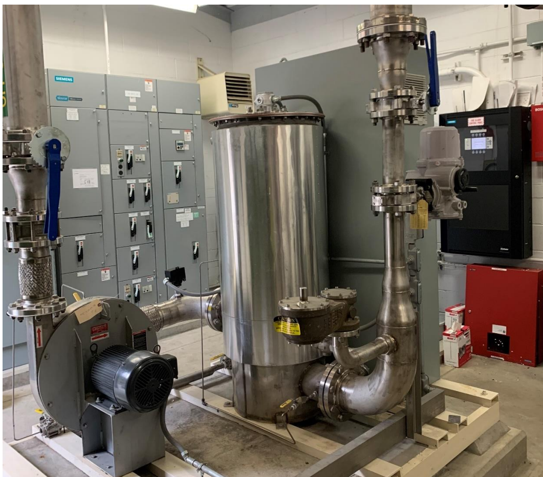
Figure 3.9. Existing Ozone Destruct Unit
