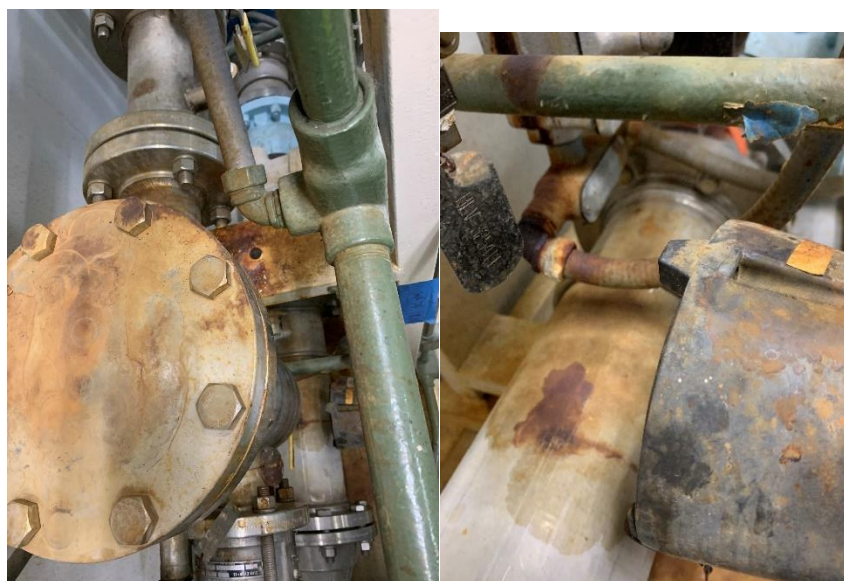
Figure 3.7. Corrosion on Reactor 5 Ozone Injection Piping
