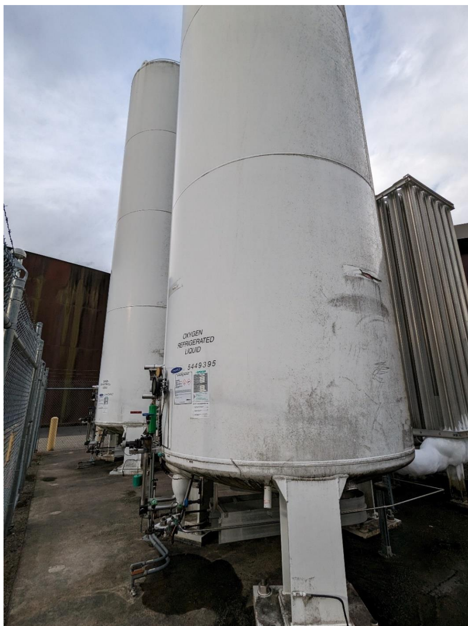
Figure 3.3. Existing LOX Tank and Vaporizers
