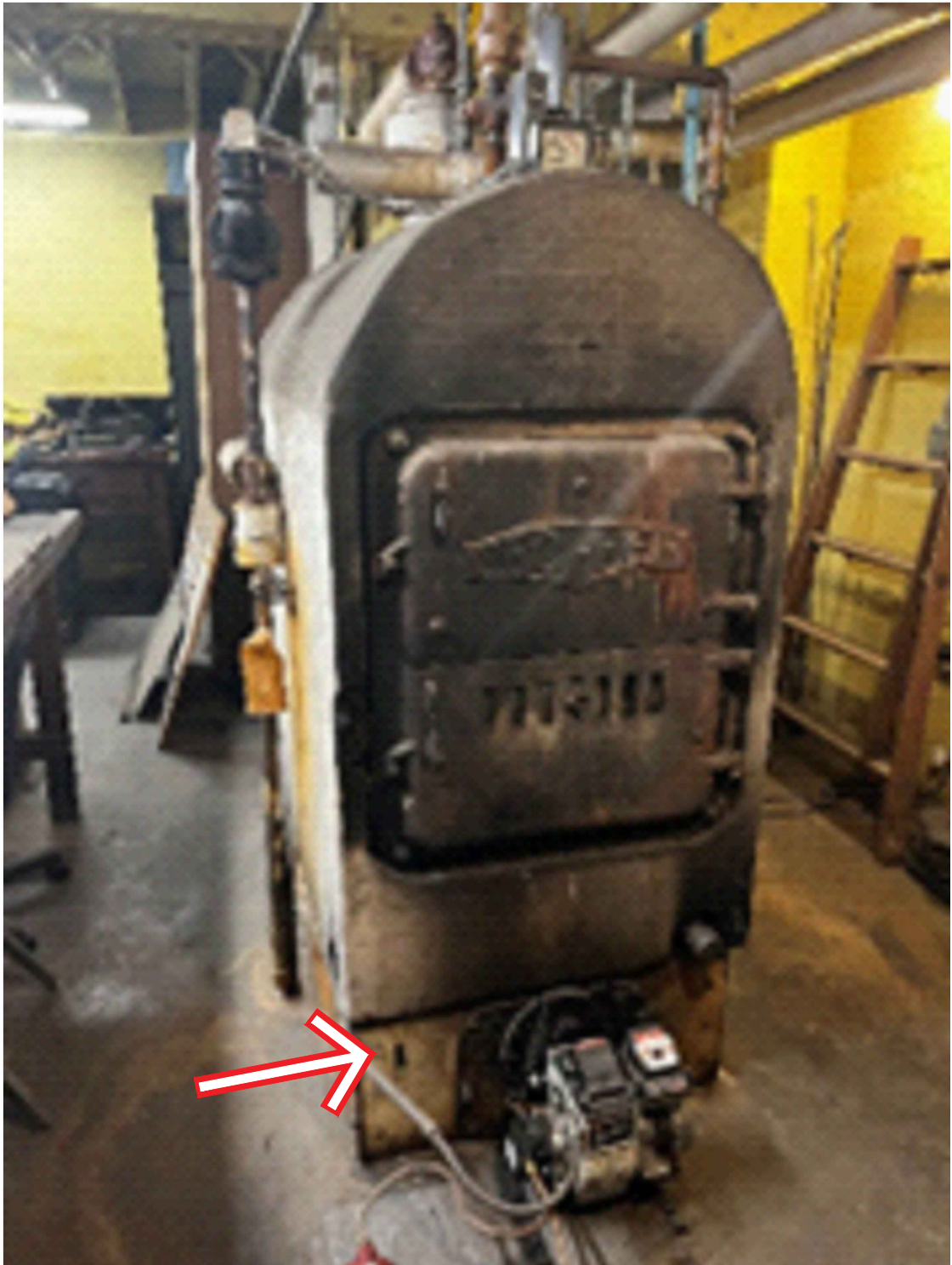
PHOTO 1 LOCATION OF ASBESTOS-CONTAINING POWDERY PATCH ON BASE OF BOILER.
