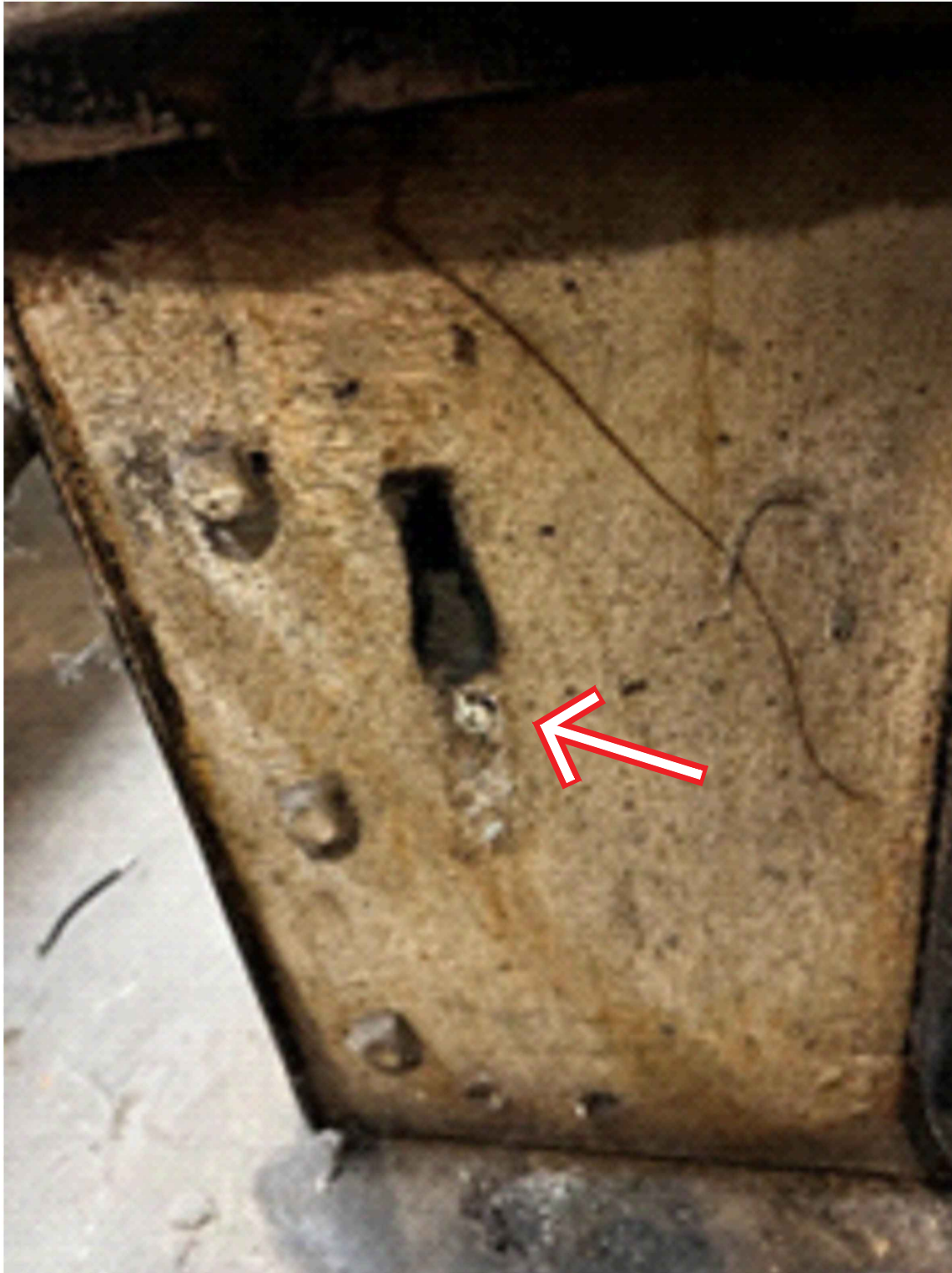
PHOTO 2 LOCATION OF ASBESTOS-CONTAINING POWDERY PATCH ON BASE OF BOILER.
