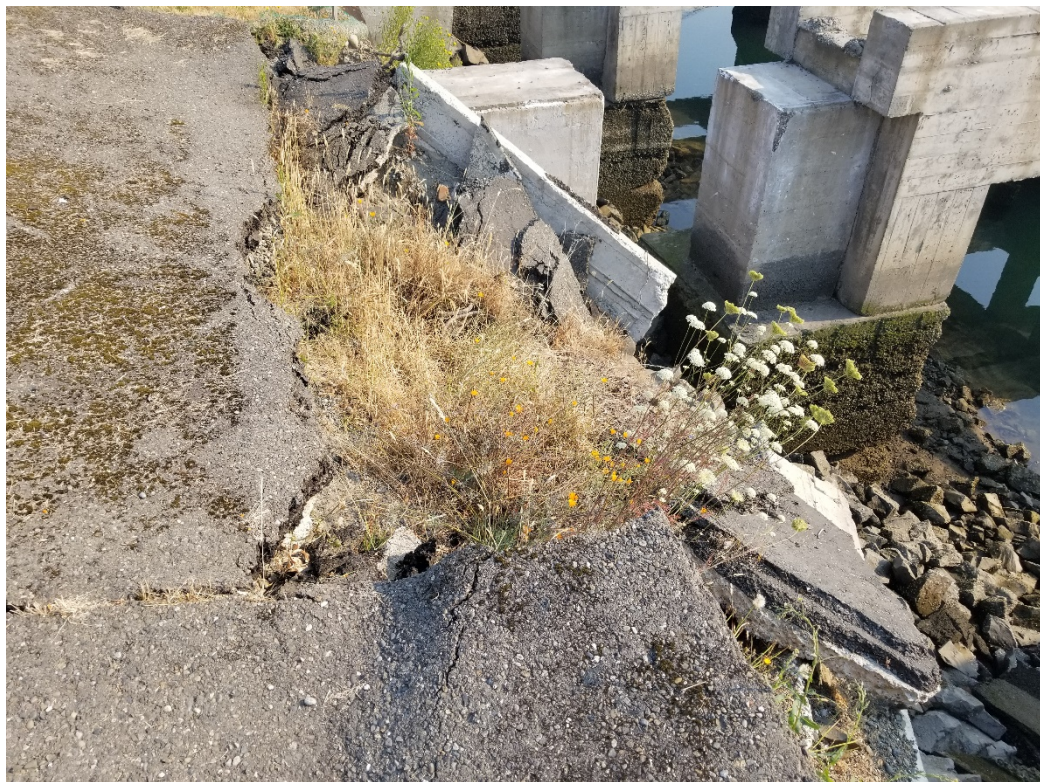
Photograph 6 – Concrete and asphalt debris to be removed, where above mean high water (MHW) and asphalt to be replaced with native grass at Municipal Dock.
