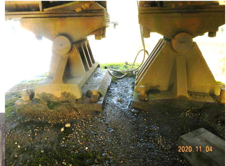
Debris accumulation on Girder Top/Bottom Gussets and Bearings
