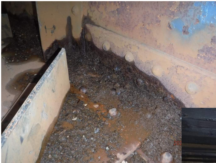
Debris accumulation on Girder Top/Bottom Gussets and Bearings
