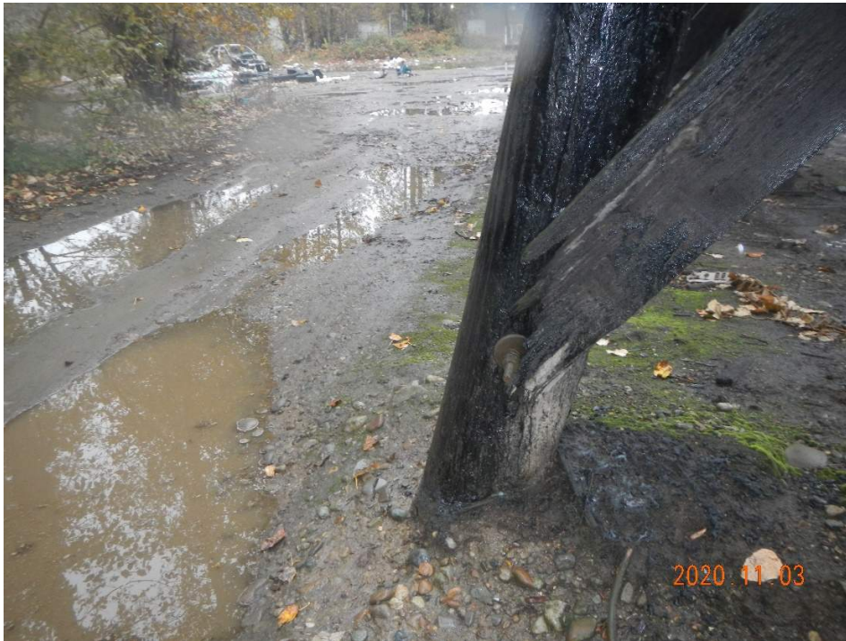
Broken sway brace at Bent 14 right side connection to base of Pile 5.
