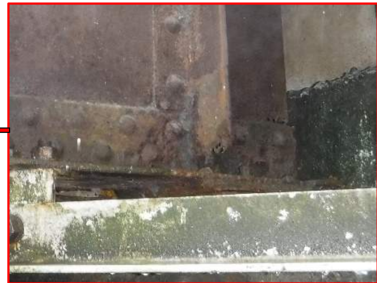
Replace Bearing Stiffener – Span 33, Stringer 4 @ Abutment 34
