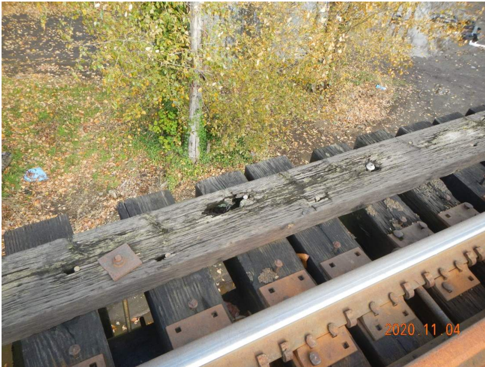
Typical Tie Spacer and Condition
