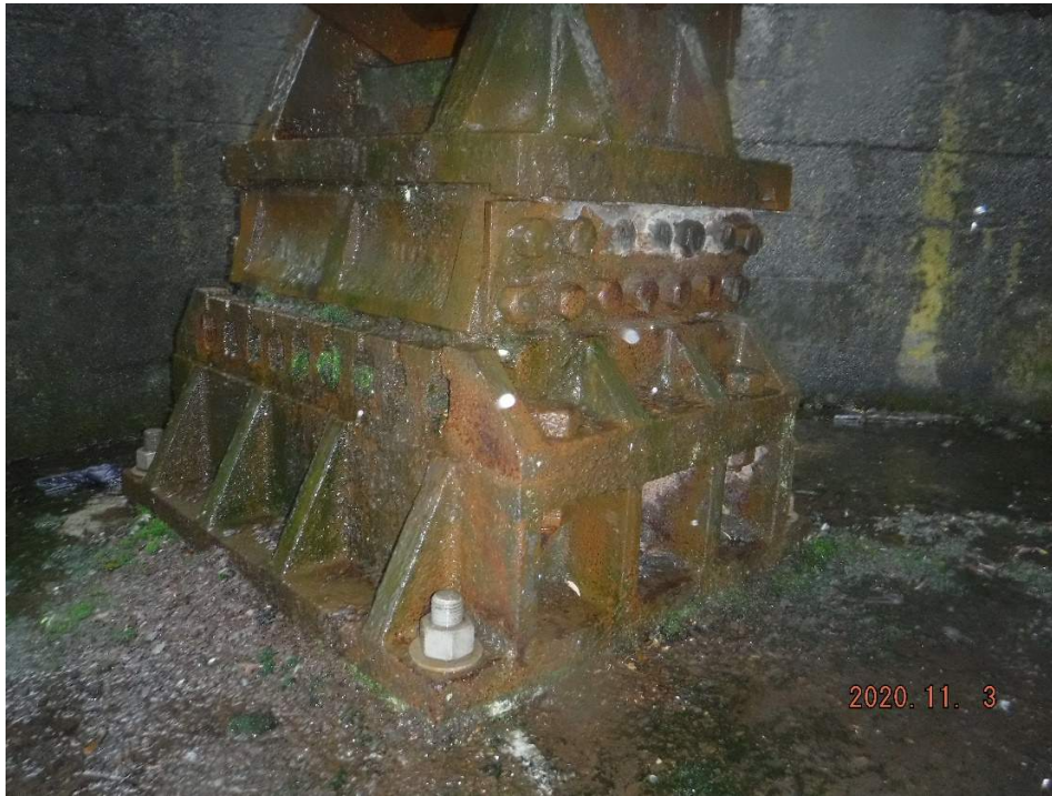
Clean and re-grease bearings for both Span 22 and 33
