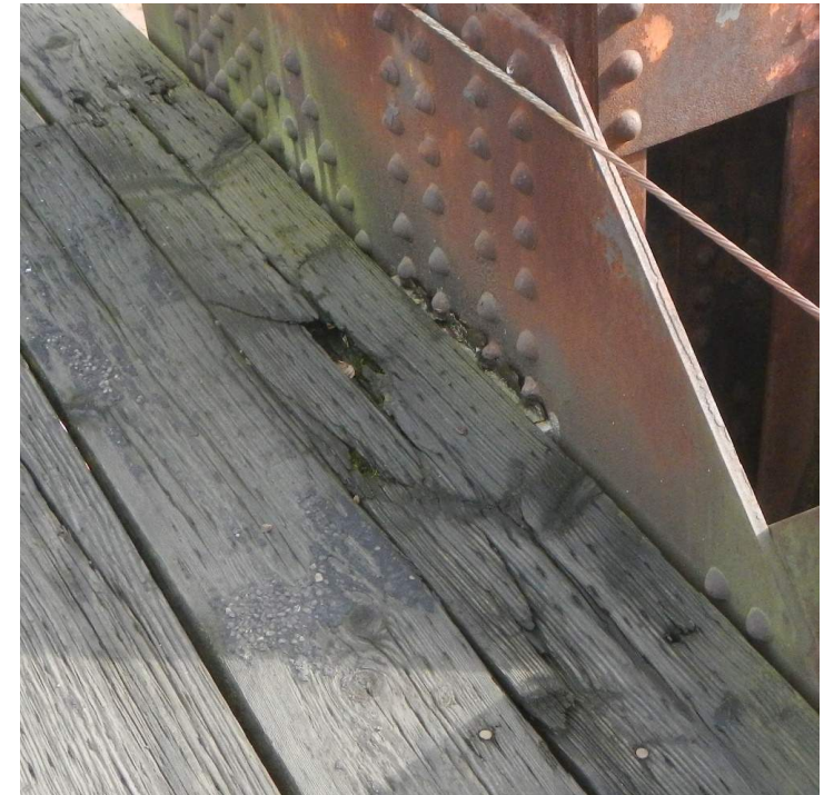
Typical decayed and failed walkway planks
