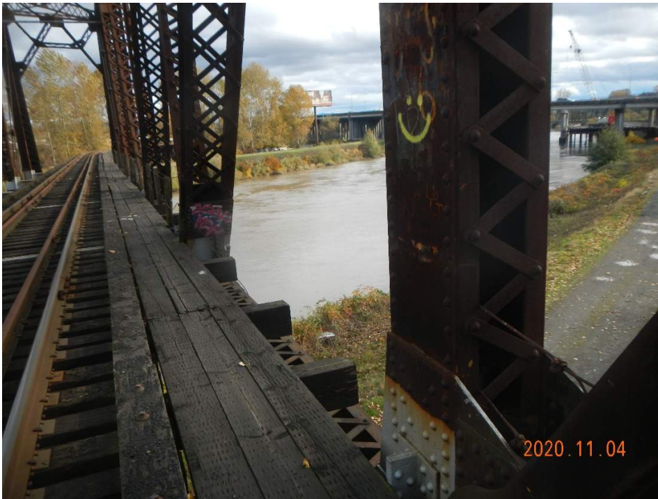
Walkway on Steel Truss Span
