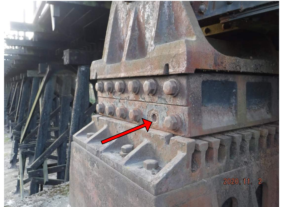
Replace missing bearing roller bolts (span 22 shown)
