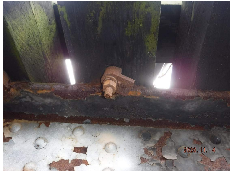
Typical loose tie bridge clip
