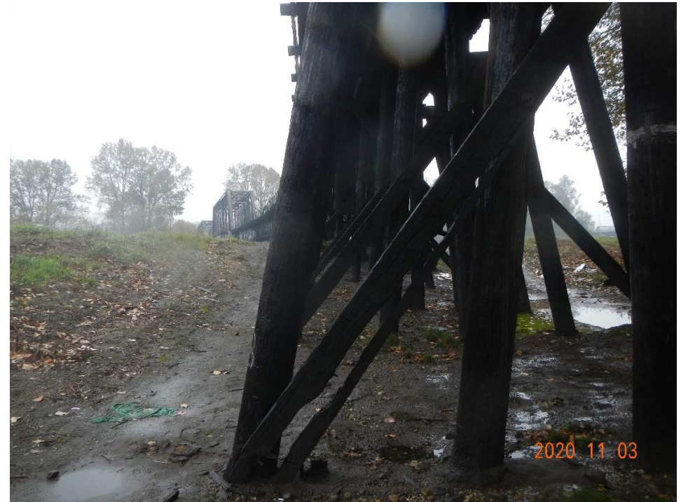
Broken sway brace at Bent 13 left side connection to base of Pile 1.
