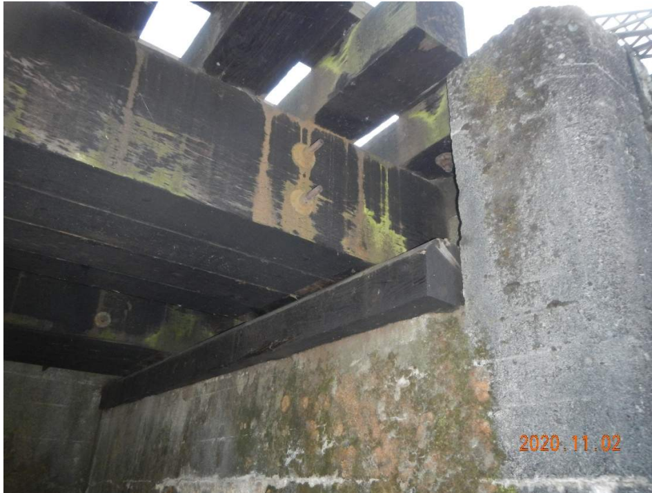
Typical Timber Stringer Configuration
