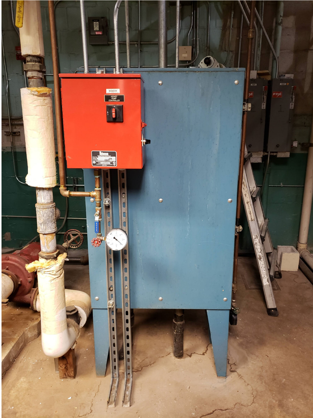
View of existing fire pump & jockey pump controllers
