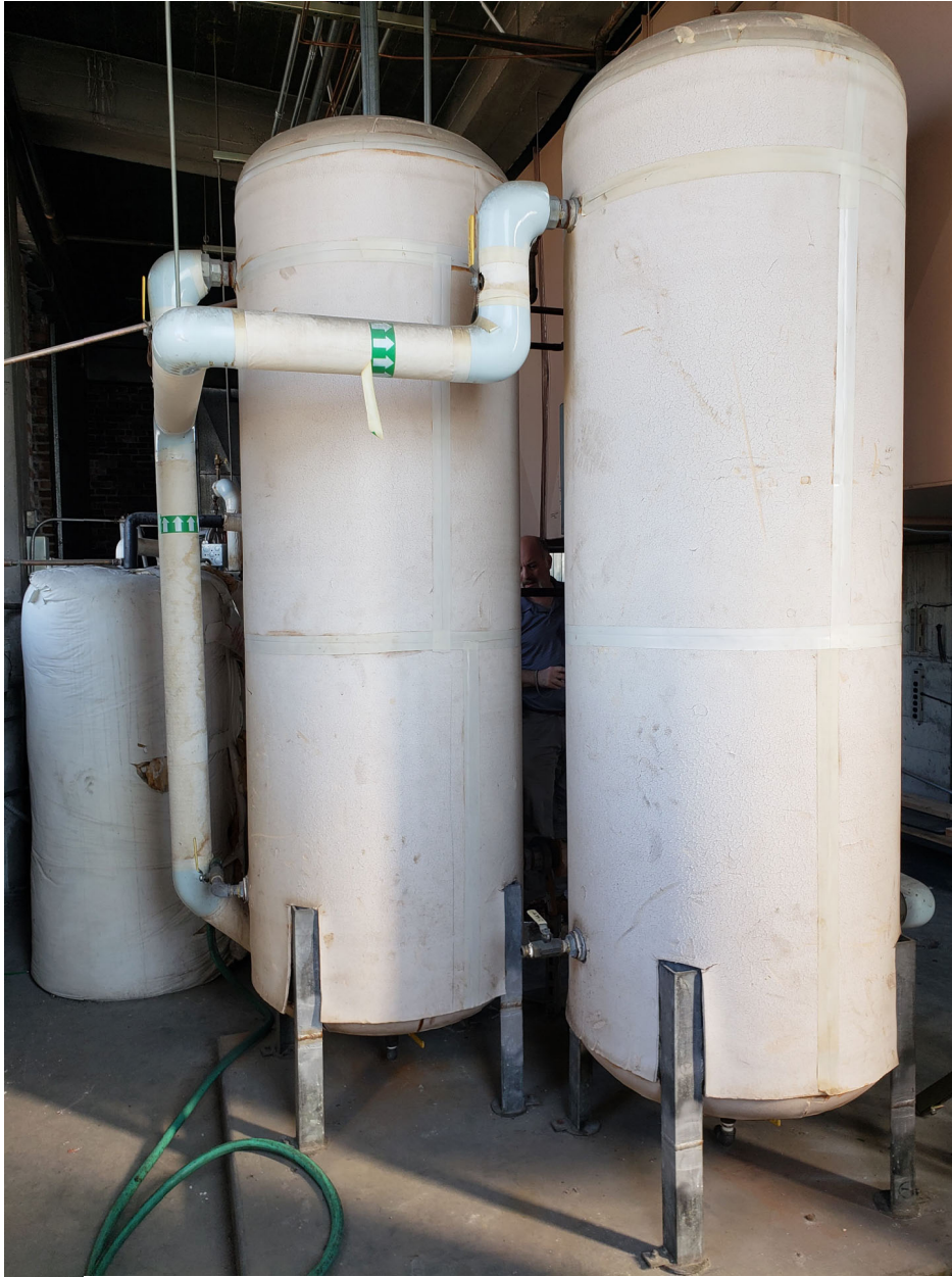
View of existing domestic water pressure tanks and water heater
