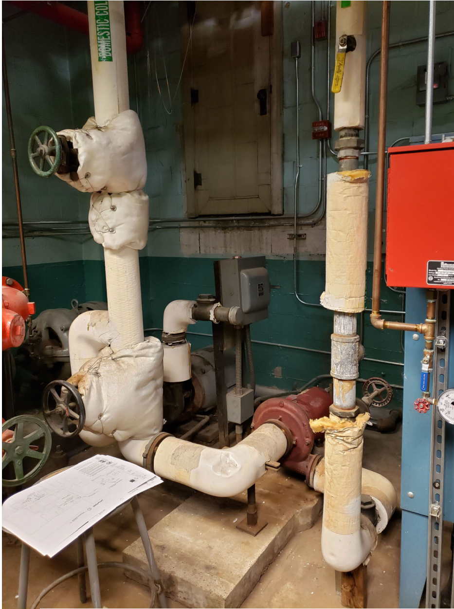
View of existing domestic water pumps
