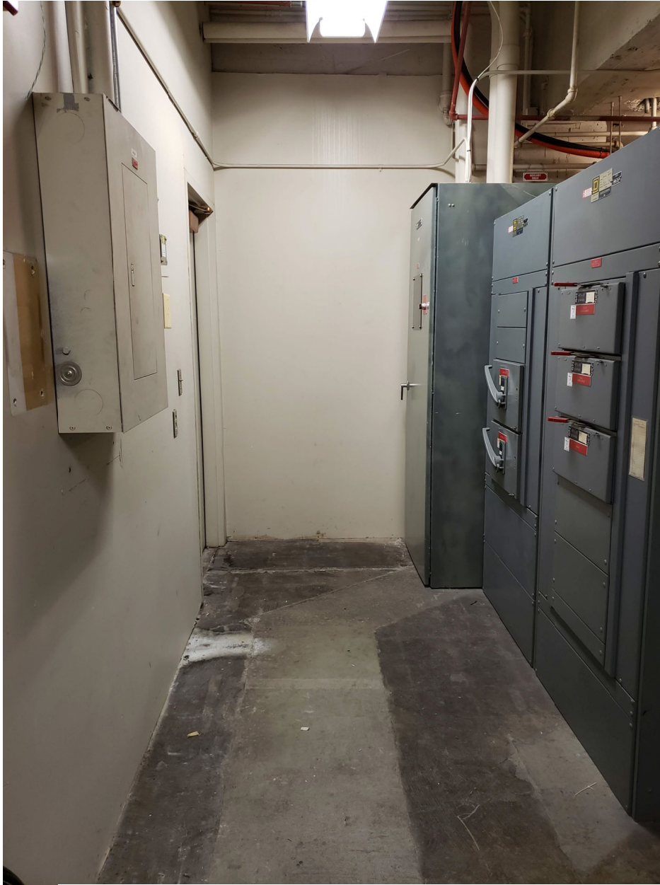
View of existing Automatic Transfer Switch Cabinet (far end right) and EM panel (left)
