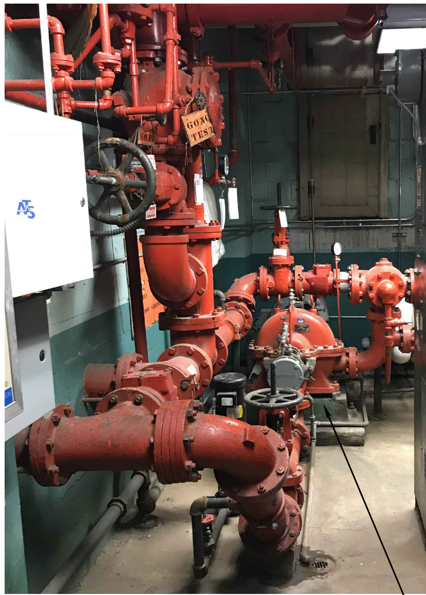
DEMO EXISTING FIRE PUMP, JOCKEY PUMP, AND ASSOCIATED PIPING AND COMPONENTS AS REQUIRED FOR NEW FIRE PUMP INSTALLATION (SEE DETAIL #4 AT LEFT)
