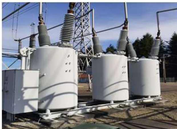
230KV Oil Circuit Breaker
