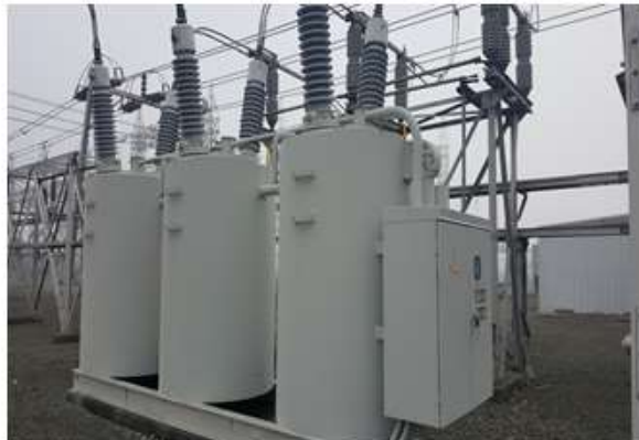
230KV Oil Circuit Breaker
