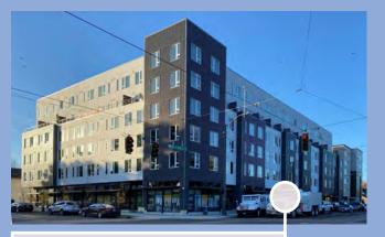
Massing breaks reduce perceived scale, provide rhythm along street-facing facade, and create opportunities for upper level outdoor spaces with additional solar access.
