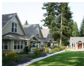
Cottage Housing in all except HMR-SRD
