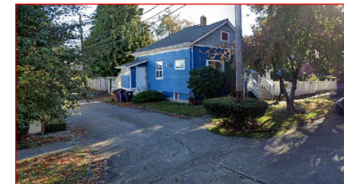
(F) VIEW OF EXISTING BUILDING ACROSS THE ALLEY WAY FROM GARAGE
