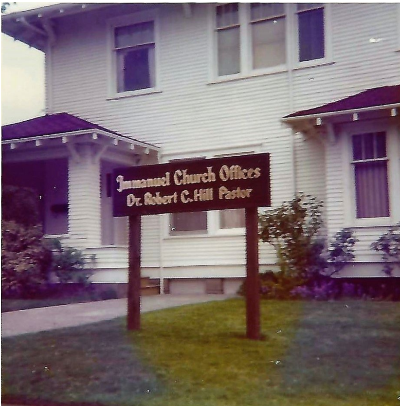
Fig. 12 –The manse, showing original cladding, ~1976 (Immanuel Coll.)
