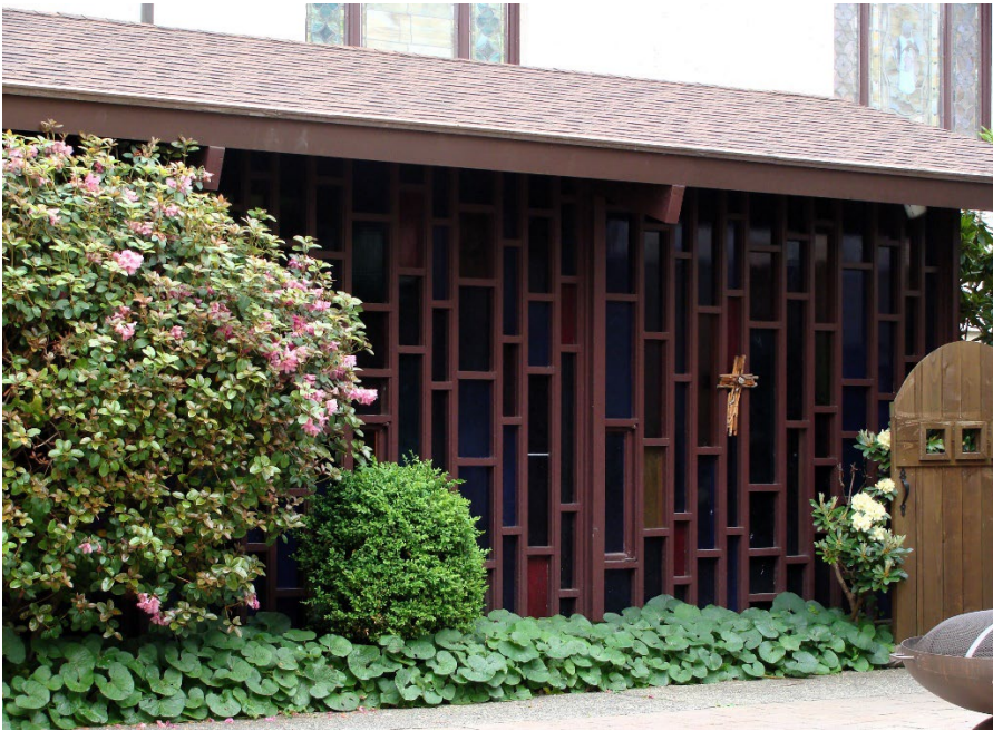
Fig. 31 – Detail of chapel showing west façade window wall, 2023 (Immanuel Coll.)
