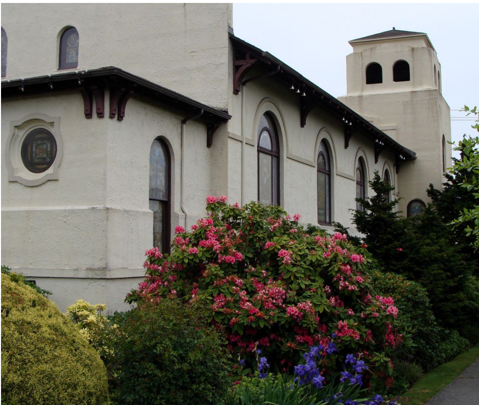
Fig. 19 – East façade of the sanctuary and belfry, 2023 (Immanuel Coll.)
