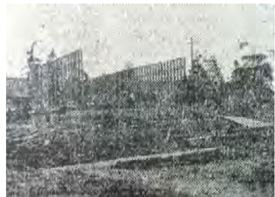
1910May22 TDT, Under Construction
