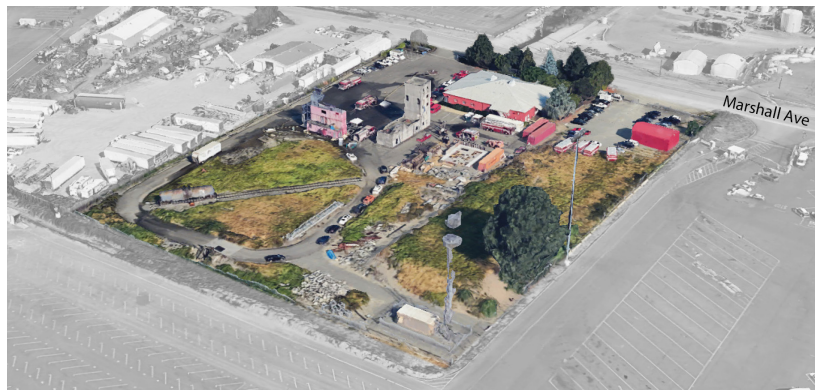
Figure 116. Fire Training Center
