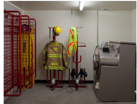
Figure 23. Decontamination room at a Hood River, OR fire station, with dedicated laundry and storage for turnout gear
