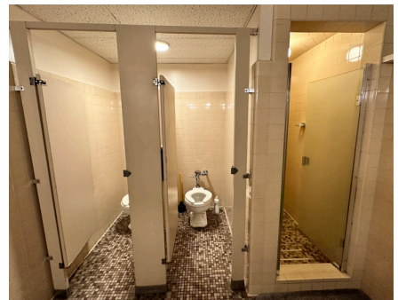
Figure 44. Station 6 has insufficient restroom facilities
