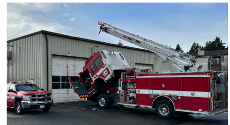
Figure 4. Fire Garage is undersized for modern apparatus
