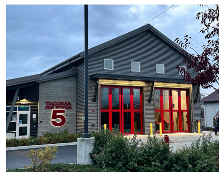
Figure 12. Completed in 2021, Station 5 is TFD’s newest facility
