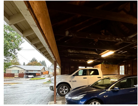
Figure 95. Staff park in a carport off the alley behind Station 14
