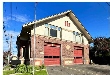
Figure 143. Renovating Station 13 preserves an historic community asset
