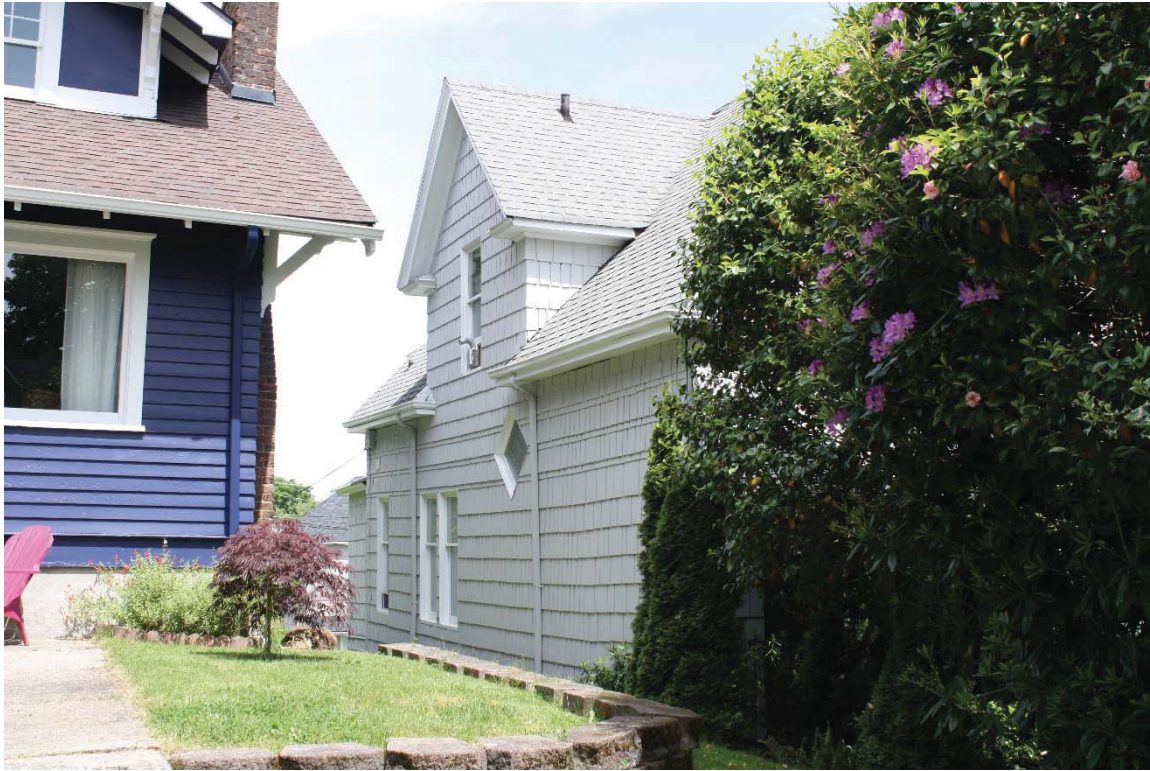
Figure 18. West elevation of 205 N. Yakima Avenue, view to northeast
