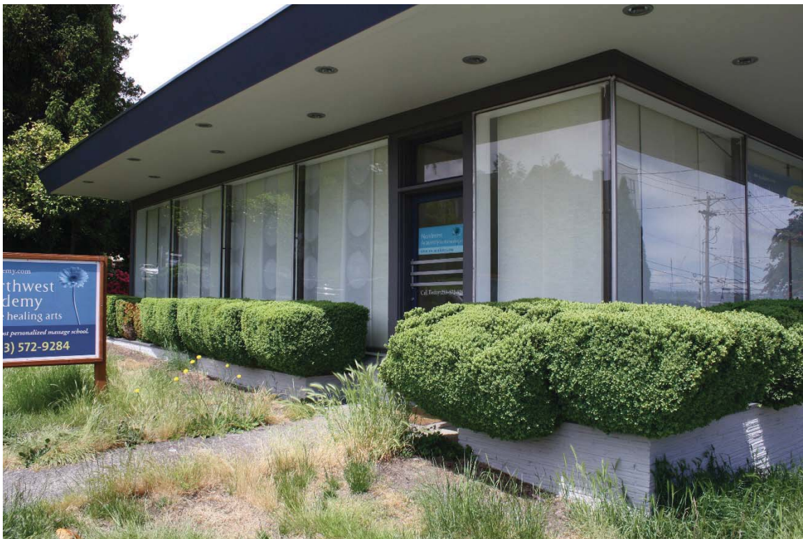
Figure 13. Detail of primary (south) elevation, 201 N. Yakima Avenue, view northwest
