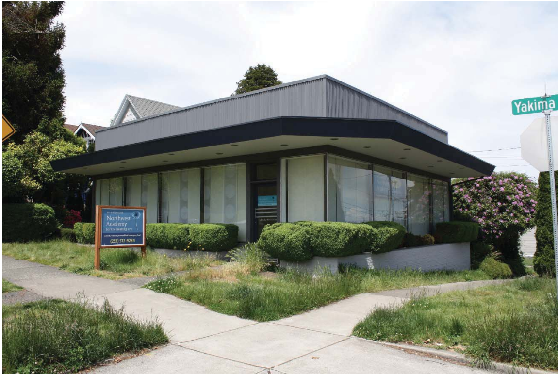
Figure 12. Overview of 201 N. Yakima Avenue, view northwest
