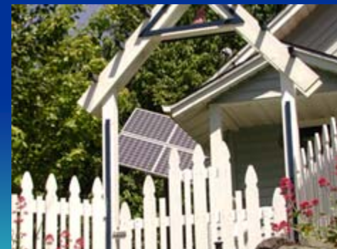
Solar power in Tacoma
