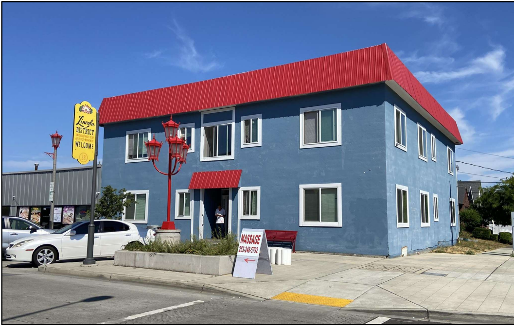
Figure 6. The Vernon Apartments at 3830 Yakima Avenue South has had significant design alterations, including the red, metal-clad mansard-style parapet and front entrance hood.
