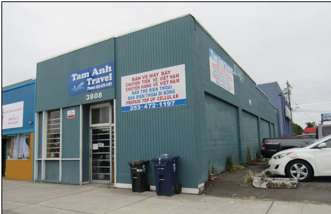
Figure 3. The former Lincoln Bank (3808 South Yakima Avenue), has lost its longtime neighbor, the Model Bakery, which once occupied the space where this surface parking lot is now located (seen on the right). This change has diminished the integrity of setting.
