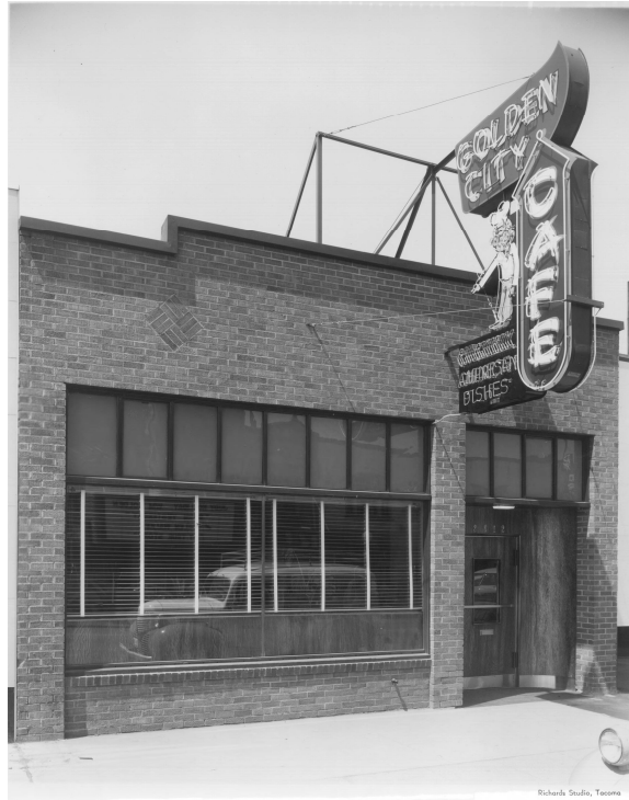
Figure A-15: The Golden City Cafe opened in the former post office building at 3812 Yakima Avenue in 1951.
