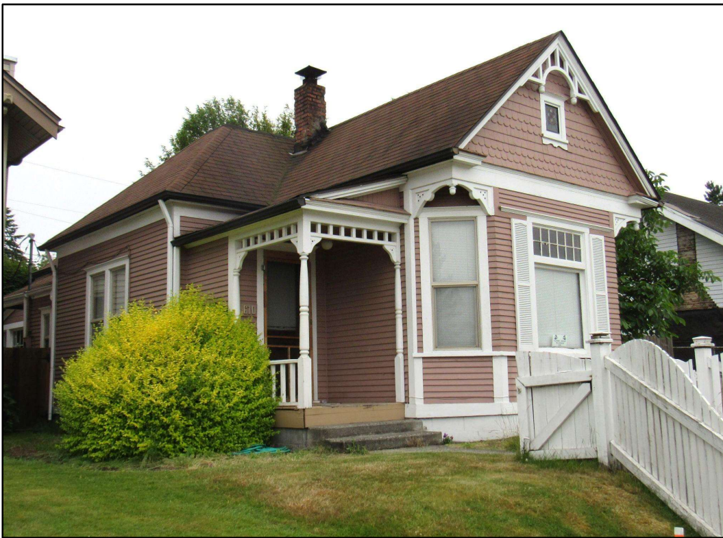
Figure 11. The front (north) and side (west) elevations of Queen Anne style 610 South 38 th Street. Note its raised position above the sidewalk.
