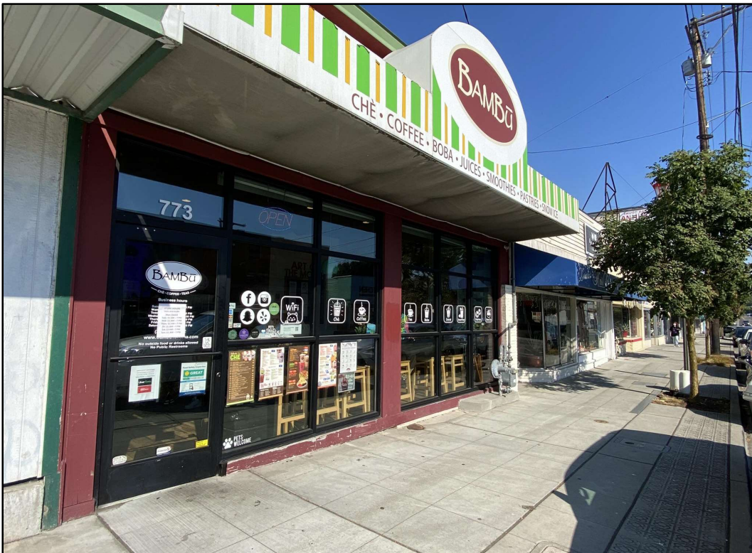
Figure 7. 769 South 38 th Street, now known as Bambo restaurant, has recently had its storefront completely replaced with a modern, metal-framed system. This modification has changed its design.
