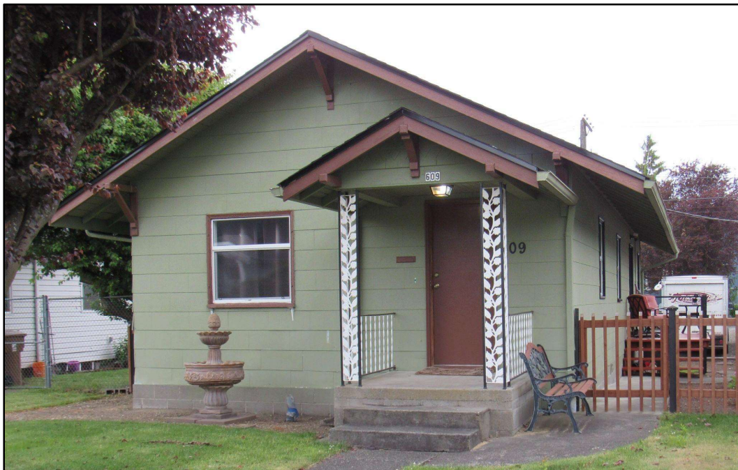
Figure 5. 609 South 34 th Street has a porch structure with a design and materials more in keeping with a 1950s house than a Craftsman bungalow.
