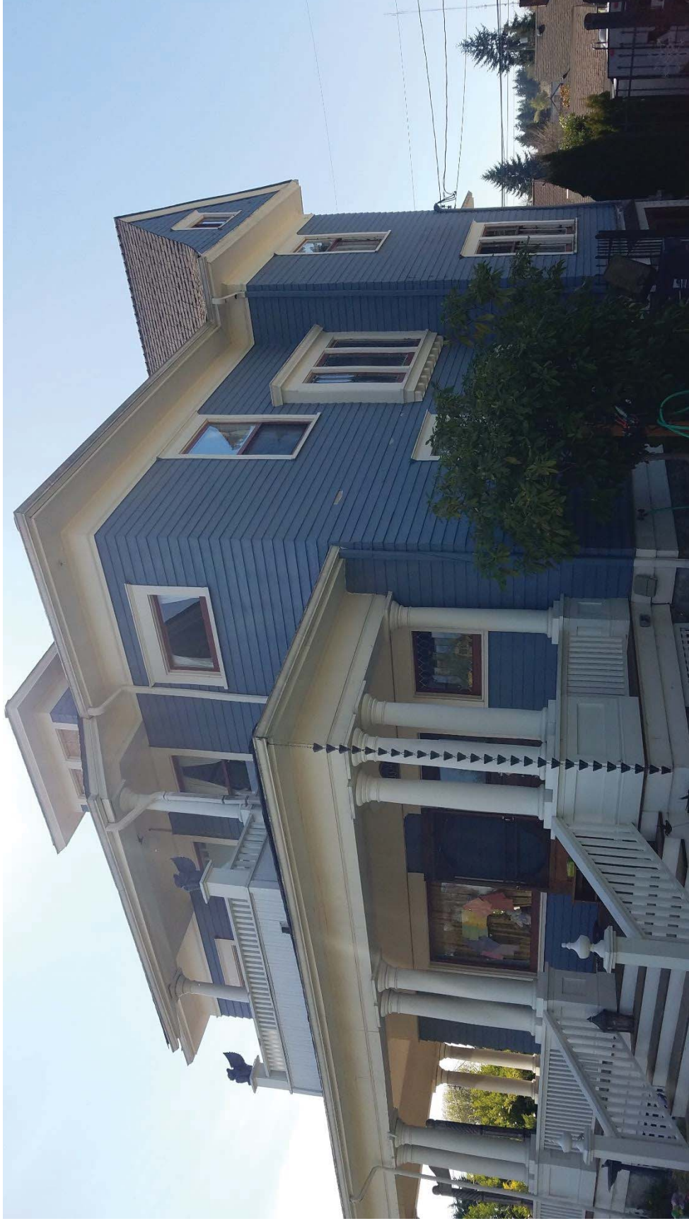
Northeast Corner of House - 2020
