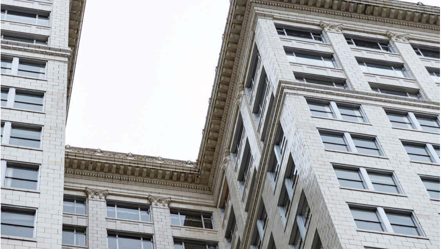
IMAGE 15. After: south facade cornice and upper stories detail.
