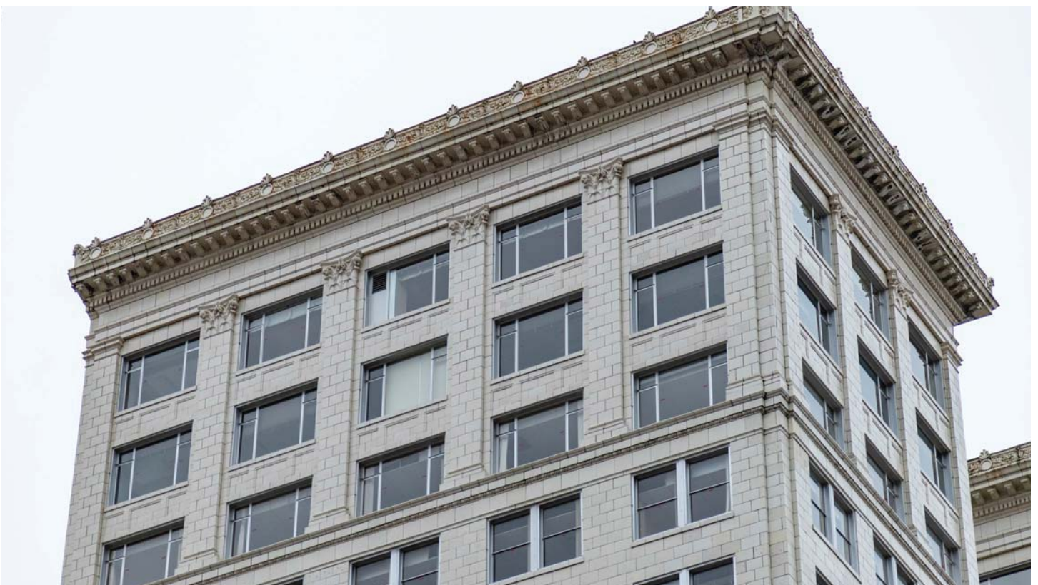
IMAGE 18. After: west facade cornice and upper story detail.
