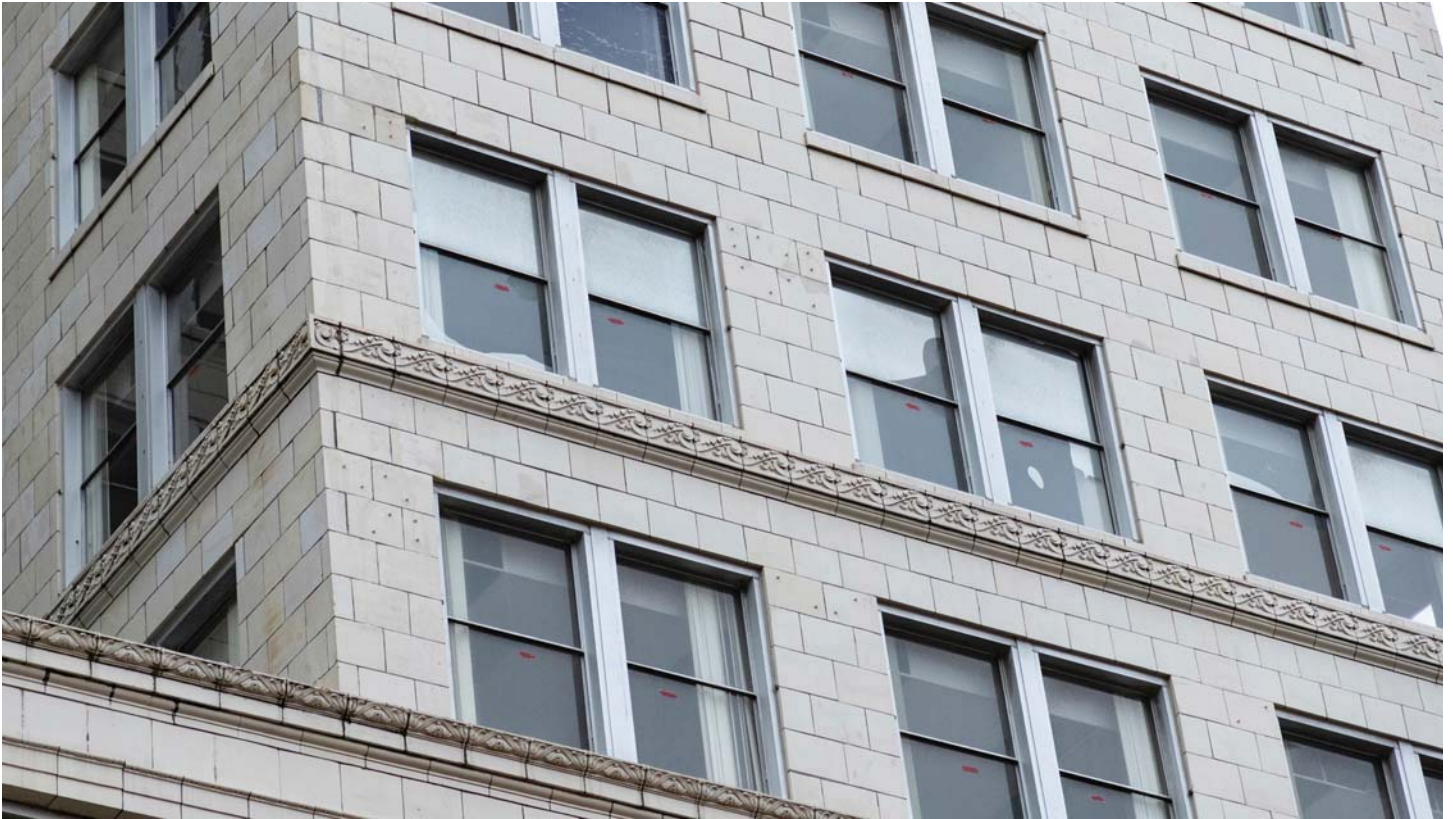
IMAGE 17. After: south facade upper story detail.
