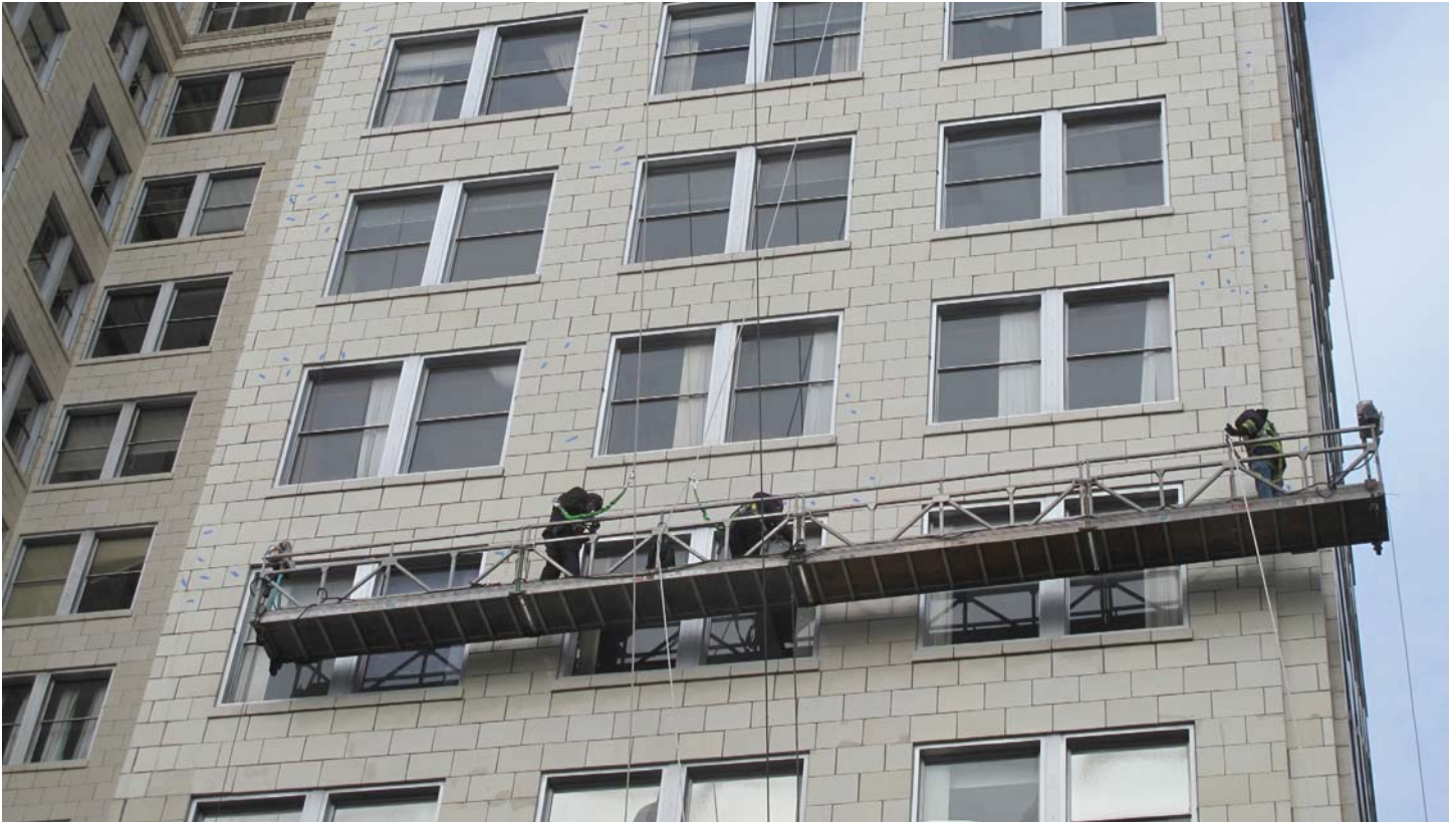
IMAGE 11. During: repair areas identification. January 22, 2018 view.
