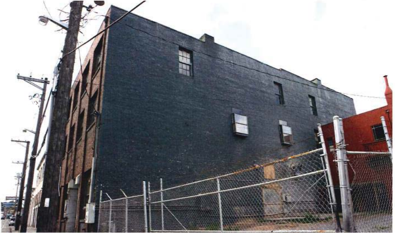
North facade in August 2014, pre-work.
