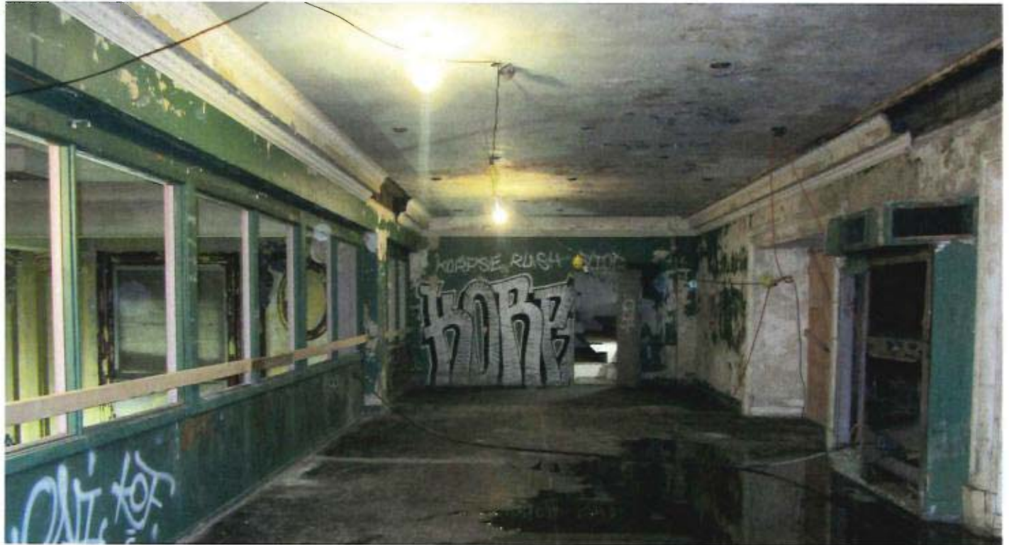
Mezzanine between ballroom and Broadway level, looking north. 2016.
