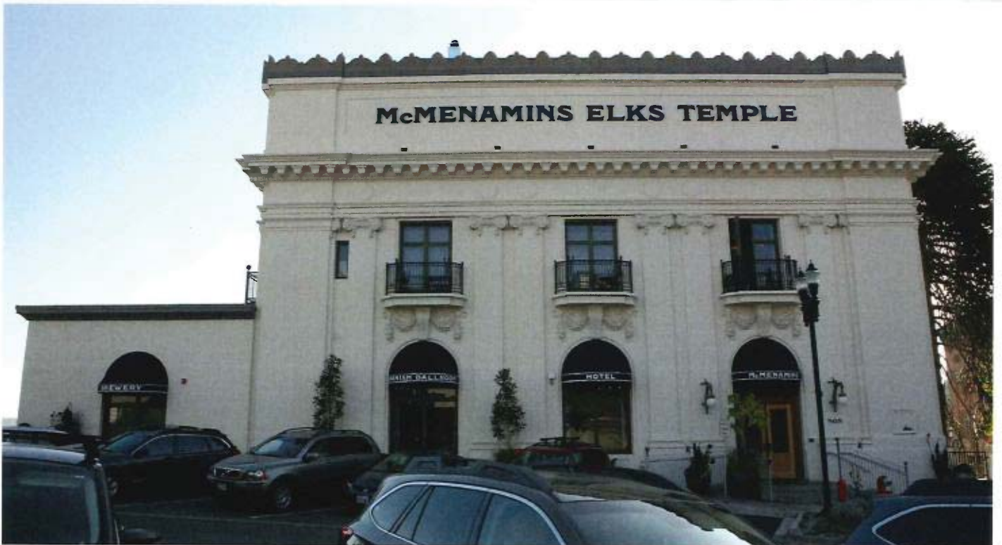
West facade in 2019, showing completed work.
