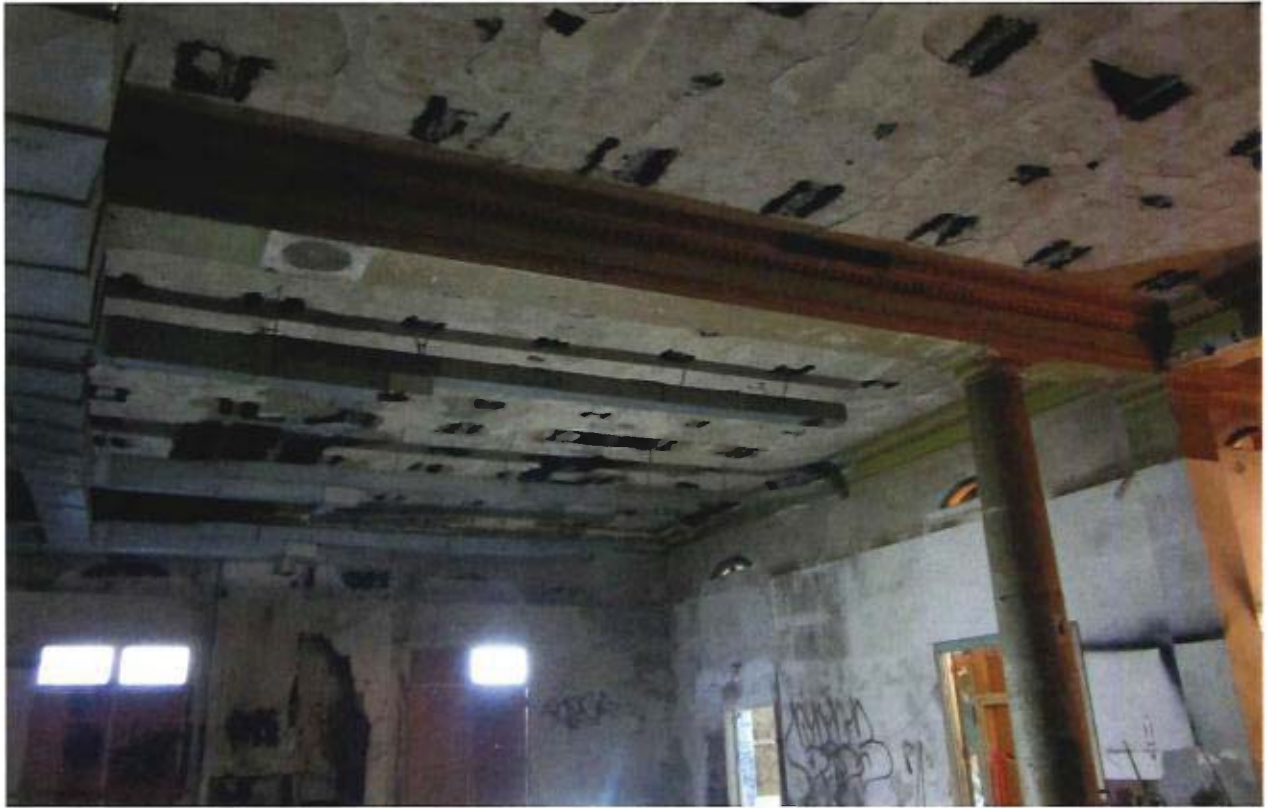
Main clubroom at Broadway level looking east/southeast, pre-work. (2016)
