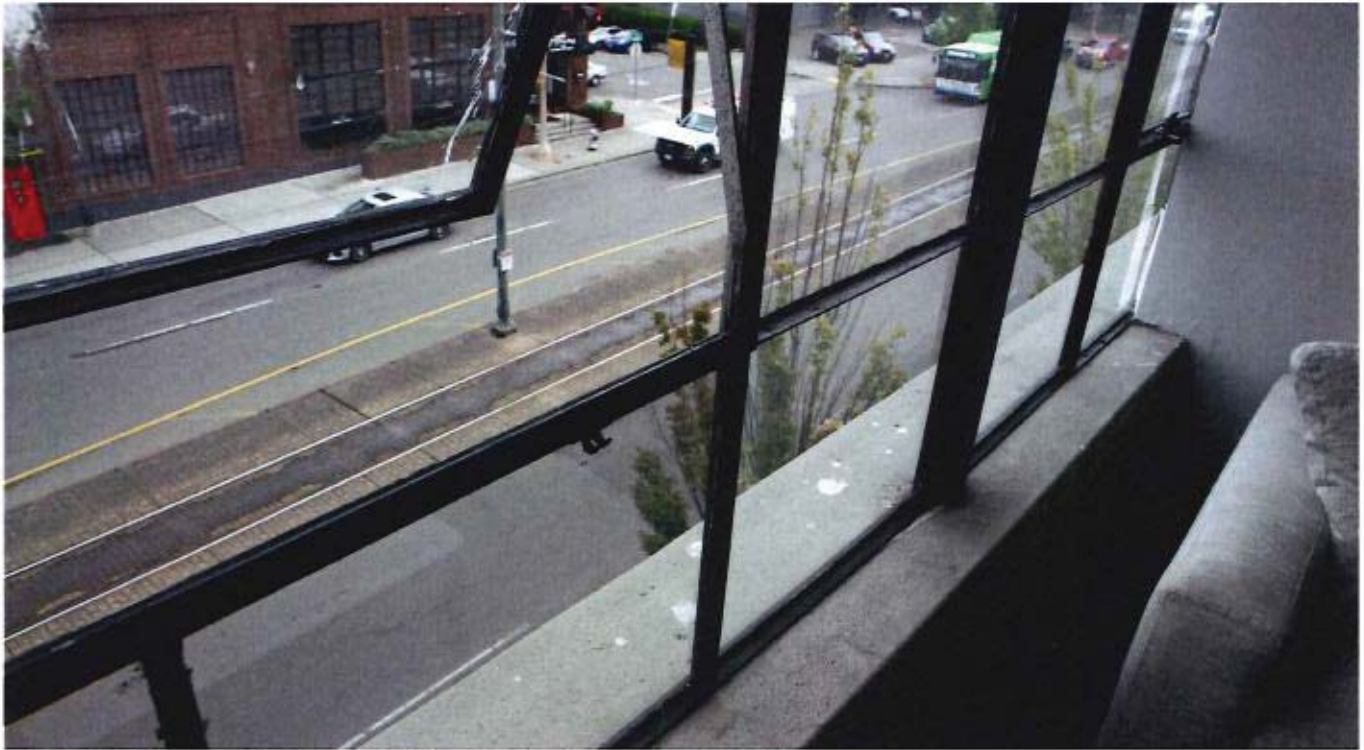
Typical metal sash window detail, looking east. September 2019.
