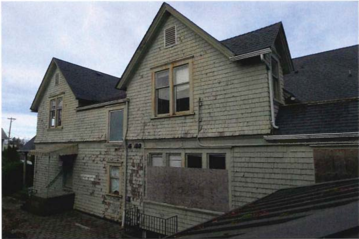
South facade, March 2017.
