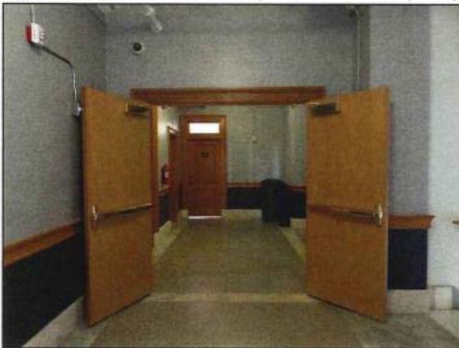
Figure 52. Fire doors added to fourth floor corridor (2019).
