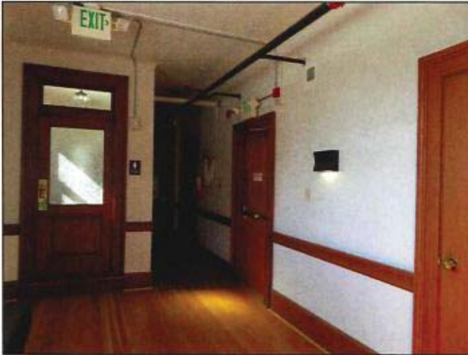
Figure 56. Fifth-floor corridor with door to stair and restroom (2019).
