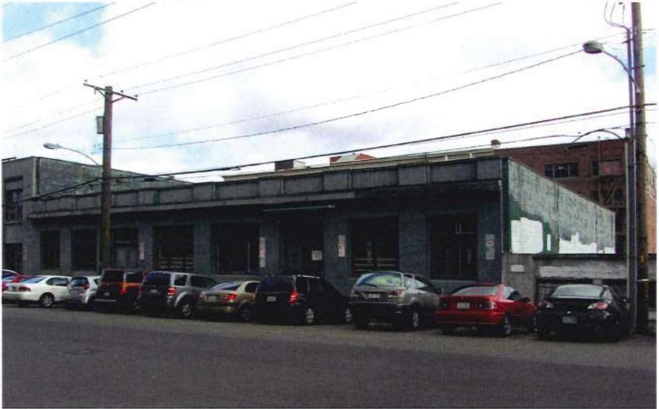
Southwest corner in 2013, pre-work.
