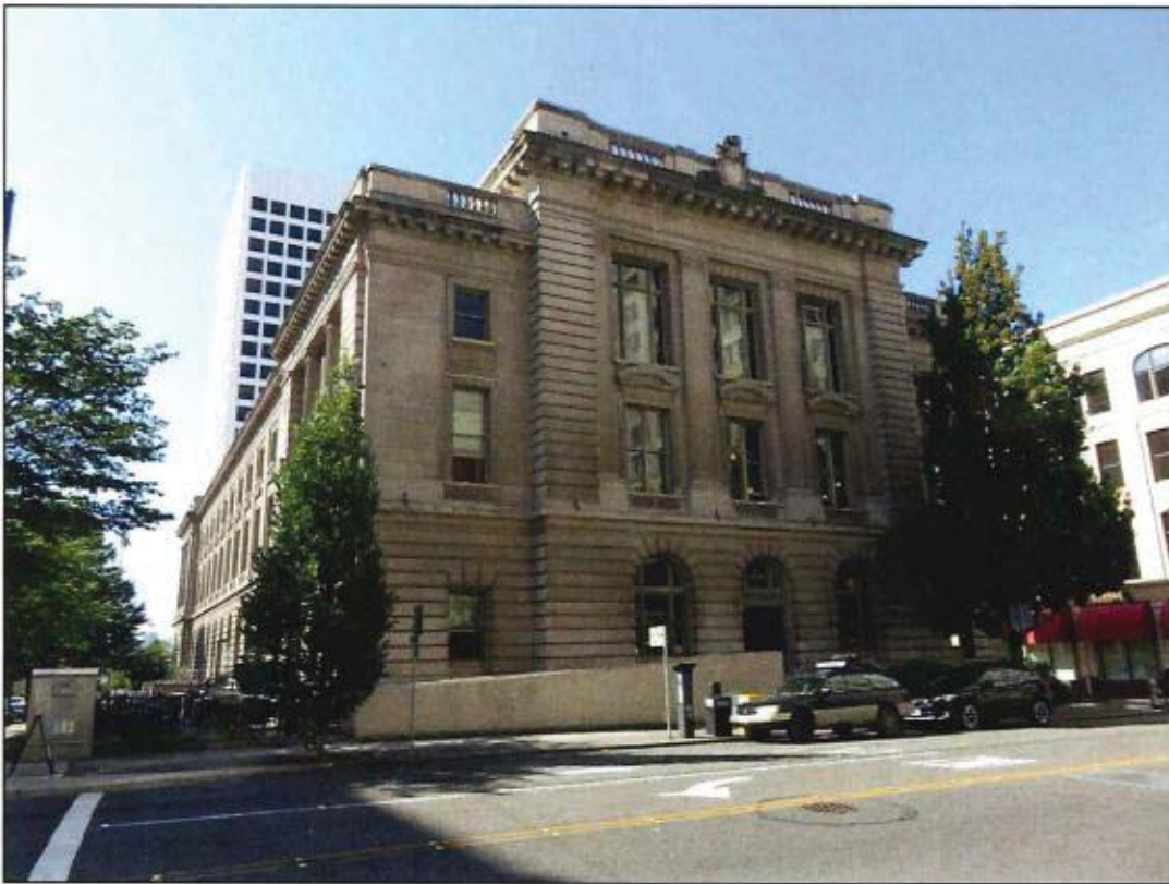
Figure 3. 1102 A Street, north elevation (C. Beckner, 2019).
