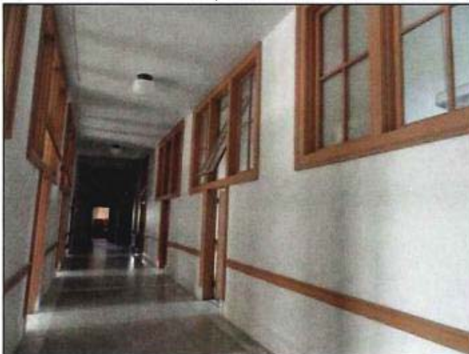
Figure 31. Double-loaded corridor, third floor (2012).
