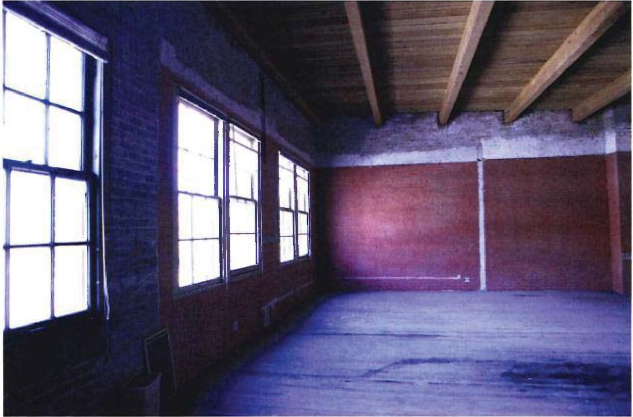
3rd floor, looking north along west wall. 2016.
