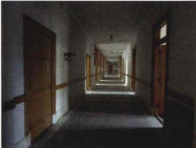
Figure 42. Fourth-floor corridor before rehabilitation (2012).
