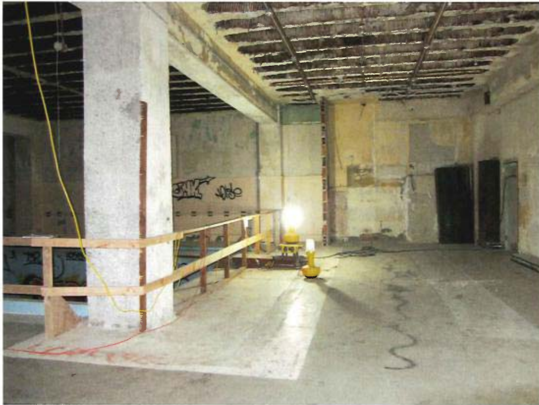
Main basement space (former pool room) looking north. 2016.
