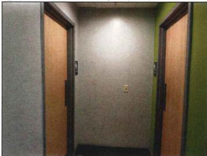
Figure 16. Basement level men's and women's restrooms (2019).
