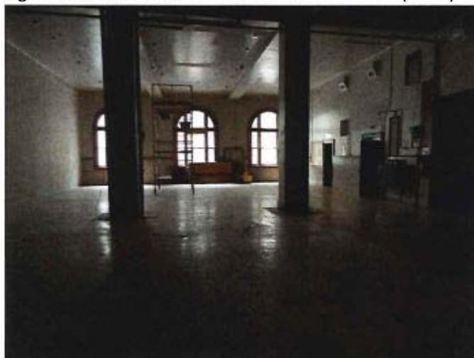
Figure 19. Example of unused main floor storage space (2012).
