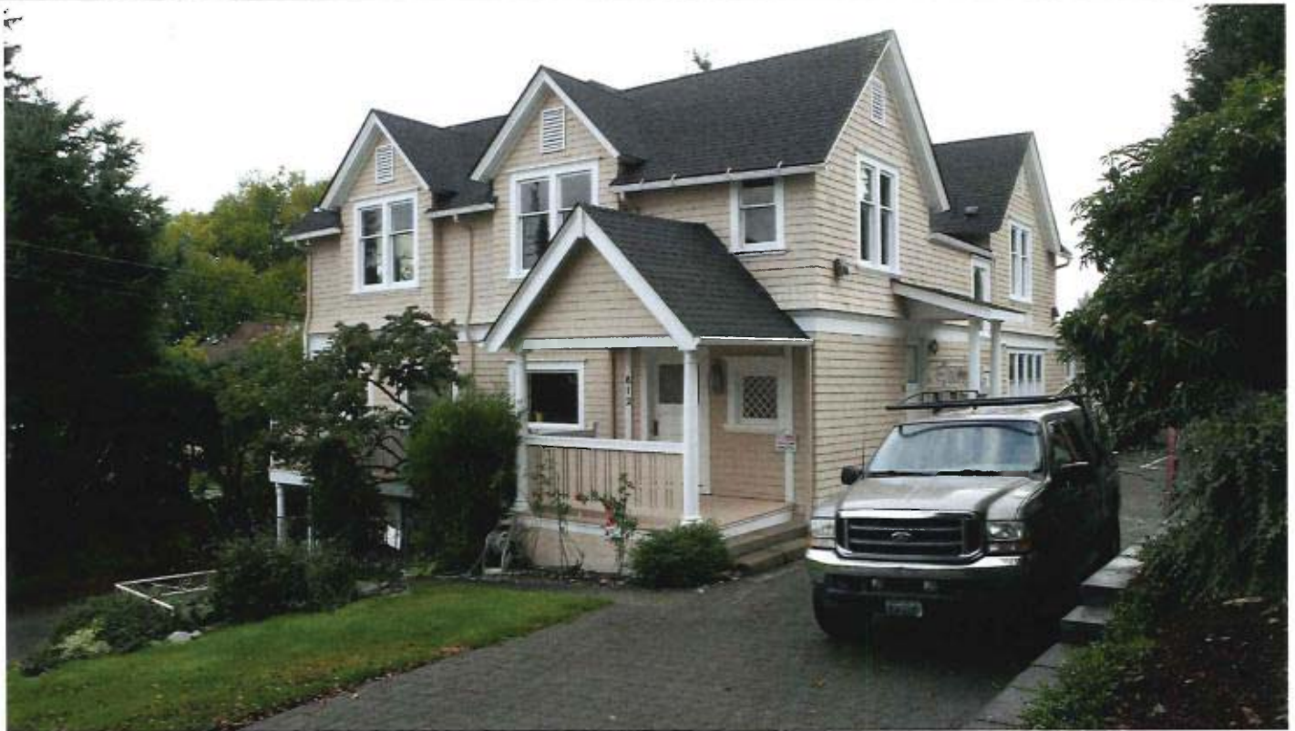
Southwest corner, September 2019.
