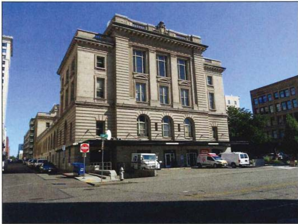
Figure 7. 1102 A Street, south elevation (C. Beckner 2019).
