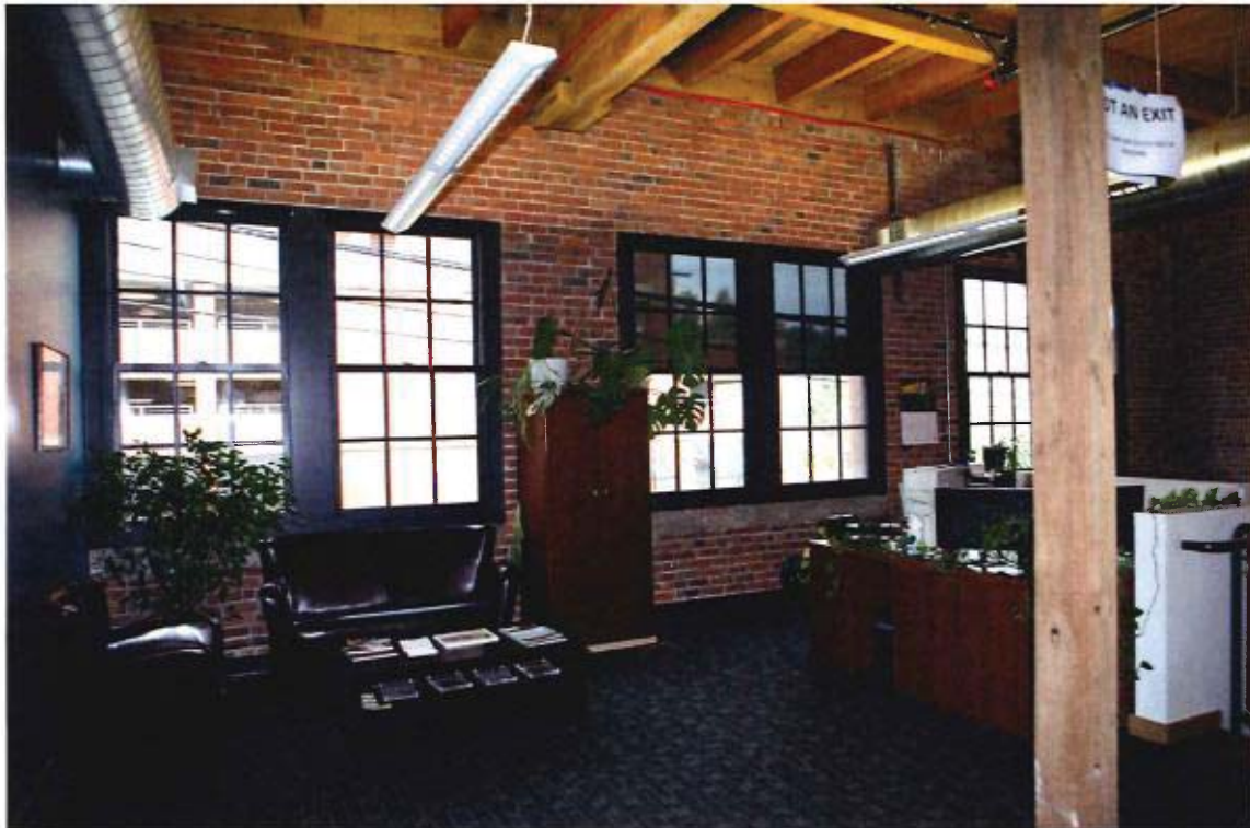
3rd floor, looking northwest at west wall. Roof/structural reinforcements visible. 2019.
