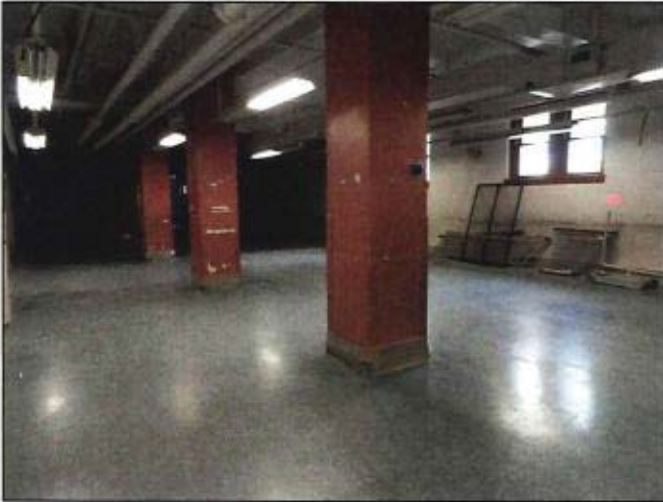
Figure 8. Basement level volumes before rehabilitation (2012).
