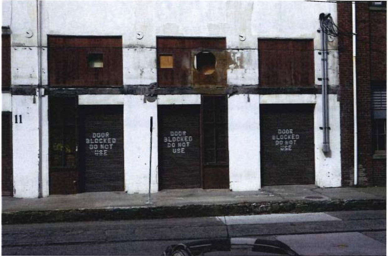
East facade detail. 2013.
