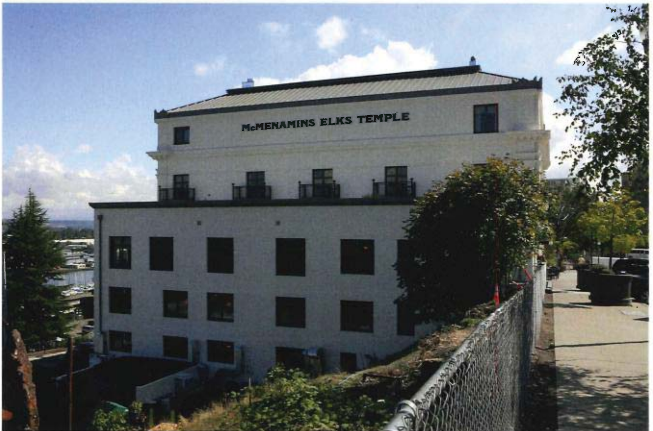
North facade showing completed work, 2019.
