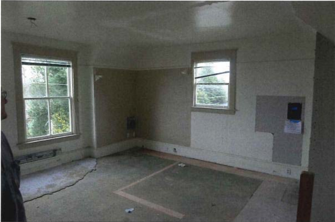
Interior, upper floor, typical apartment. March 2017.
