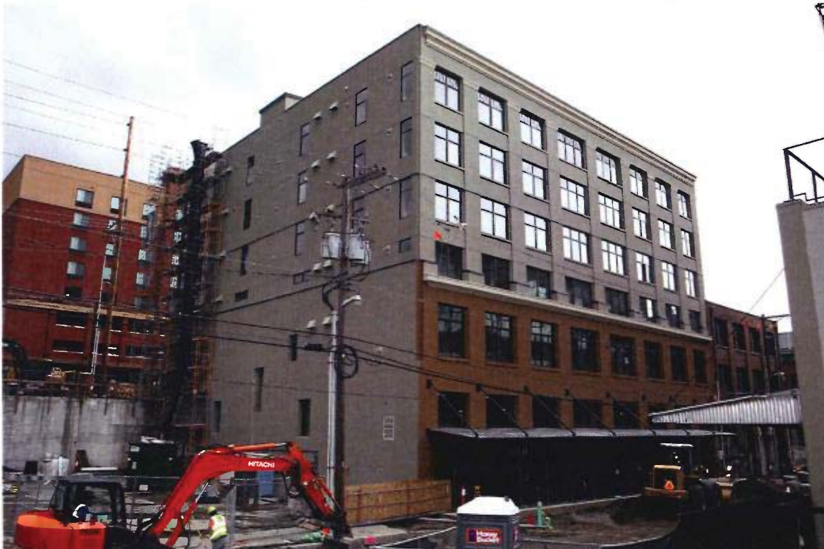
Southeast corner, September 2019. Four upper stories added.
