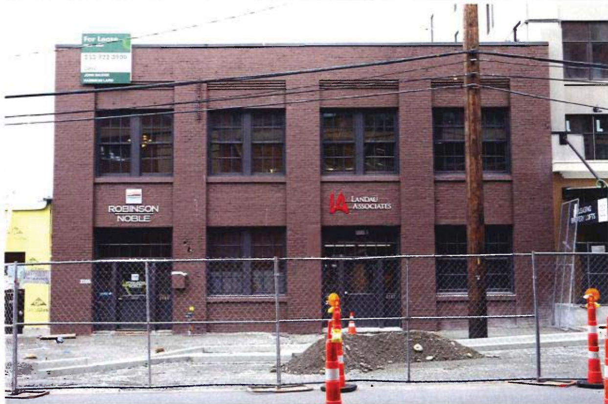
West facade, showing completed work, September 2019.
