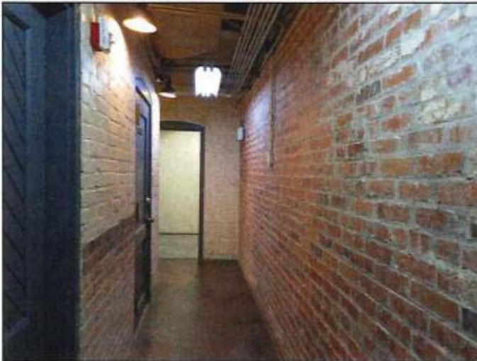
Figure 12. Basement corridors with original brick and wood doors (2019).
