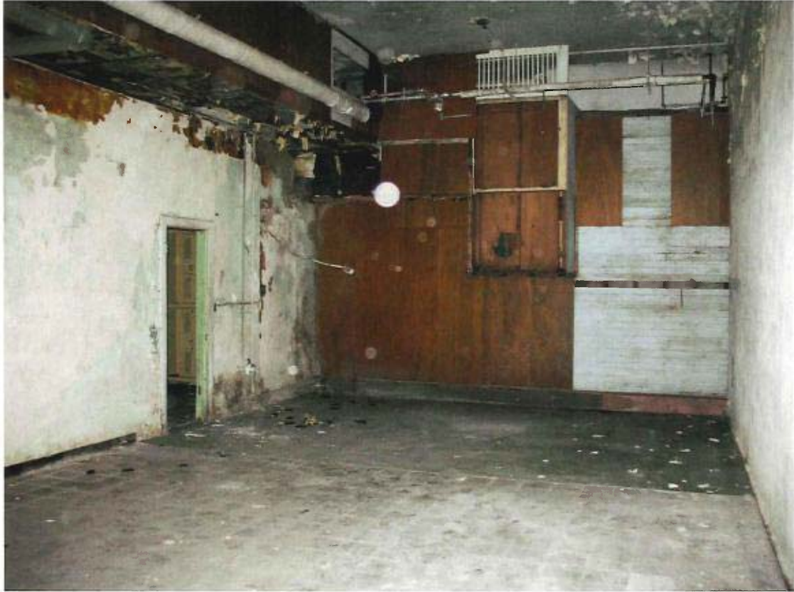
Basement of Annex, northeast corner pre-renovation. 2017.
