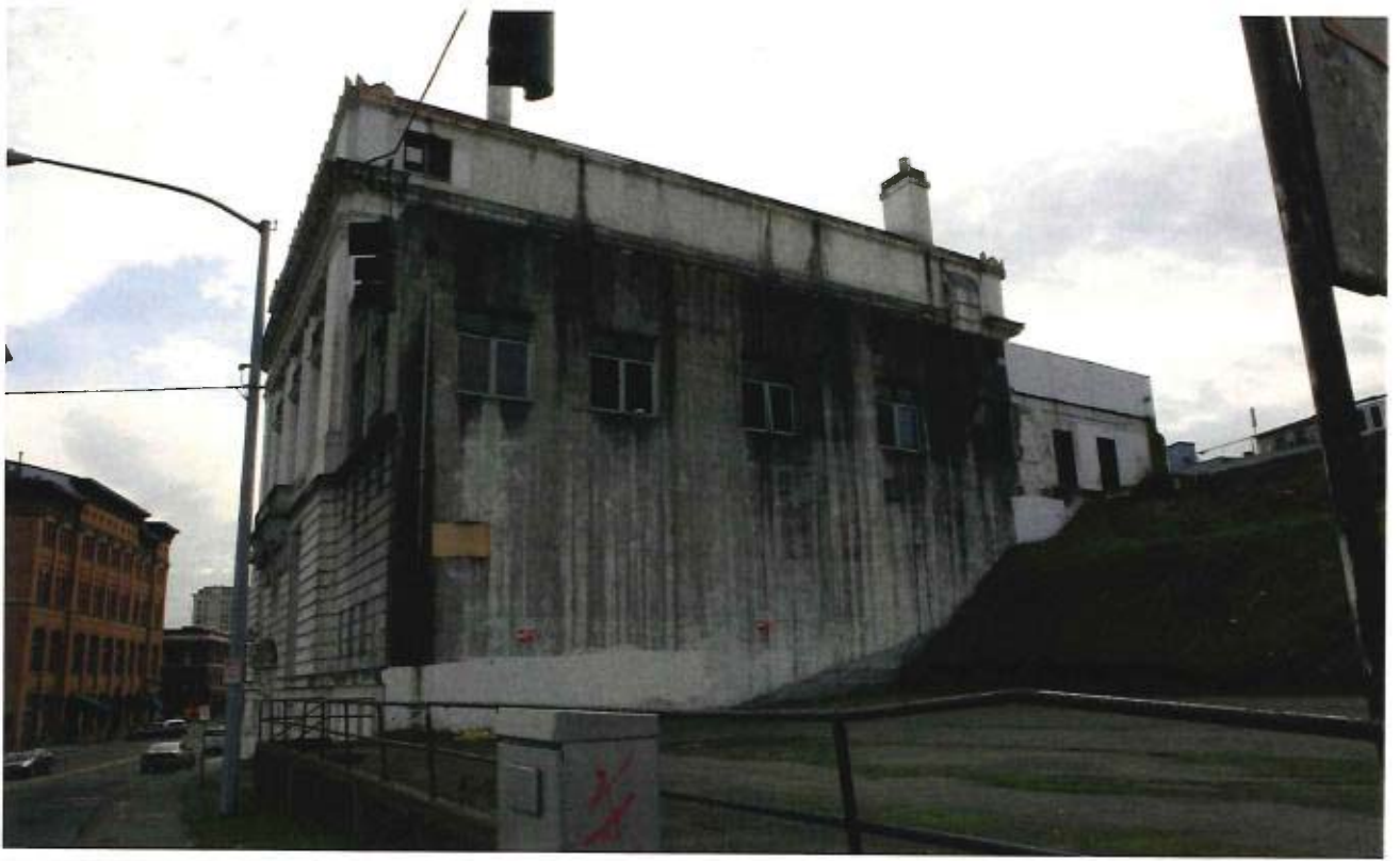
Northeast corner pre-work, 2017.
