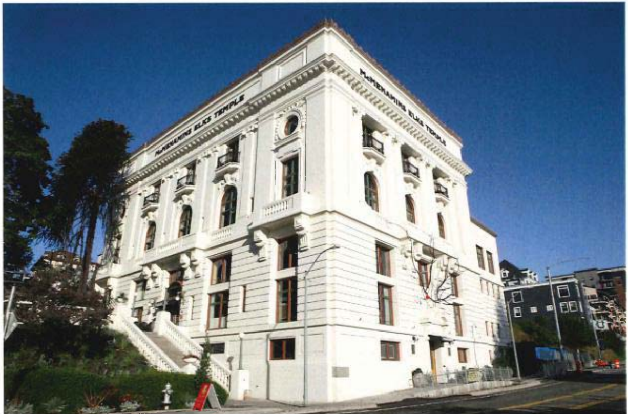
Southeast corner after work, 2019.
