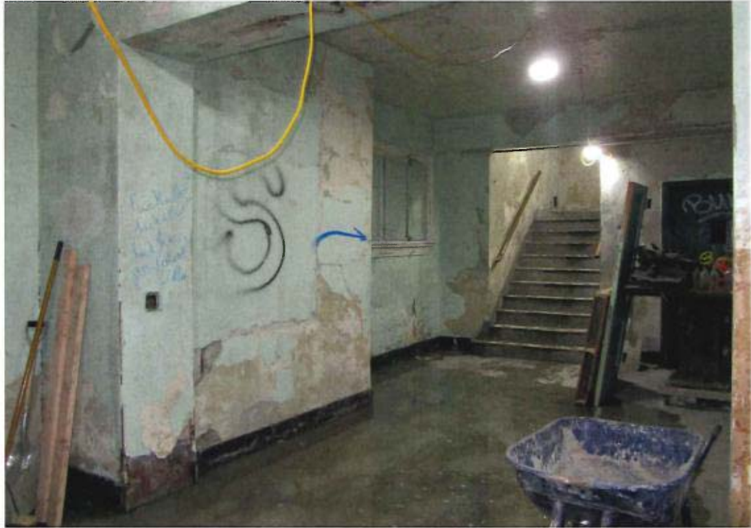
Entry hall at Commerce Street (basement), looking south/southeast. 2017.
