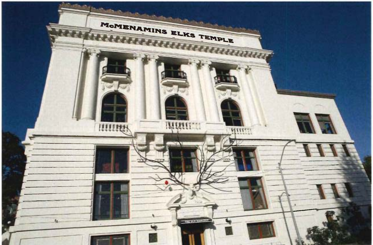
East facade including north annex, showing completed work. 2019.
