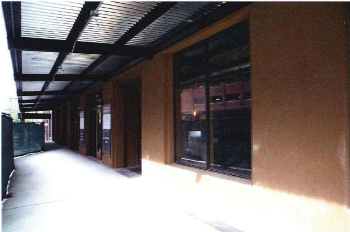
West facade detail, completed work. (2019)
