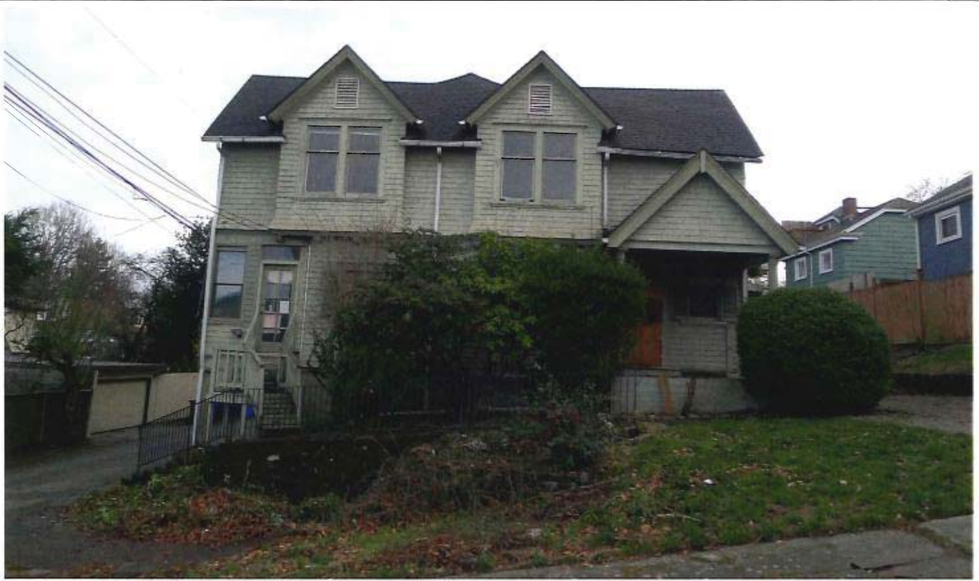
Front (west) facade, March 2017.
