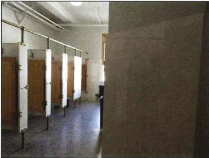
Figure 49. Original restroom, restored, fourth floor (2019).
