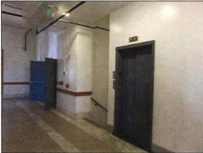
Figure 33. Third floor elevator and stairs with added fire doors (2019).
