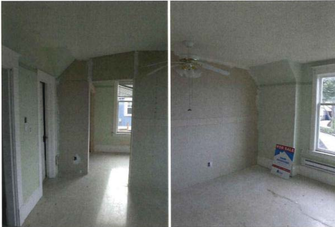
Interior, upper floor, typical apartment. Southwest corner unit, looking south. March 2017.
