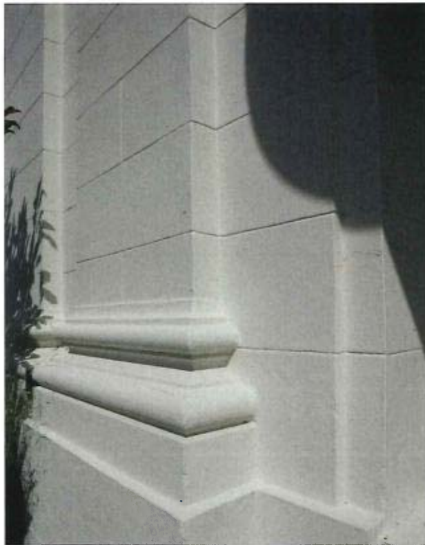
West facade detail, showing exterior walls repaired. 2019.
