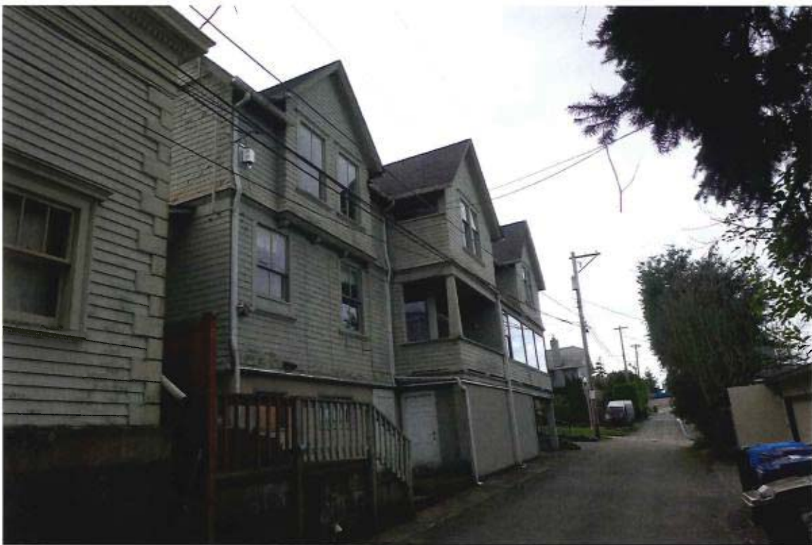
Northeast corner and north (alley) facade, March 2017.
