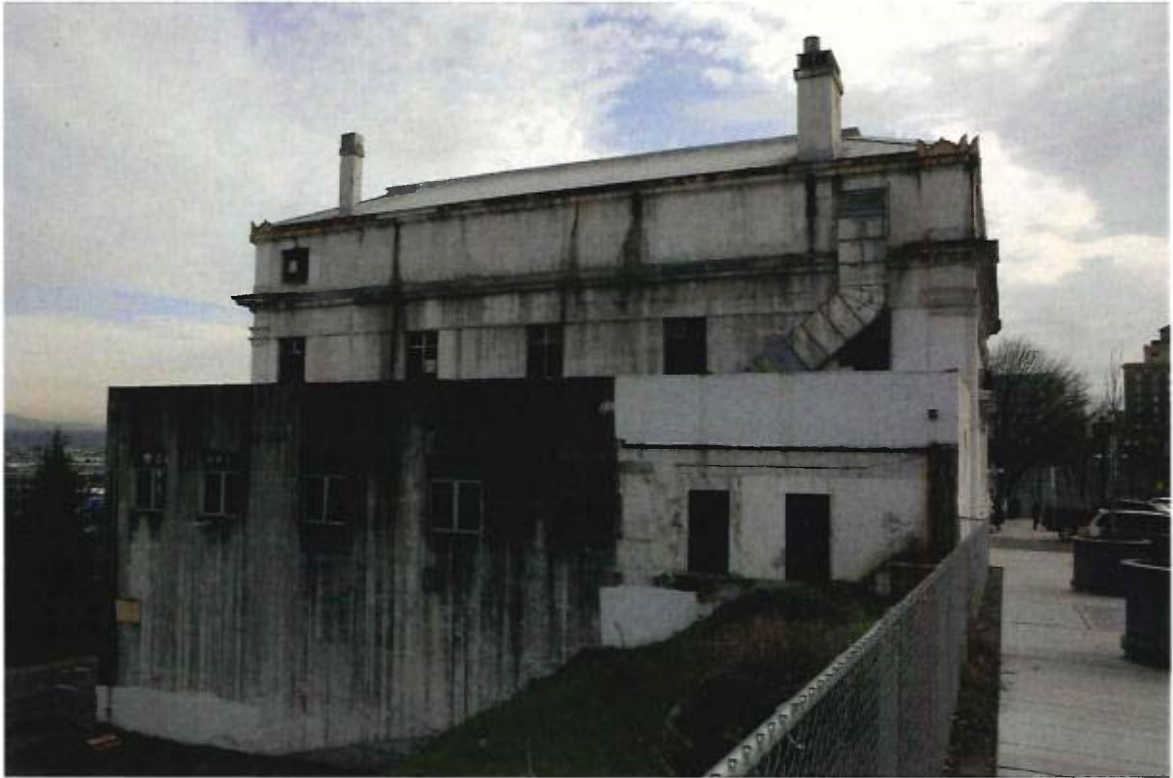
North facade pre-work, 2017.
