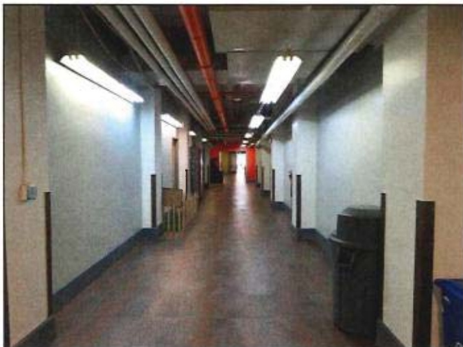
Figure 14. Basement corridor providing access to commercial spaces (2019).
