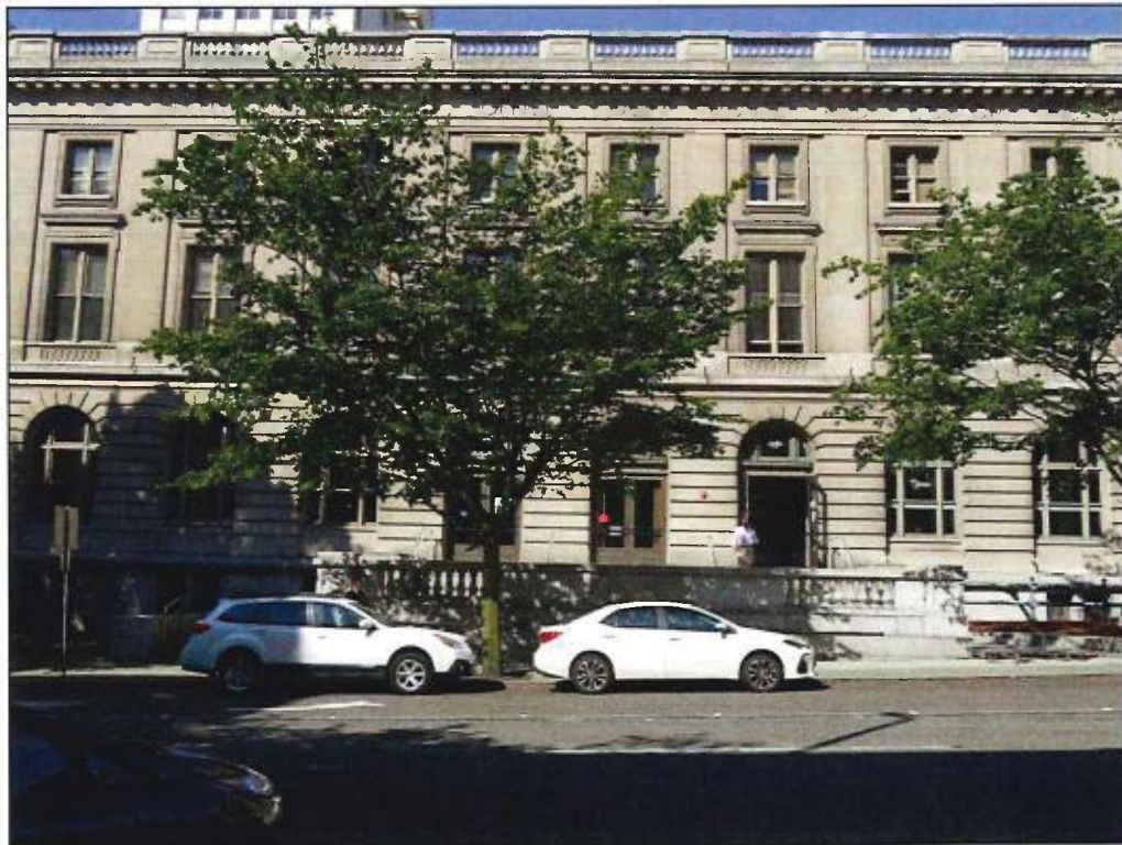
Figure 5. 1102 A Street, east elevation (C. Beckner, 2019).
