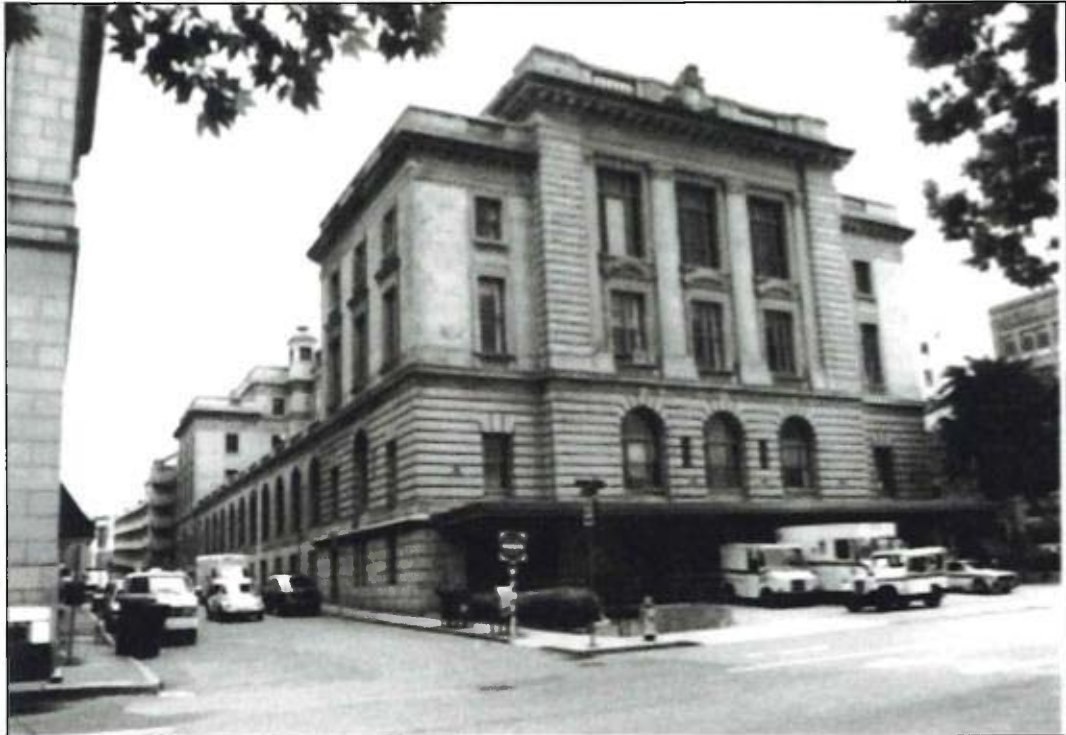
Figure 6. 1102 A Street, south elevation (Kolva and Franks, 1989).
