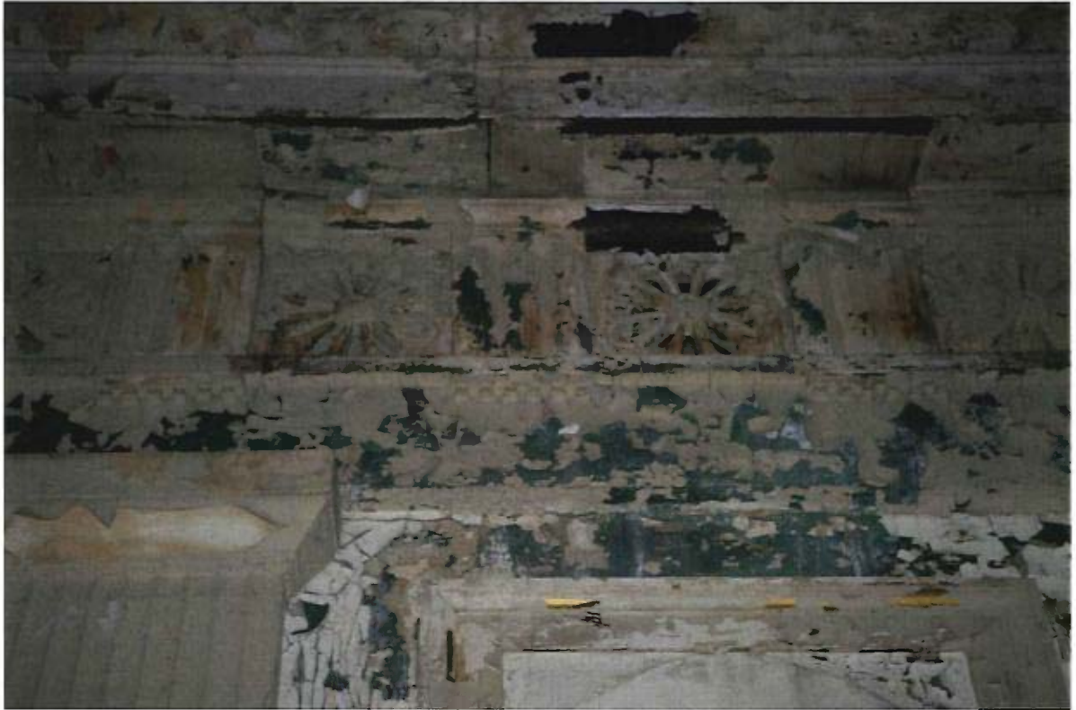
Former Lodge Room (top floor), upper wall and ceiling detail. 2016.
