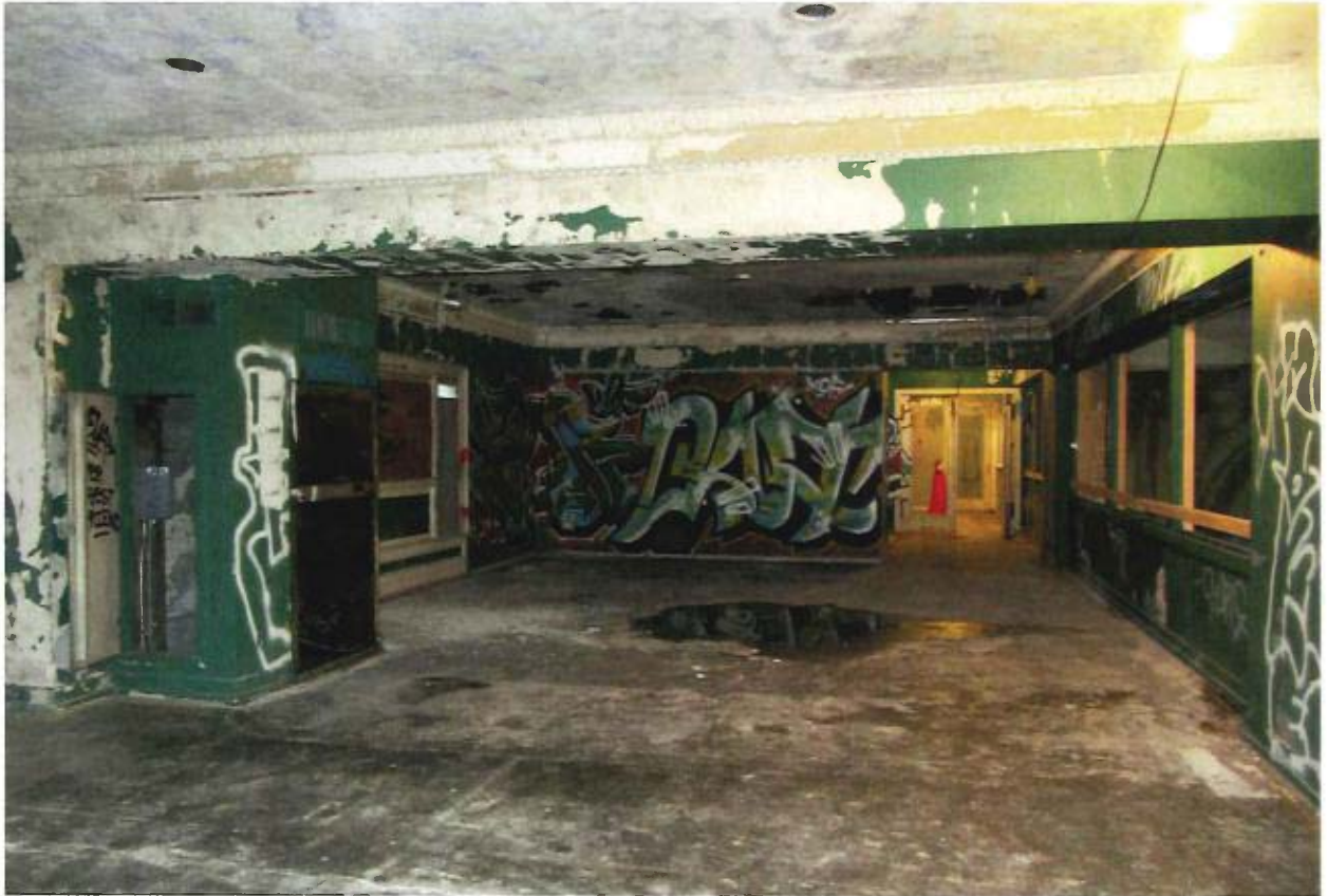
Mezzanine between ballroom and Broadway level, looking west. 2016.
