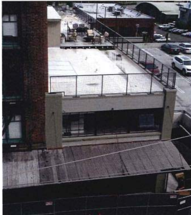
West facade and roof in September 2019, showing completed work.
