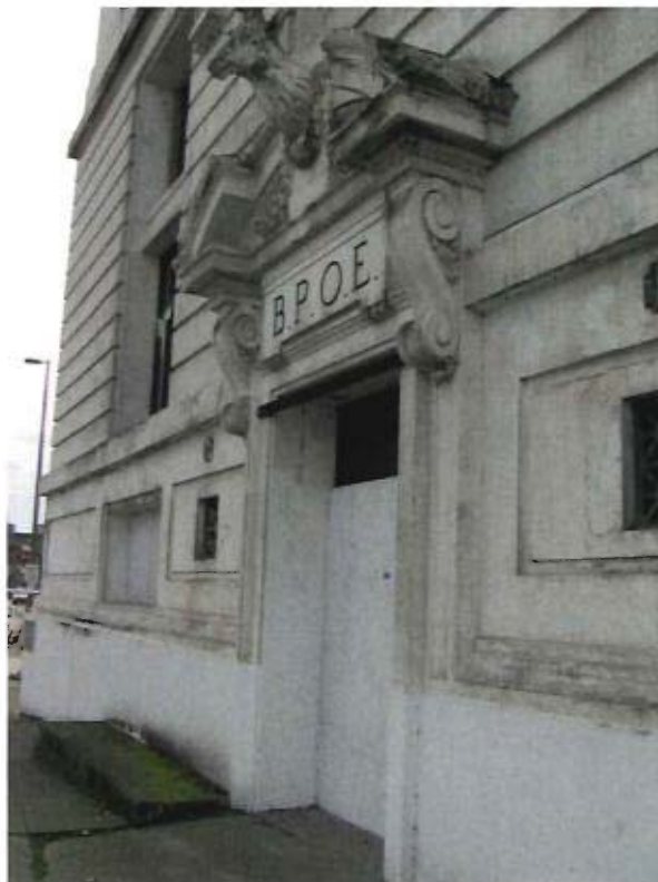
Commerce Street (east) entry, looking southwest. 2017.
