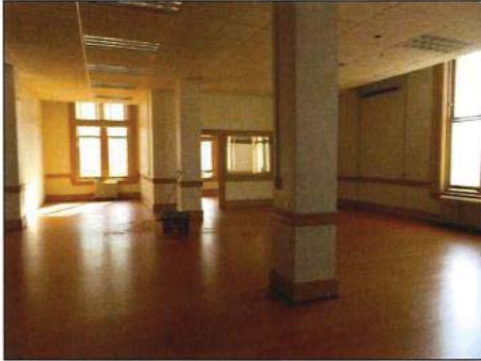
Figure 36. Rehabilitated office space, third floor (2019).
