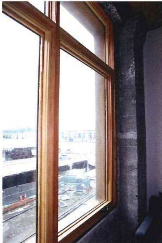
Replacement window detail, looking southeast. 2019.
