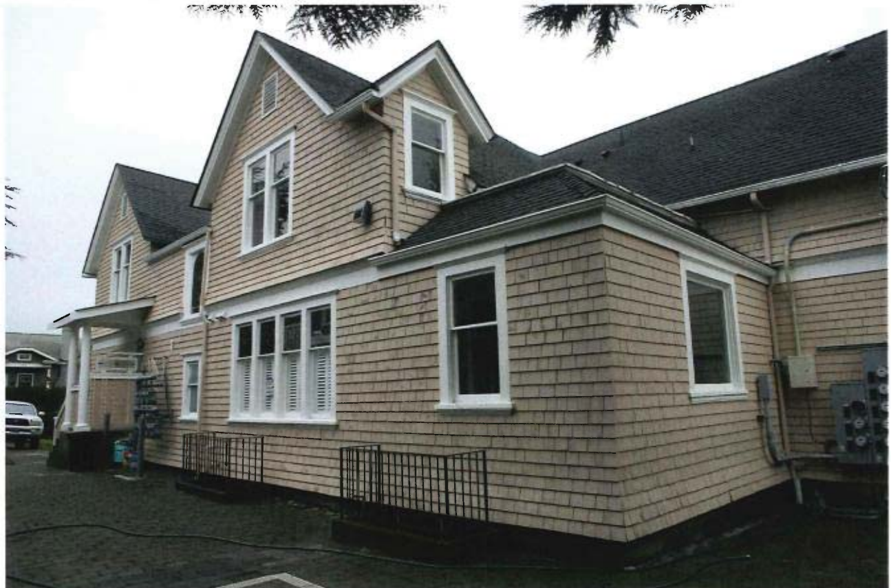
South facade, September 2019.
