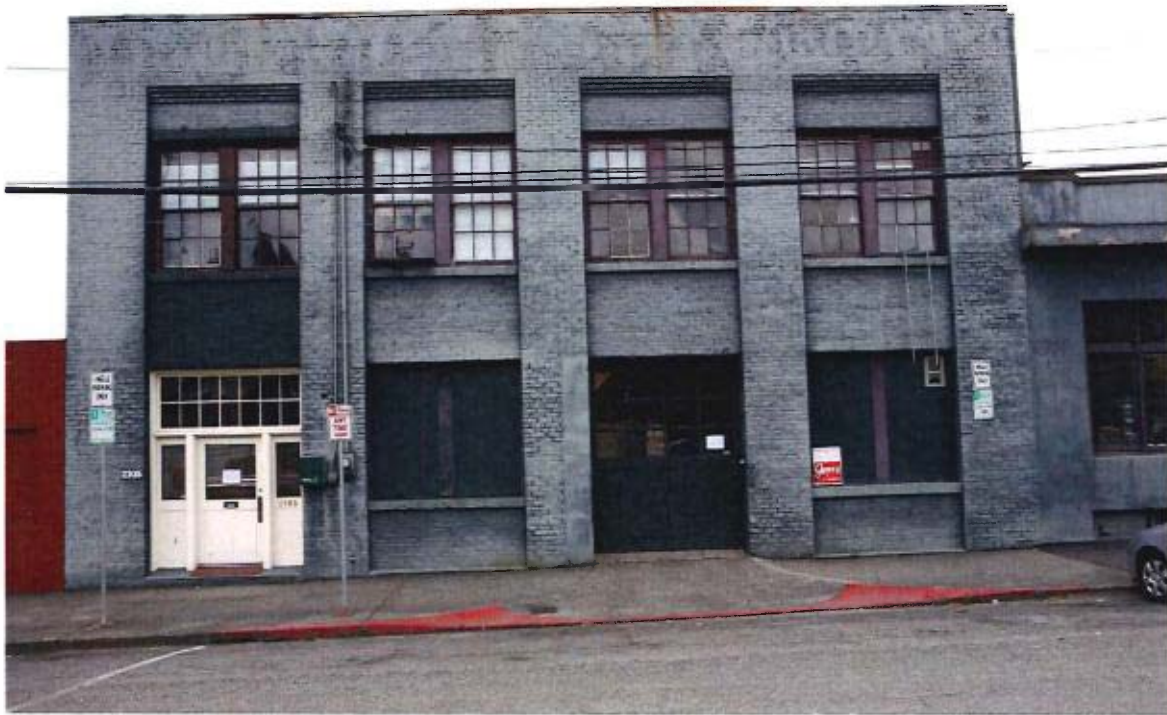
West facade, pre-work. (August 2014)
