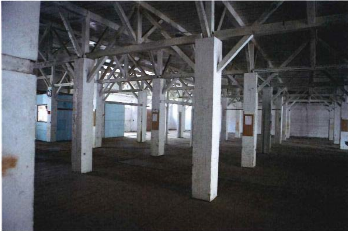
2nd floor, typical open space with large wood posts. 2013.
