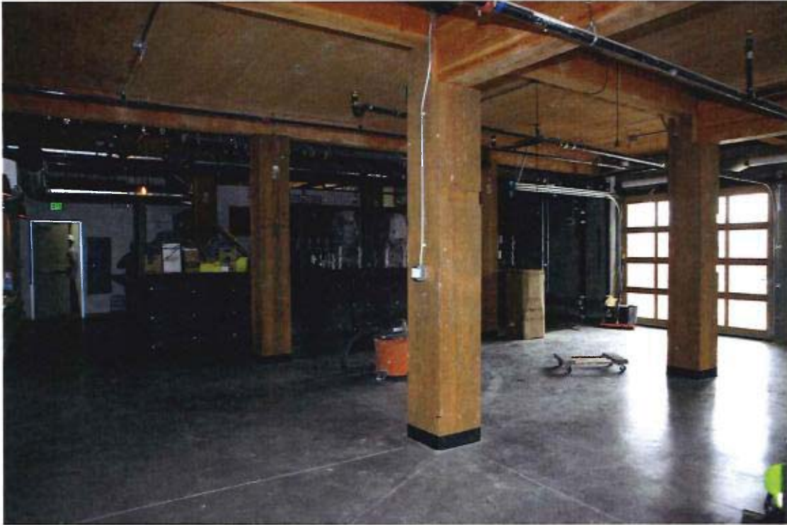
New commercial space, SW corner of 2nd floor (Incline Cider). 2019.
