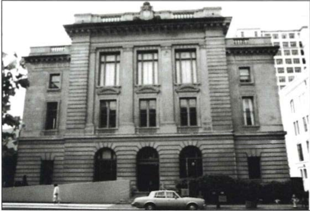
Figure 2. 1102 S A Street, north elevation (Kolva and Franks, 1989).
