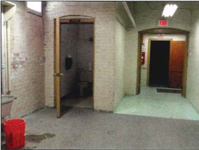
Figure 9. Basement level restroom and painted brick walls (2012).
