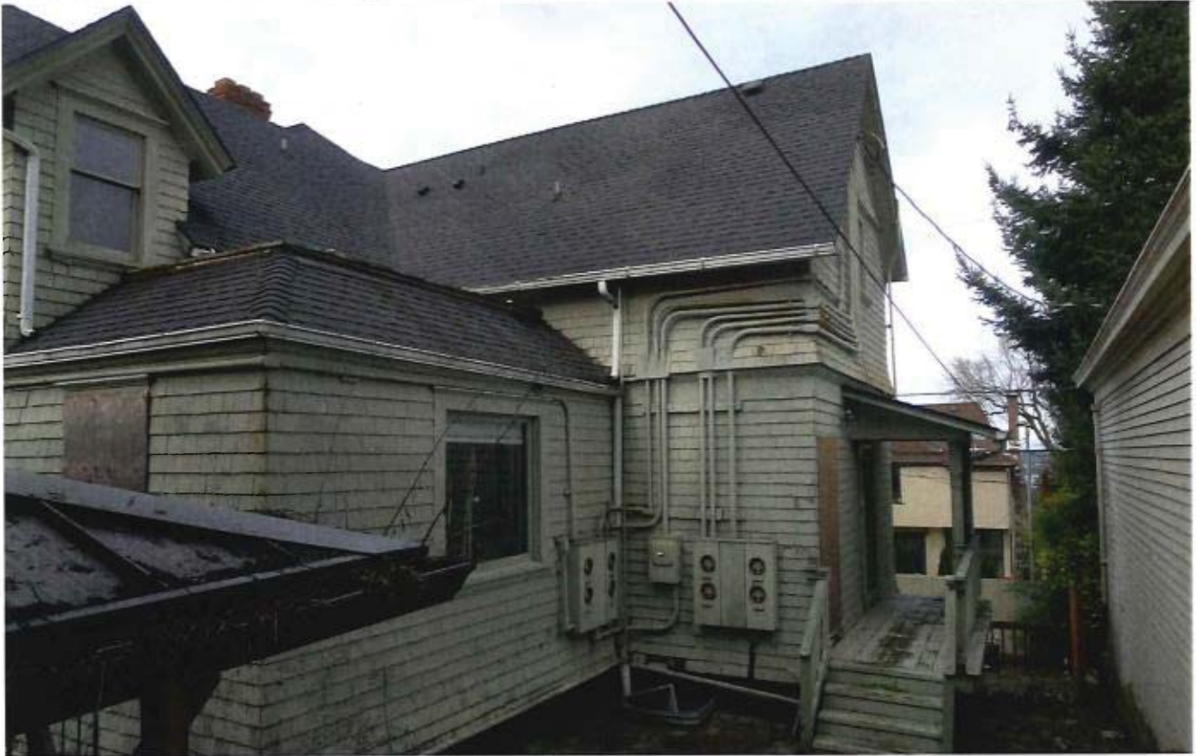
Southeast corner, March 2017.
