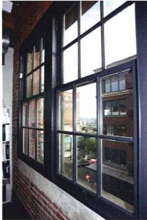
Window repair detail, looking northeast. September 2019.
