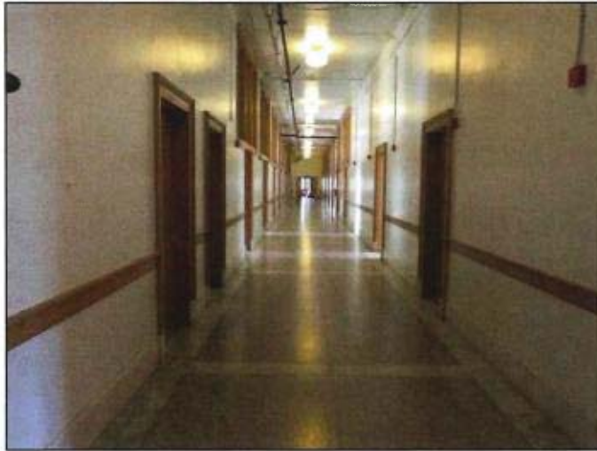
Figure 39. Third floor corridor, with all original materials in place (2019).
