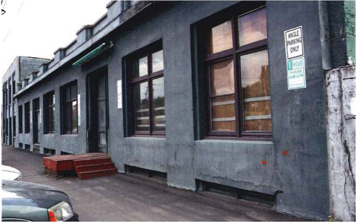
West facade detail, pre-work. (2013)
