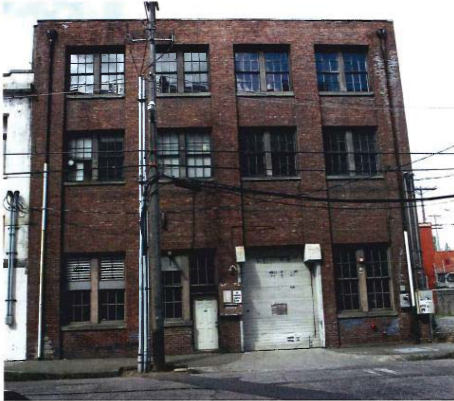
East facade in August 2014, pre-work.
