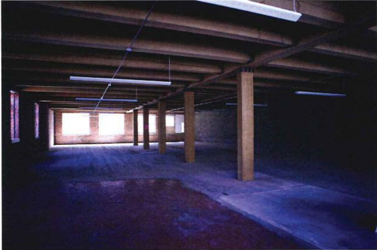
2nd floor (South C St. level) looking east pre-work, 2013.
