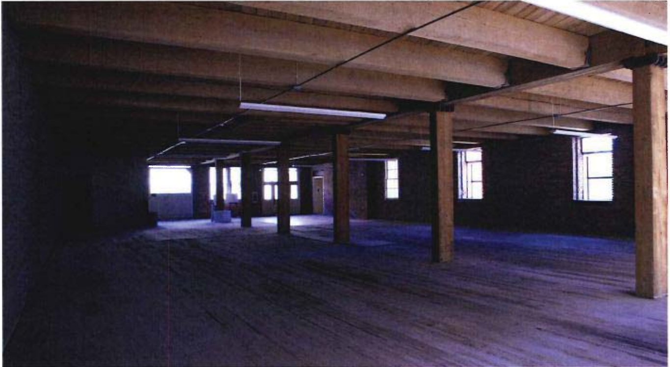
2nd floor (South C St. level) looking northwest pre-work, 2013.
