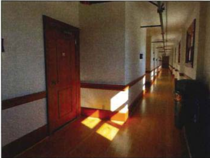
Figure 57. Rehabilitated fifth-floor corridor (2019).
