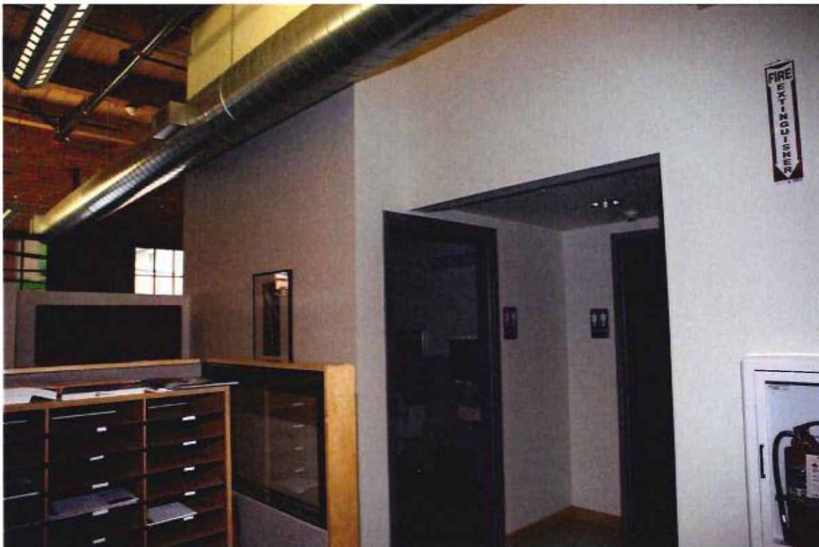
Typical new (added) restrooms, 3rd floor. 2019.
