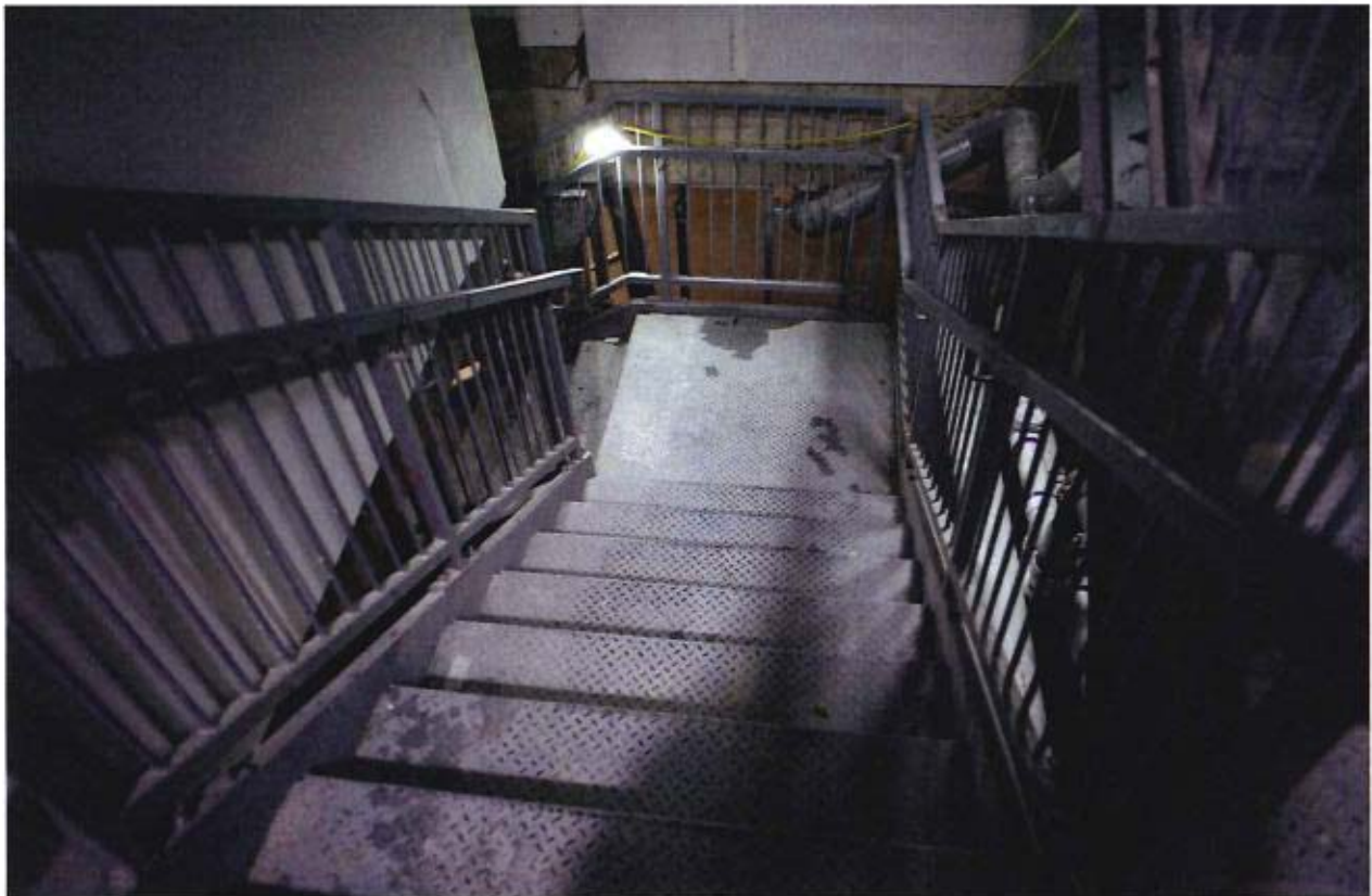
Typical new stairwell. September 2019.
