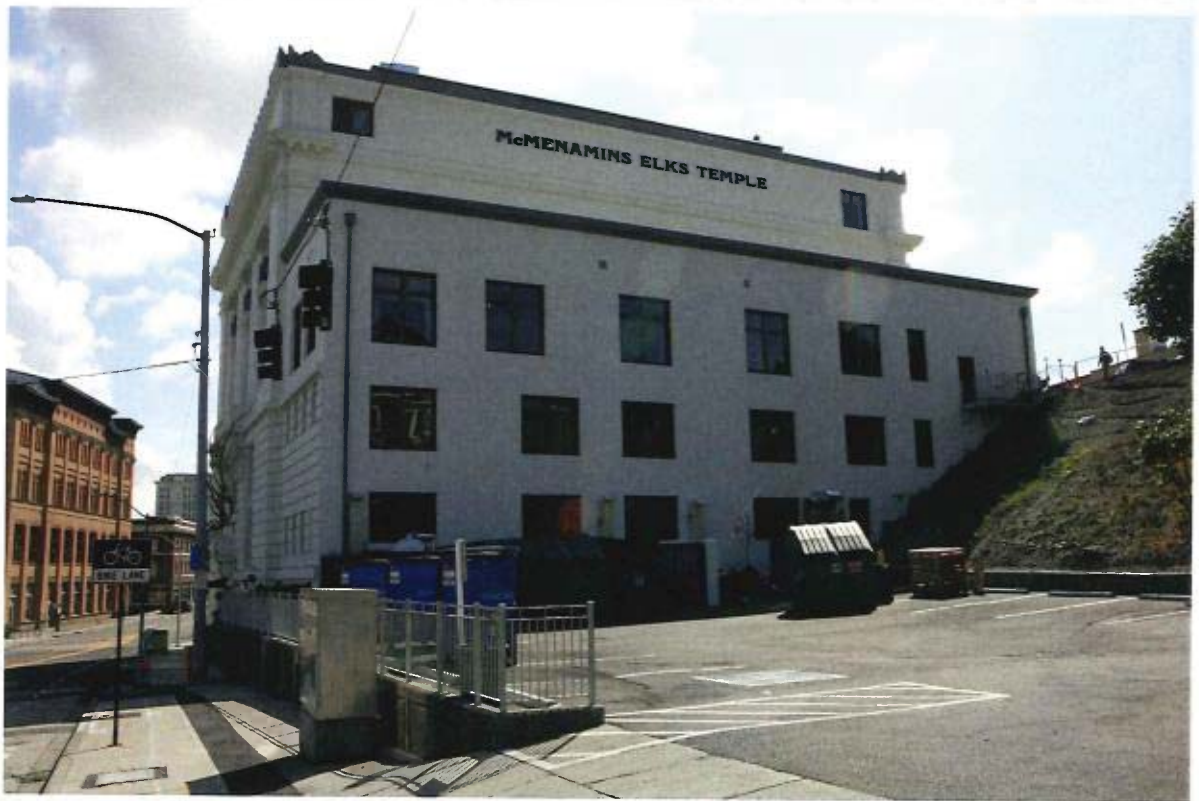
Northeast corner showing completed work, 2019.
