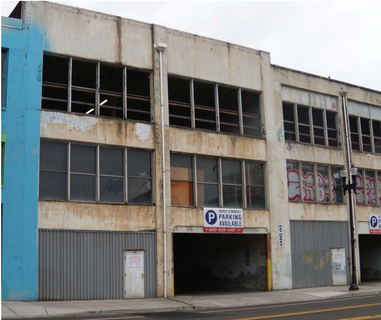
EXISTING FACADE ALONG COMMERCE STREET
