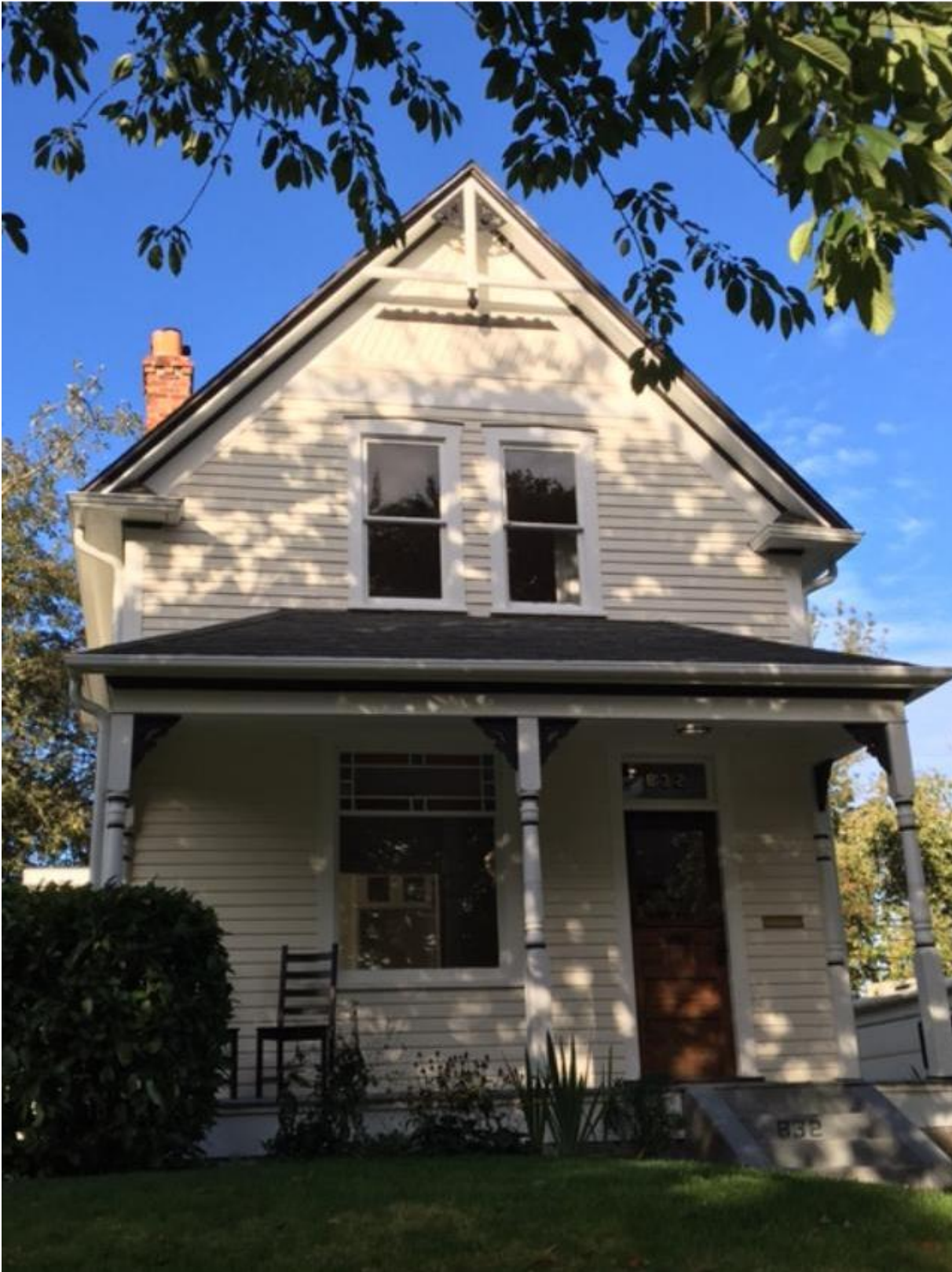
Figure 9. Front (East) Façade, 2021 (Collection of Scott Armstrong)
