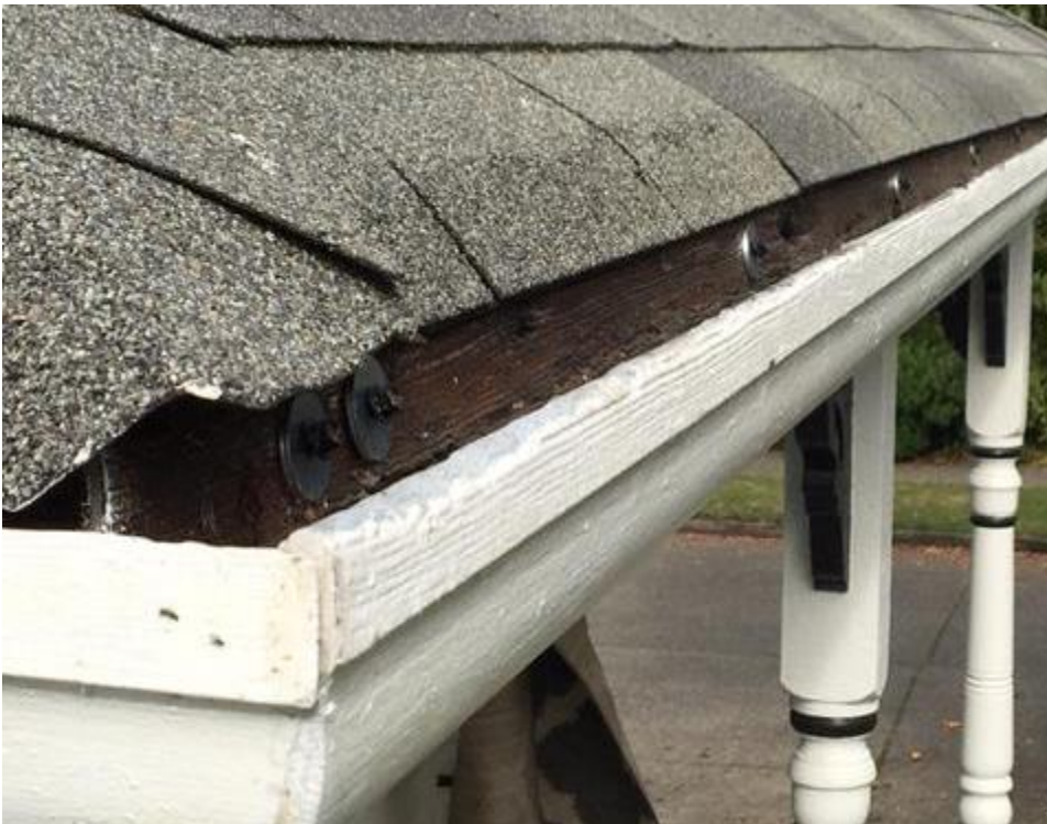
Figure 11. Original restored Boston-patterned cedar gutters, front porch roof (Collection of Scott Armstrong)
