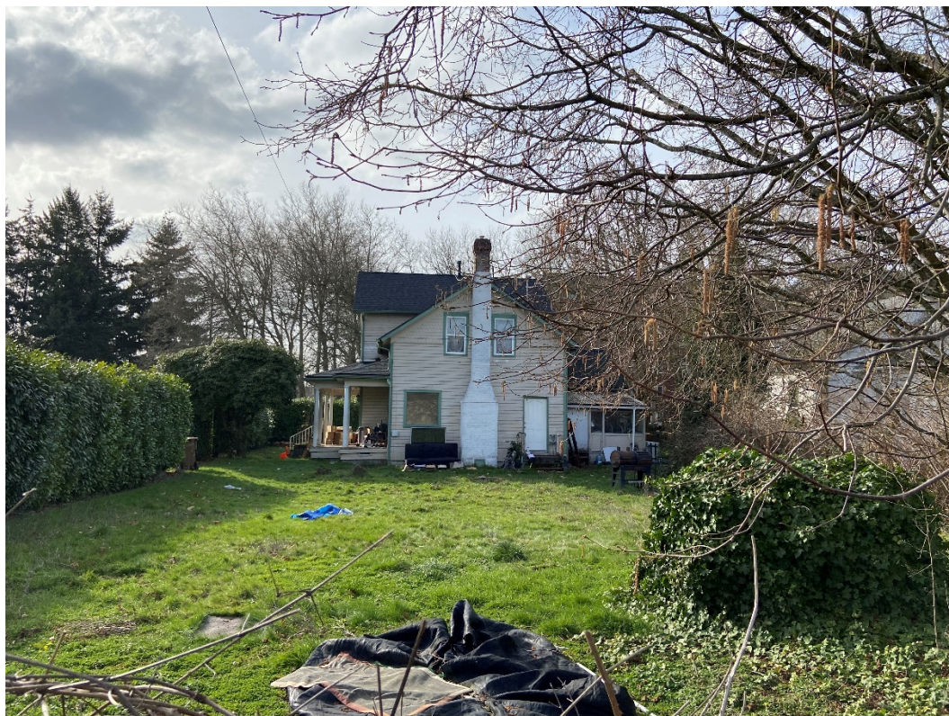
Fig. 4. East Elevation from alley showing side yard.
