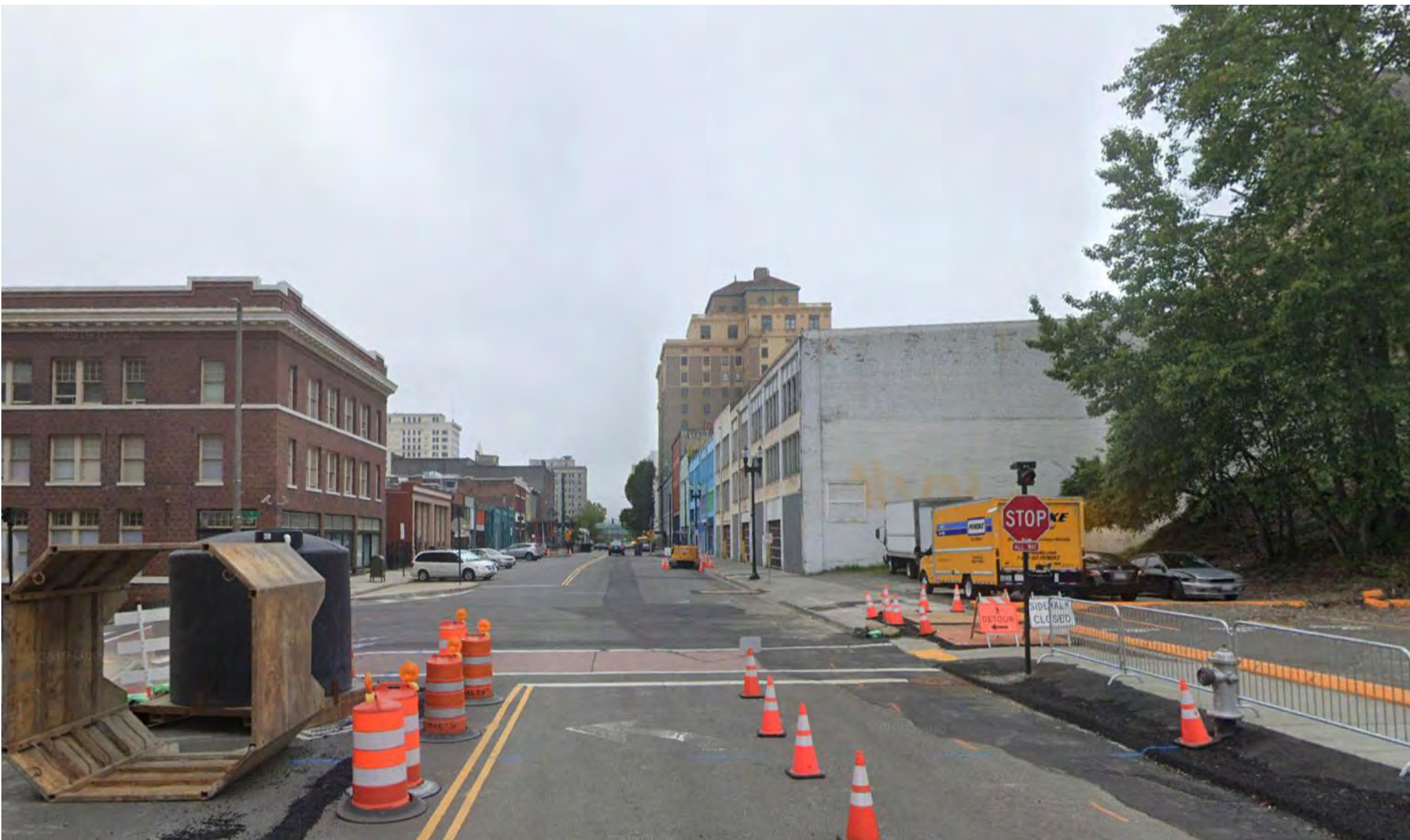
COMMERCE - EXISTING VIEW SOUTH
