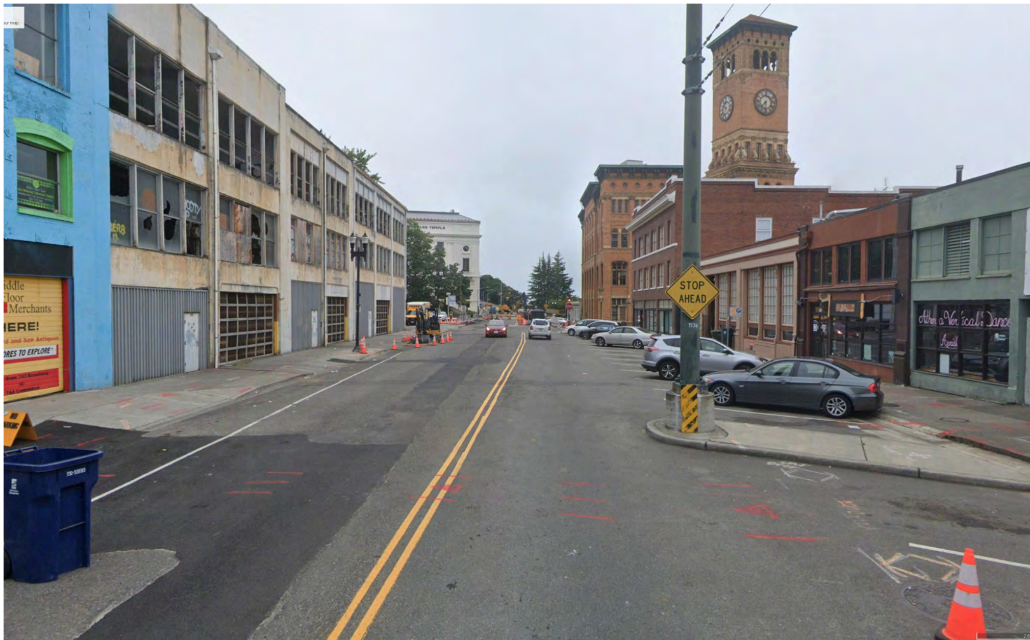
COMMERCE - EXISTING VIEW NORTH
