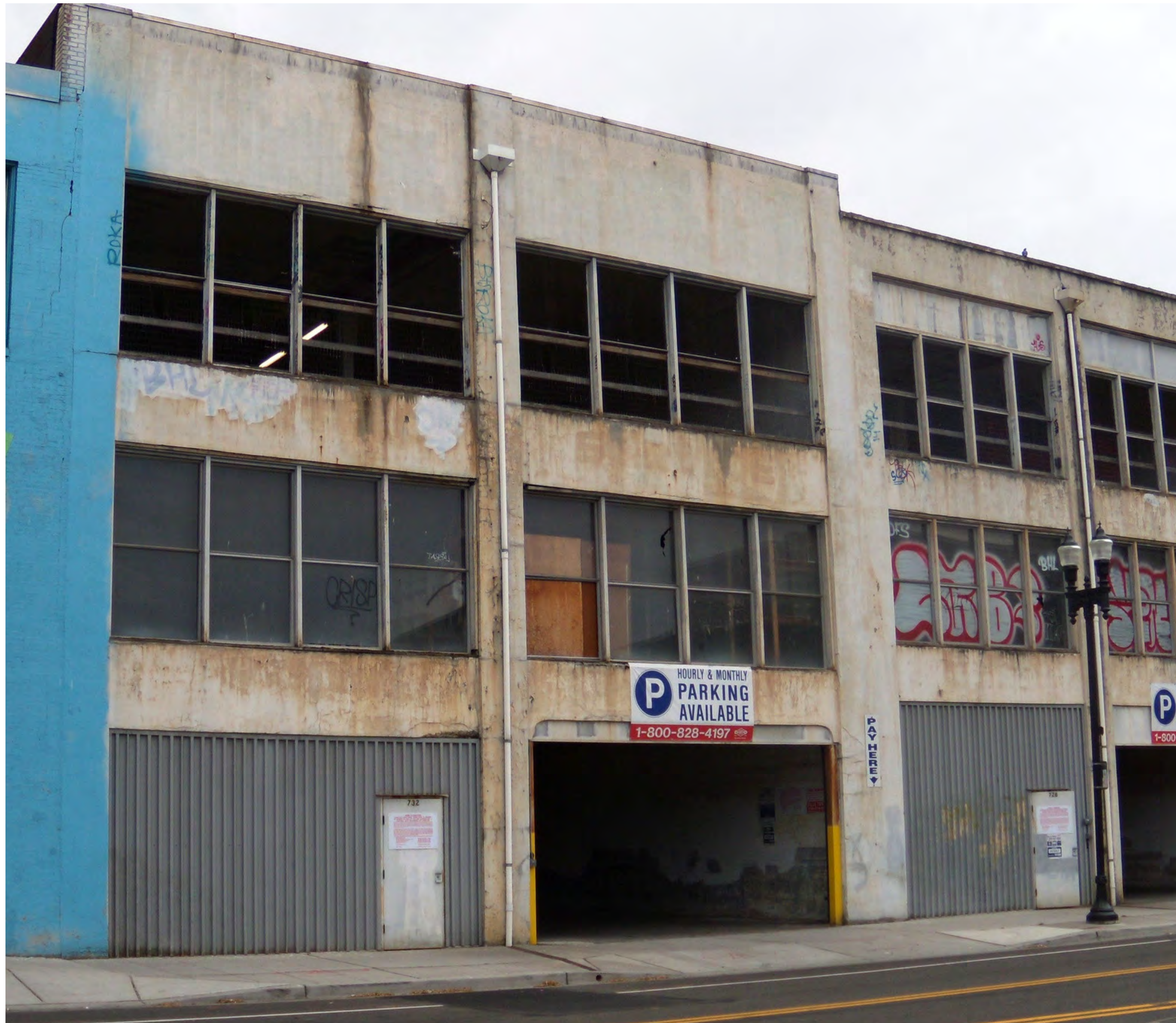
EXISTING FACADE ALONG COMMERCE STREET
