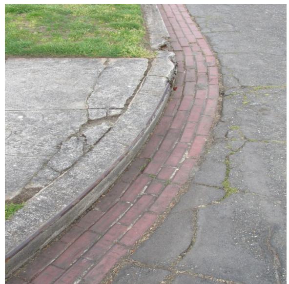
Brick gutter detailing
