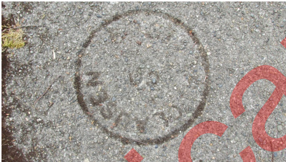
Makers marks, dated contractor stamps
