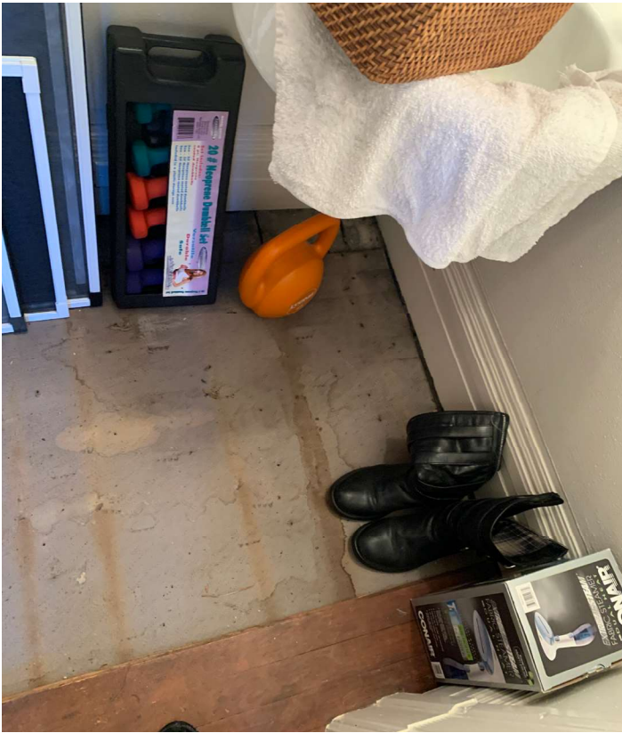
Closet prior to system installation
