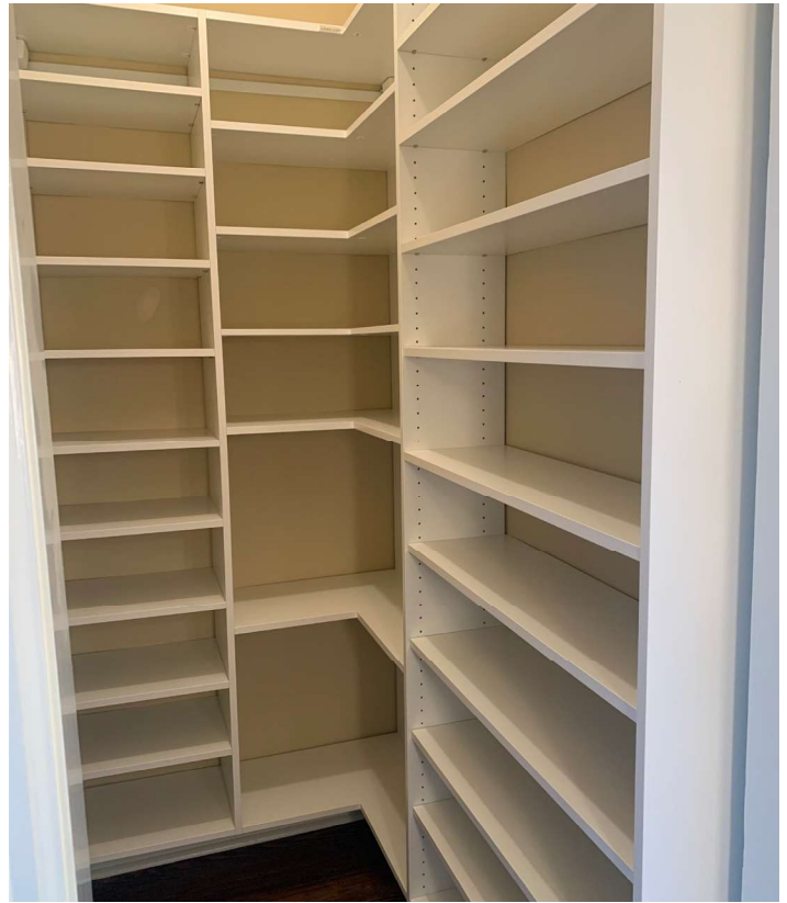
New closet system installed
