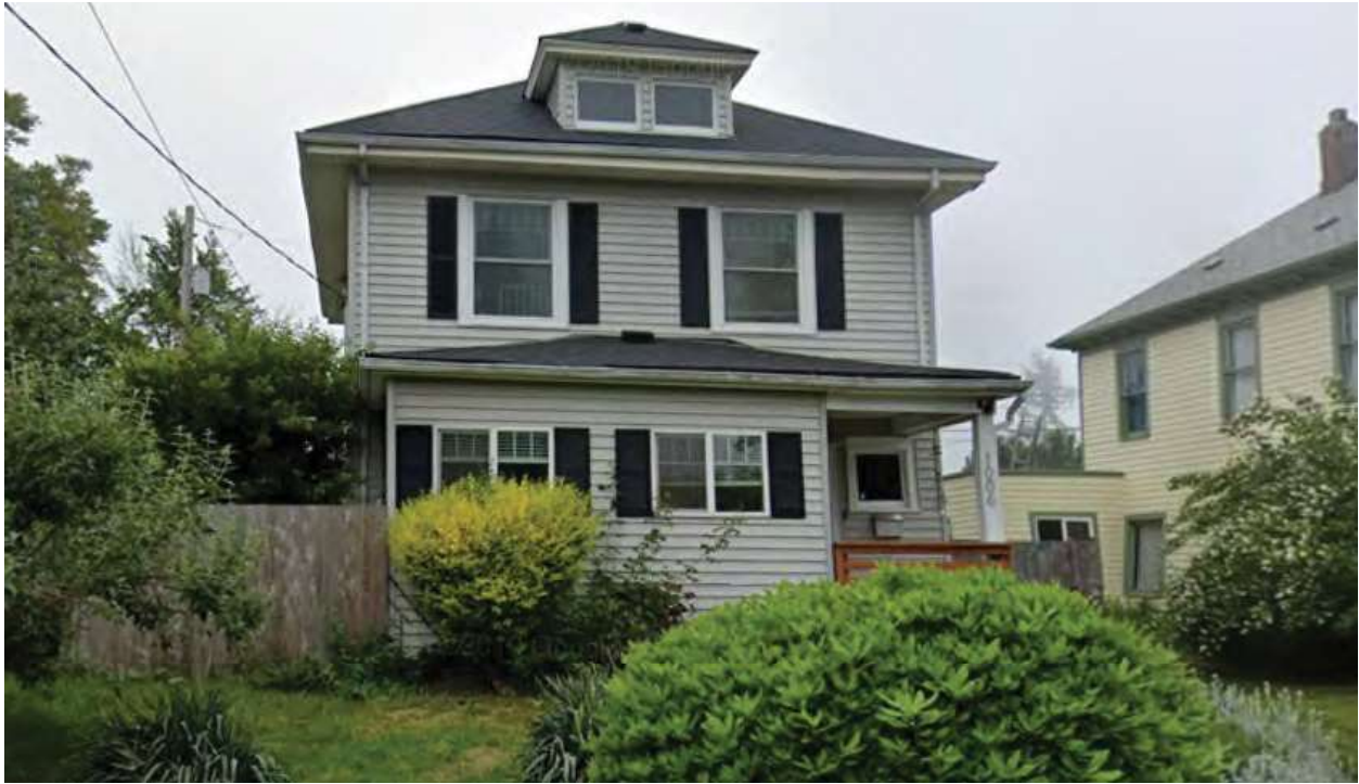
Figure 37. Neighboring house, 1006 S Anderson Street, with similar massing and roof.
