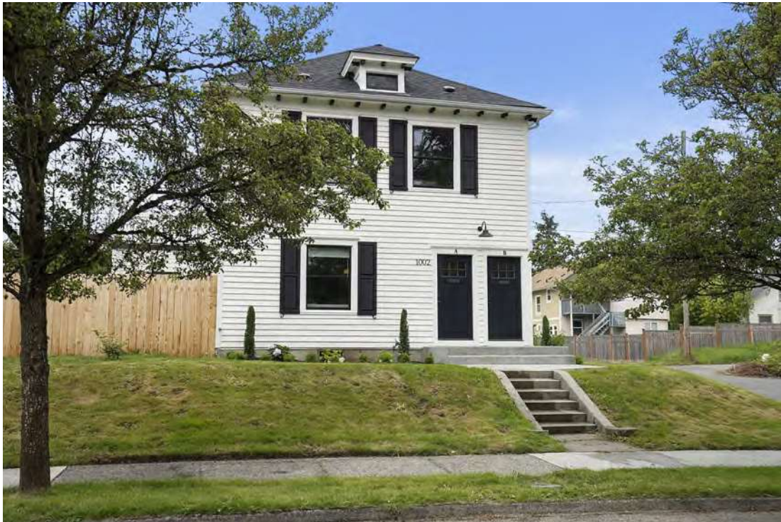
Figure 6. East (main) elevation, 2020.
