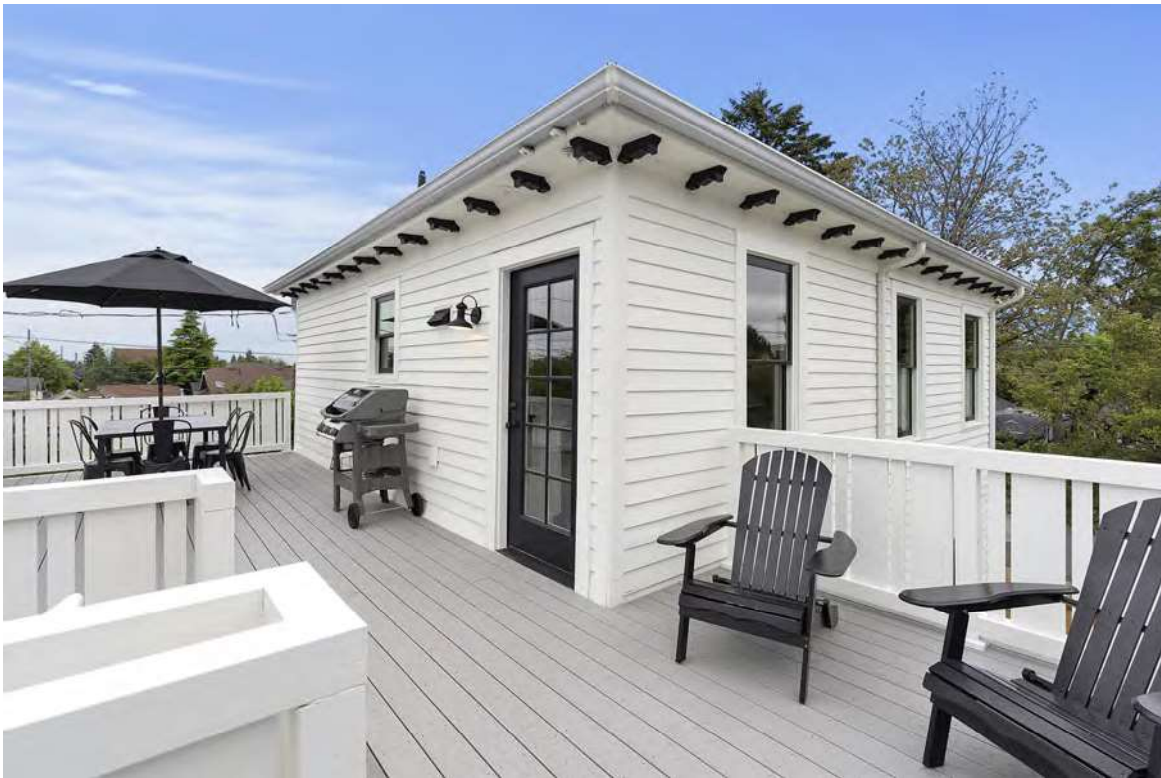
Figure 12. Southwest corner and 2nd floor deck, 2020.
