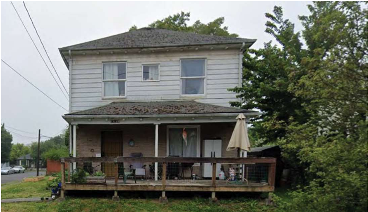
Figure 38. Neighboring house, 1016 S Anderson Street, with similar massing and roof.
