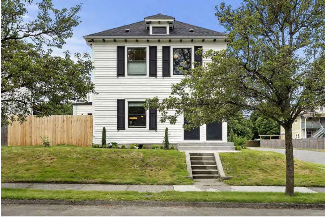
Figure 5. East (main) elevation, 2020.
