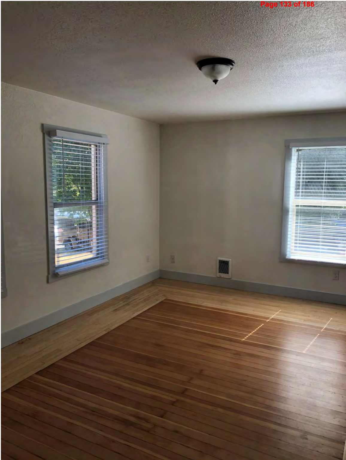
Fig. 37 (After). Newton Apartments, Typical First Floor unit, former Unit 8, original oak/fir flooring, looking southeast. August 2020. Source: Stephen Day Architecture.
