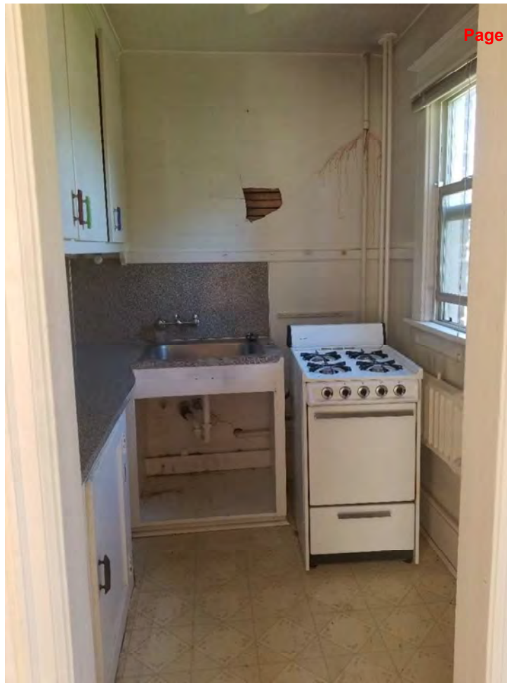
Fig. 38. Newton Apartments, kitchen prior to rehabilitation, Unit 7, looking west, 2018. Source: Owner.
