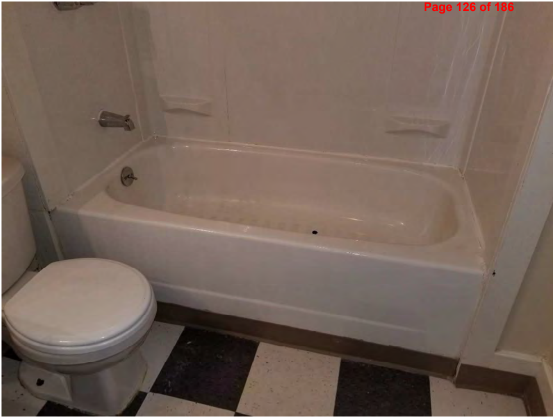
Fig. 34D. Newton Apartments, Basement Unit 18, looking southeast, 2018. Source: Owner.
