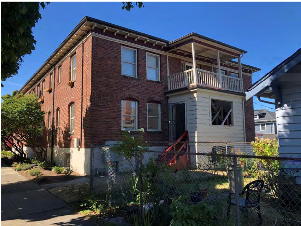
Fig. 9 (After). Newton Apartments, porch at east façade, looking NW. August 2020. Source: Stephen Day Architecture.
