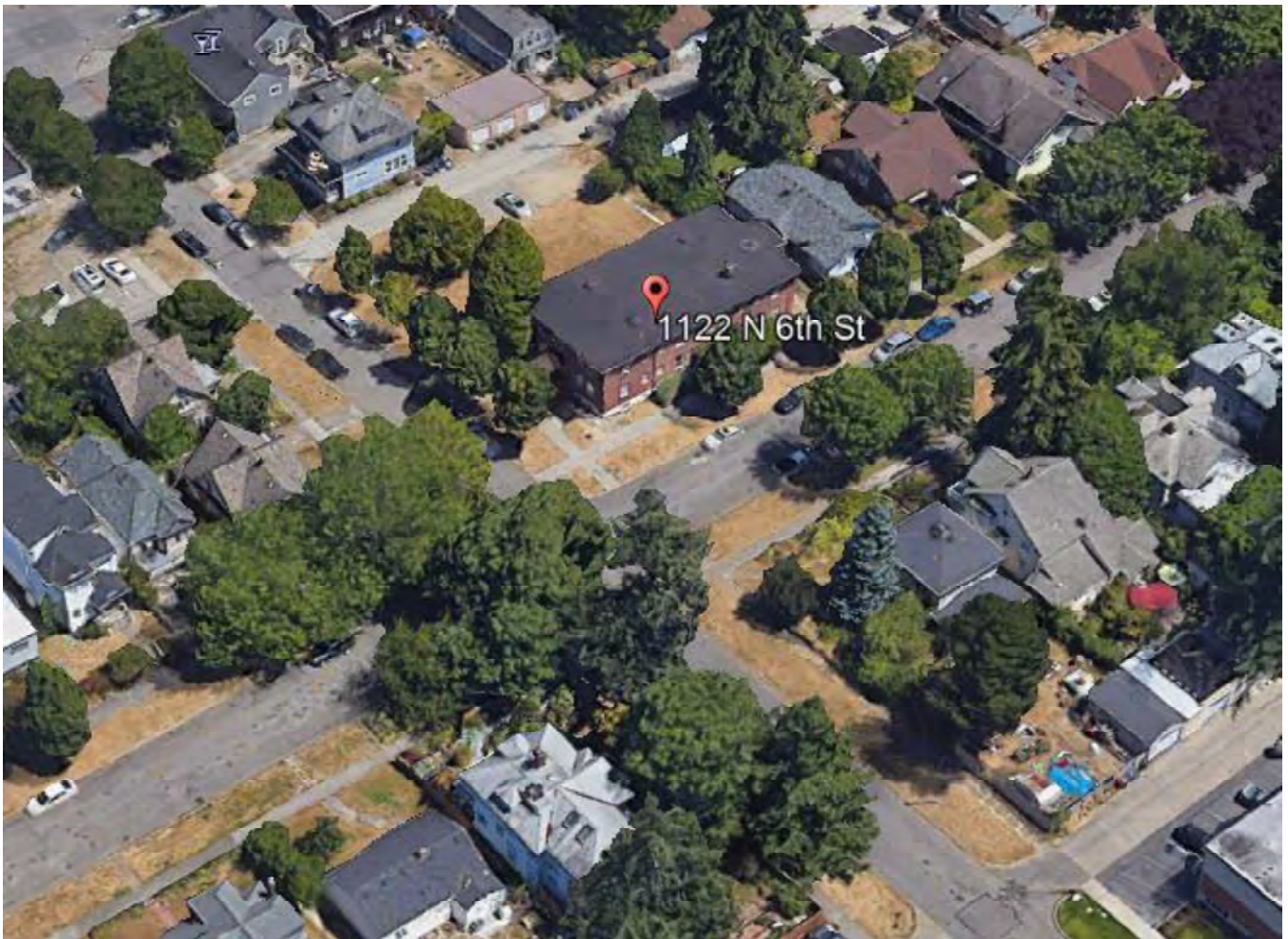
Fig. 5. Aerial view, with location of Newton Apartments indicated. Source: Google Earth.
