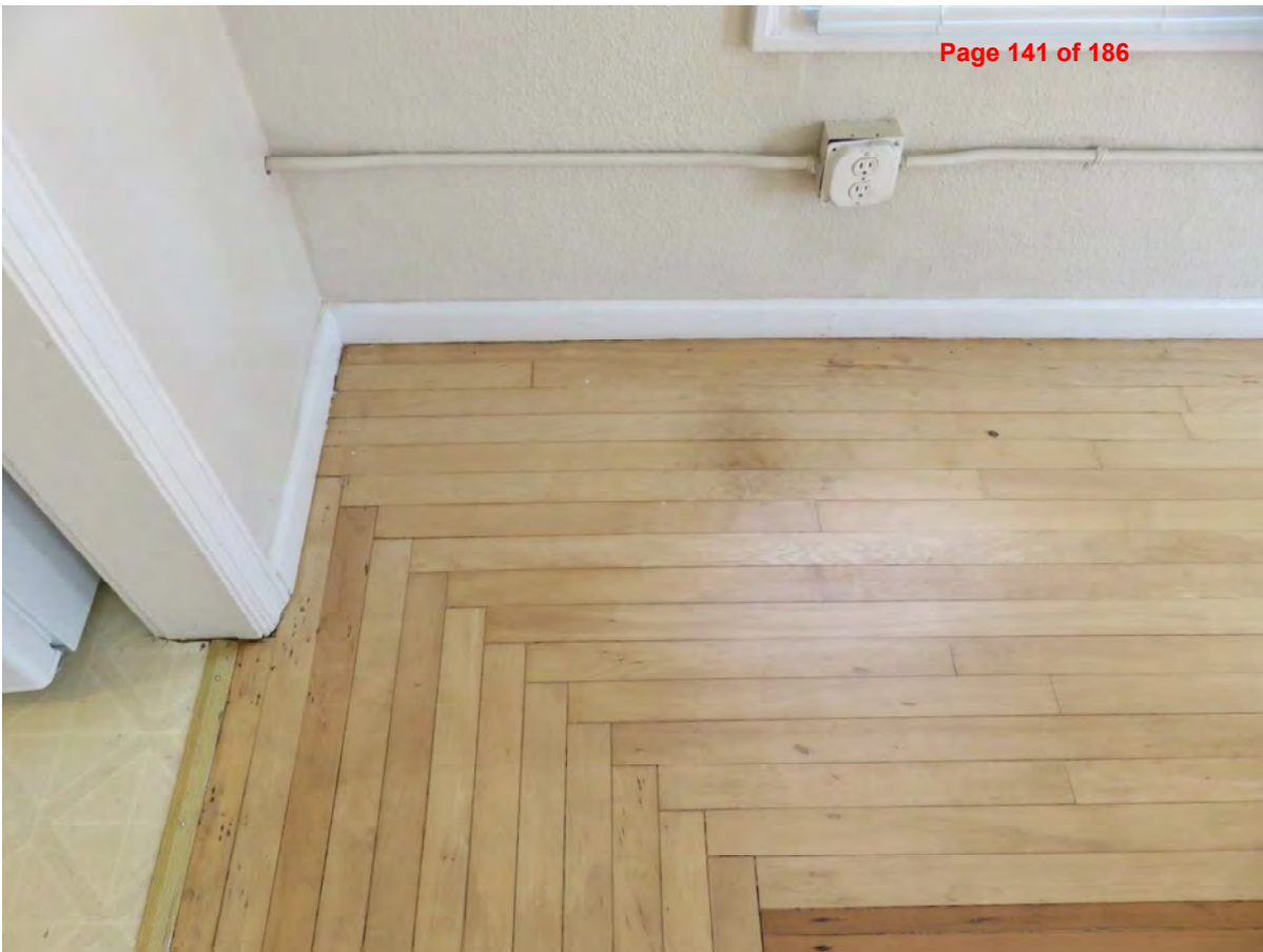
Fig. 45. Newton Apartments, detail of original oak/fir floors, Unit 17, looking northwest, 2018. Source: Owner.
