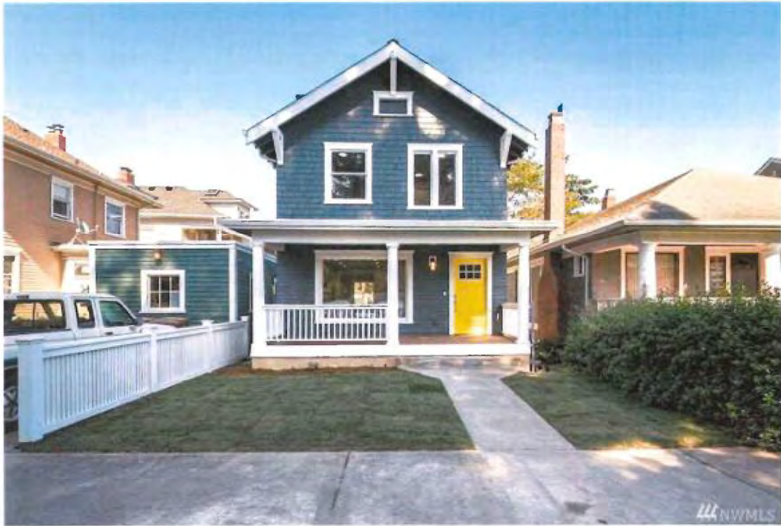
After Exterior Pictures
