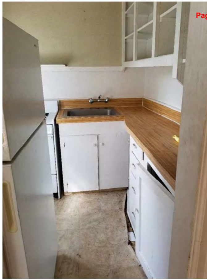
Fig. 43. Newton Apartments, kitchen prior to rehabilitation, Unit 12, looking west, 2018. Source: Owner.
