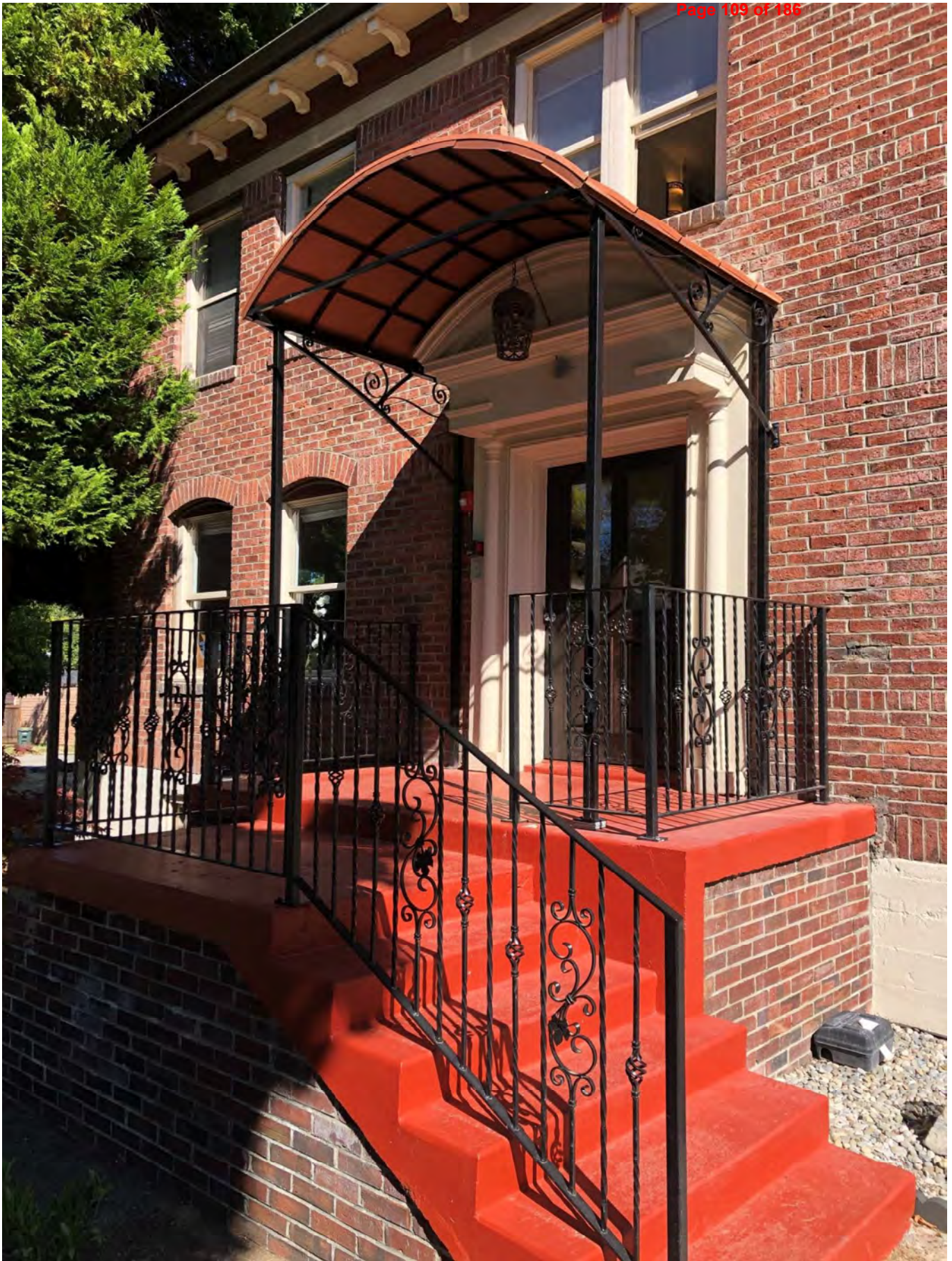
Fig. 22 (After). Newton Apartments front porch, looking northeast, with new awning and support. August 2020. Source: Stephen Day Architecture.
