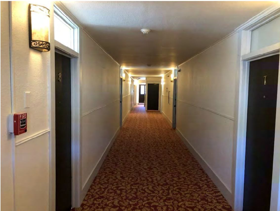
Fig. 28 (After). Newton Apartments, First Floor corridor, looking west to entry, door to Basement stair. August 2020. Source: Stephen Day Architecture.
