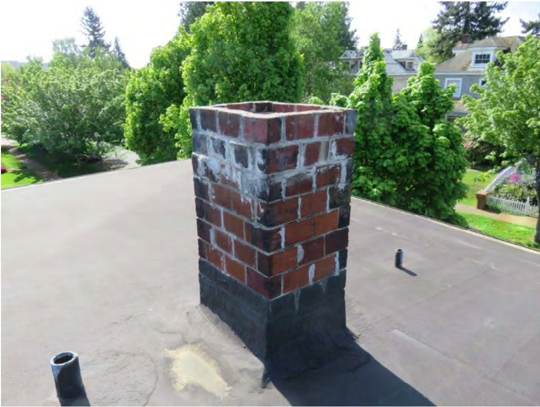
Fig. 24. Newton Apartments roof at southeast corner, looking southeast, 2018. Source: Owner.
