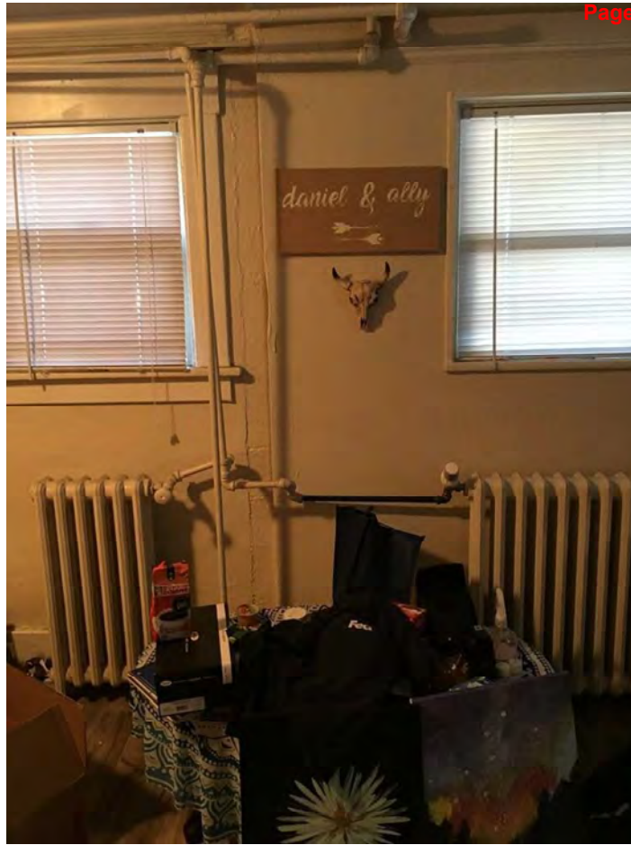
Fig. 34B. Newton Apartments, Basement Unit 18, looking west, 2018. Source: Owner.
