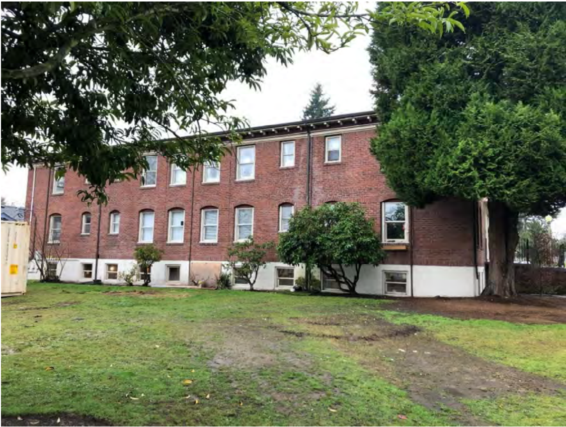
Fig. 12. Newton Apartments, north façade, looking south. December 2019. Source: Stephen Day Architecture.
