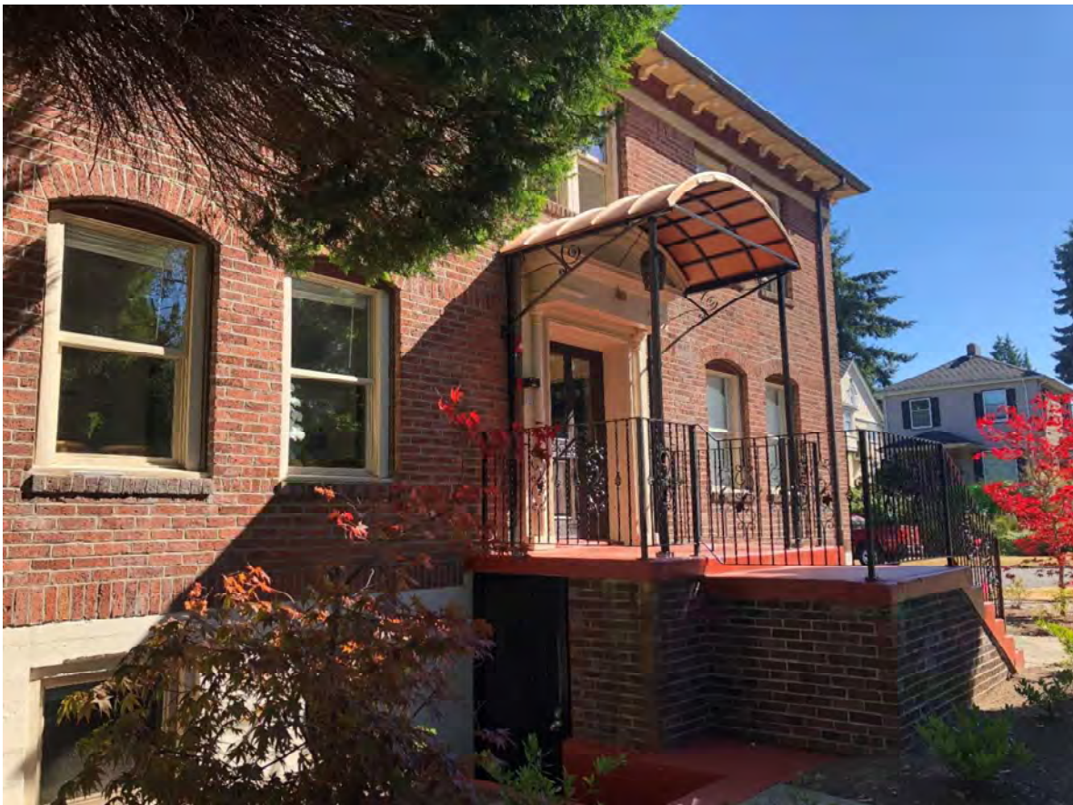
Fig. 14 (After). Newton Apartments, east facade, looking southeast. August 2020. Source: Stephen Day Architecture.
