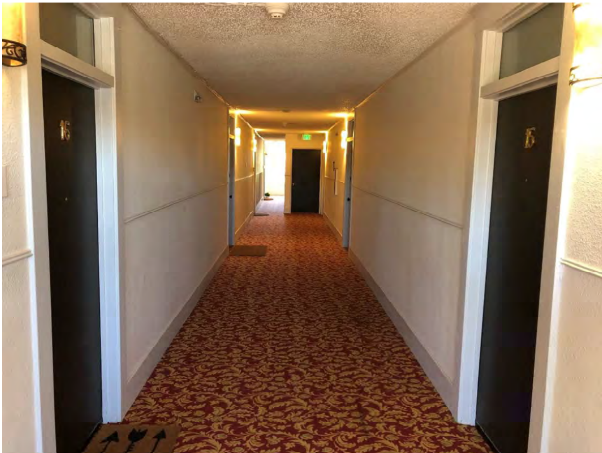
Fig. 29 (After). Newton Apartments, Second Floor corridor, looking west toward door to stair. August 2020. Source: Stephen Day Architecture.
