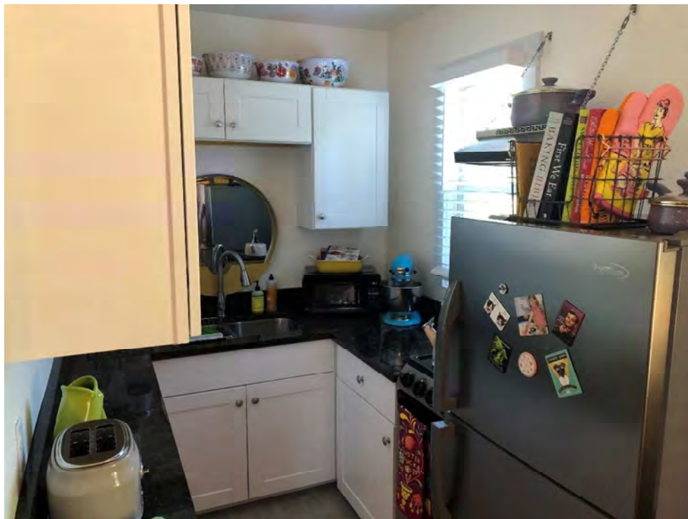
Fig. 38 (After). Newton Apartments, kitchen after rehabilitation, former Unit 7, looking west. August 2020. Source: Stephen Day Architecture.
