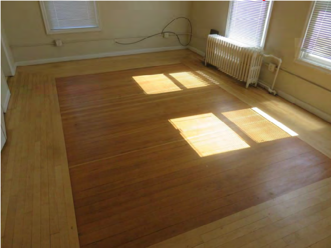
Fig. 46. Newton Apartments, original oak/fir floors, Unit 17, looking northeast 2018. Source: Owner.
