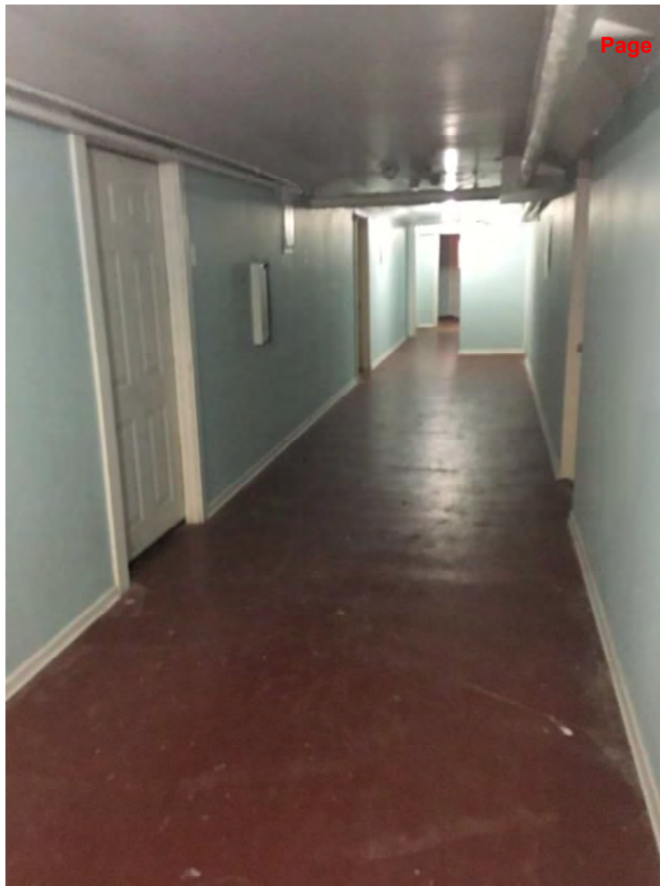
Fig. 27. Newton Apartments, Basement corridor, looking west toward enclosed stair, 2018. Source: Owner.
