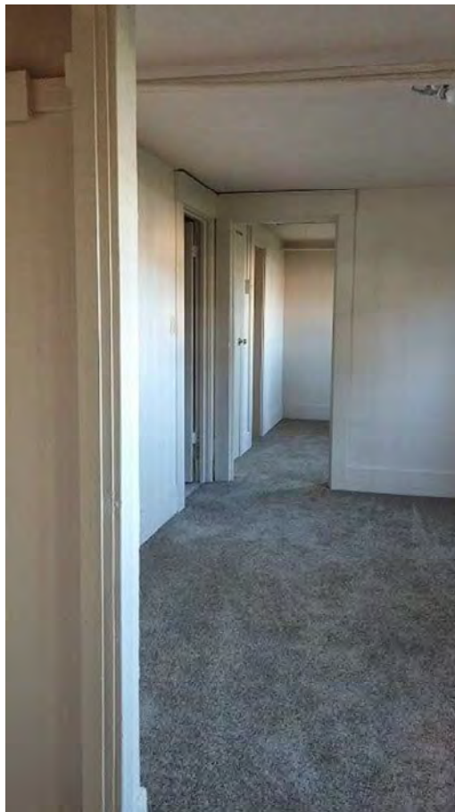
Fig. 35A. Newton Apartments, Basement Unit 20, looking west to middle room, 2018. Source: Owner.
