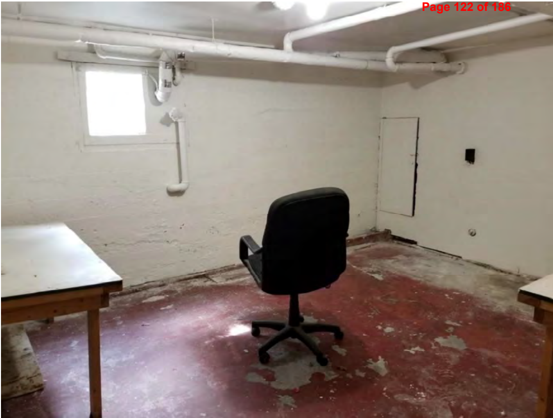
Fig. 33. Newton Apartments, Basement storage/laundry area, looking south, 2018. Source: Owner.
