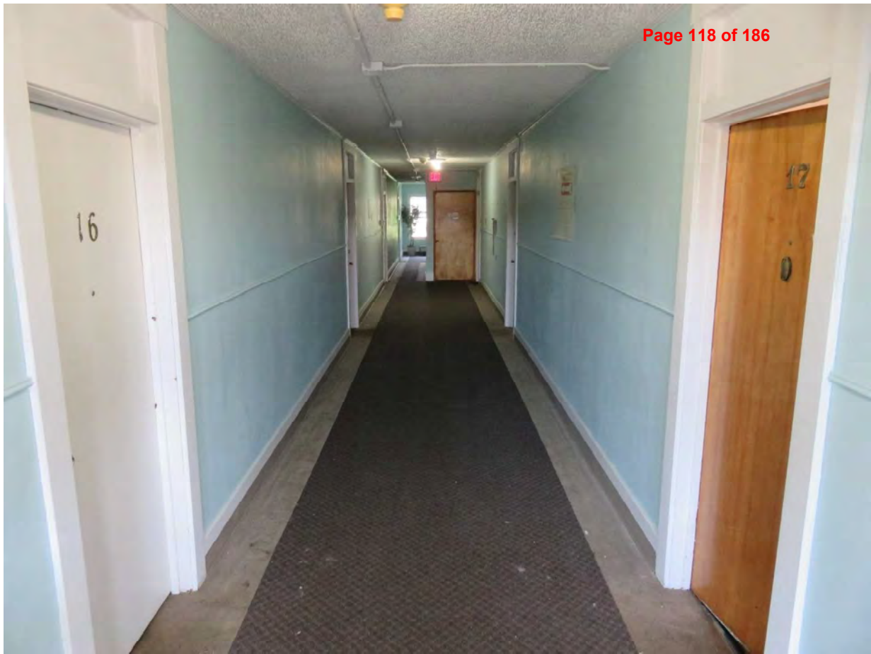
Fig. 29. Newton Apartments, Second Floor corridor, looking west toward door to stair, 2018. Source: Owner.
