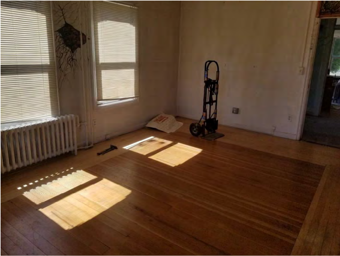
Fig. 41. Newton Apartments, original oak/fir floors, Unit 7, looking southeast, 2018. Source: Owner.
