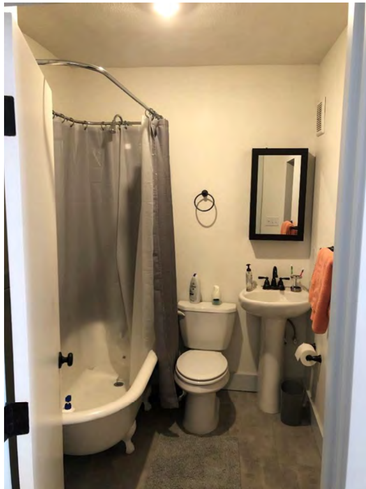
Fig. 40 (After). Newton Apartments, typical bathroom after rehabilitation, former Unit 6, looking northeast. August 2020. Source: Stephen Day Architecture.
