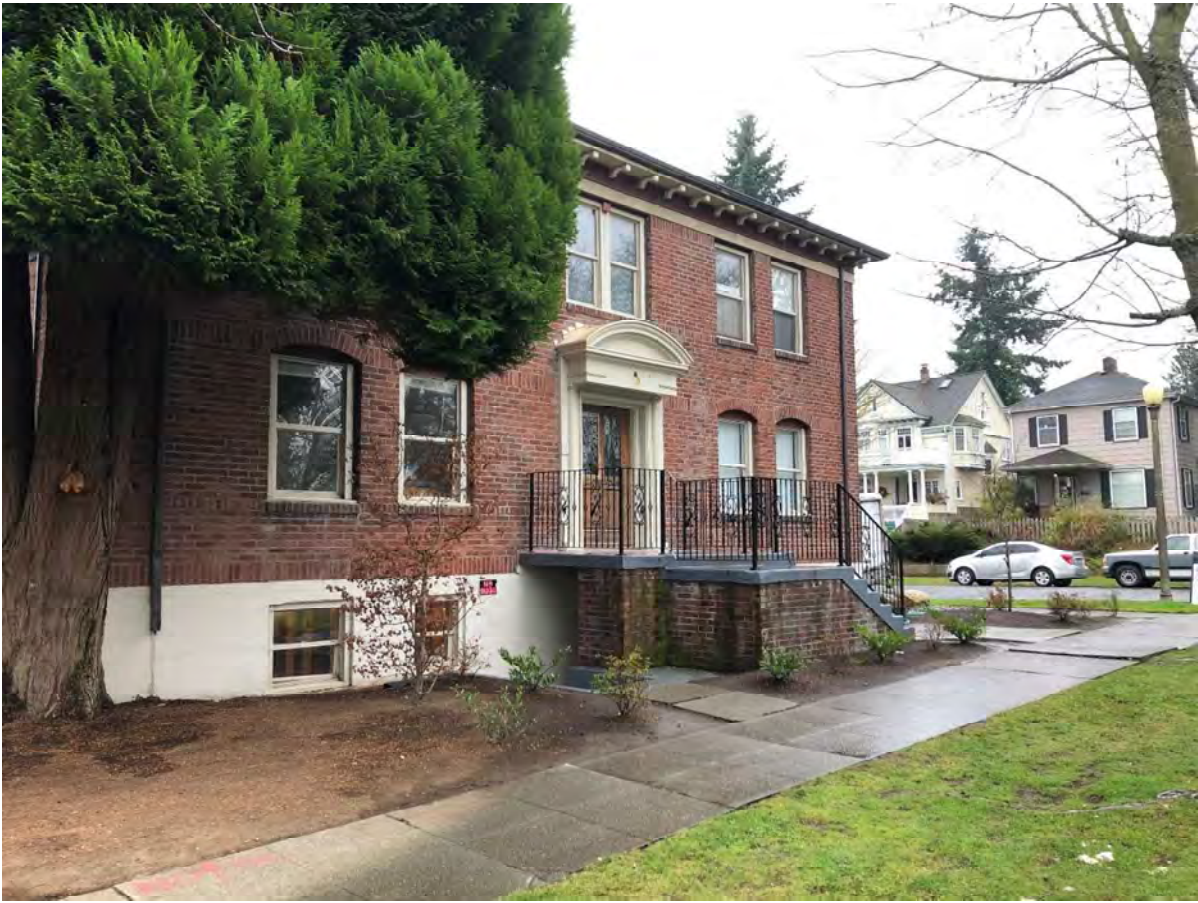
Fig. 14. Newton Apartments, east facade, looking southeast. December 2019. Source: Stephen Day Architecture.
