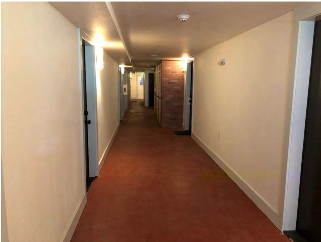
Fig. 27 (After). Newton Apartments, Basement corridor, looking west toward enclosed stair, August 2020. Source: Stephen Day Architecture.
