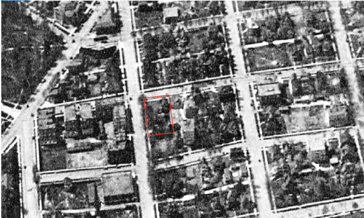
Figure 4. 1920 aerial photo, Detail with 205 N. Yakima in red. (General Photo. Coll., BAC-002, Tacoma Public Library)
