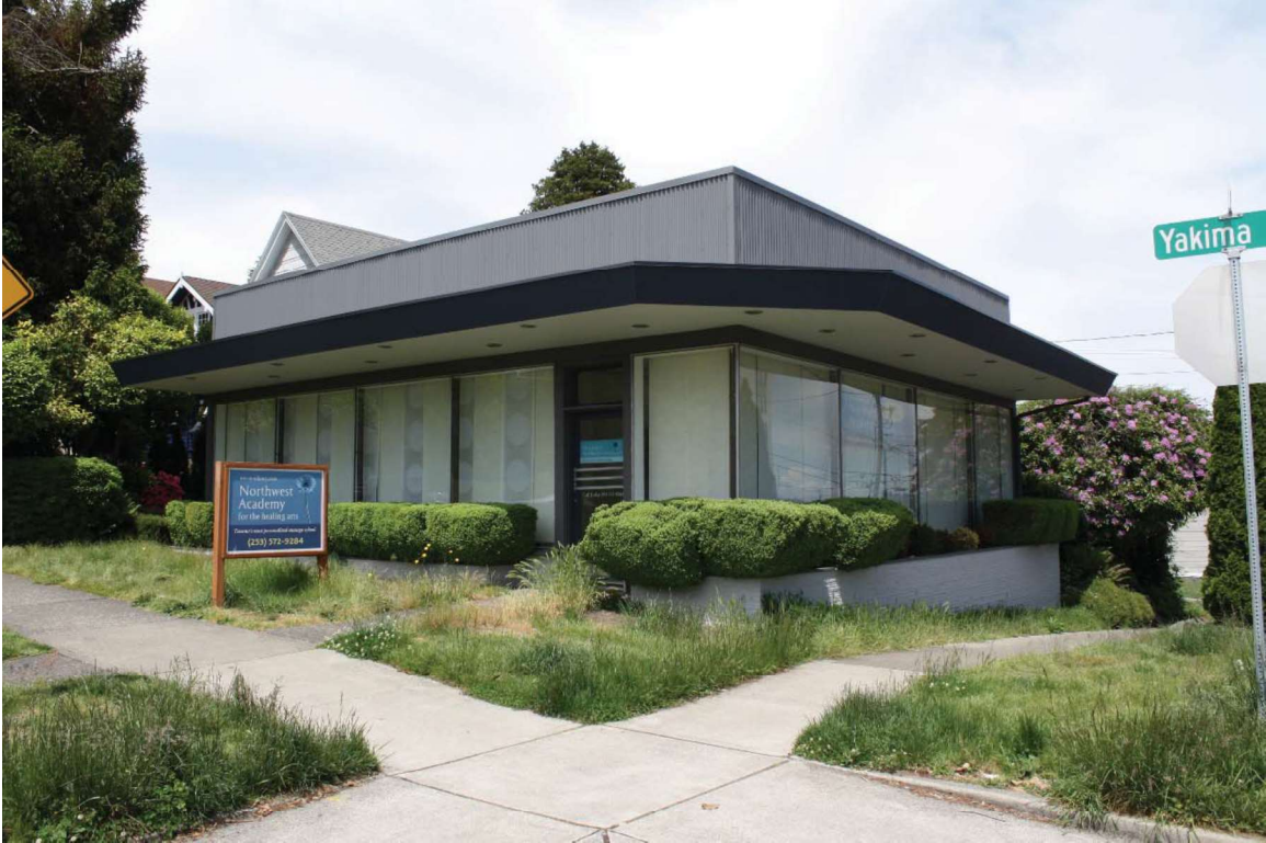
Figure 12. Overview of 201 N. Yakima Avenue, view northwest
