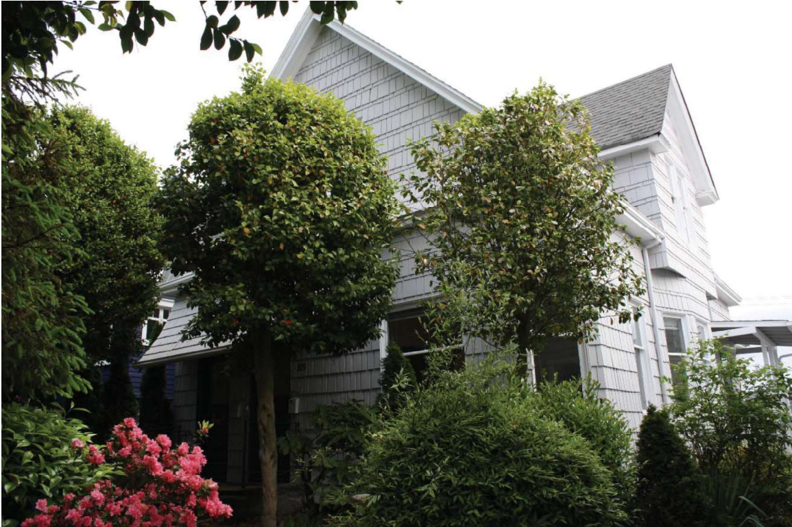
Figure 17. Primary (south) and east elevations of 205 N. Yakima Avenue, view north
