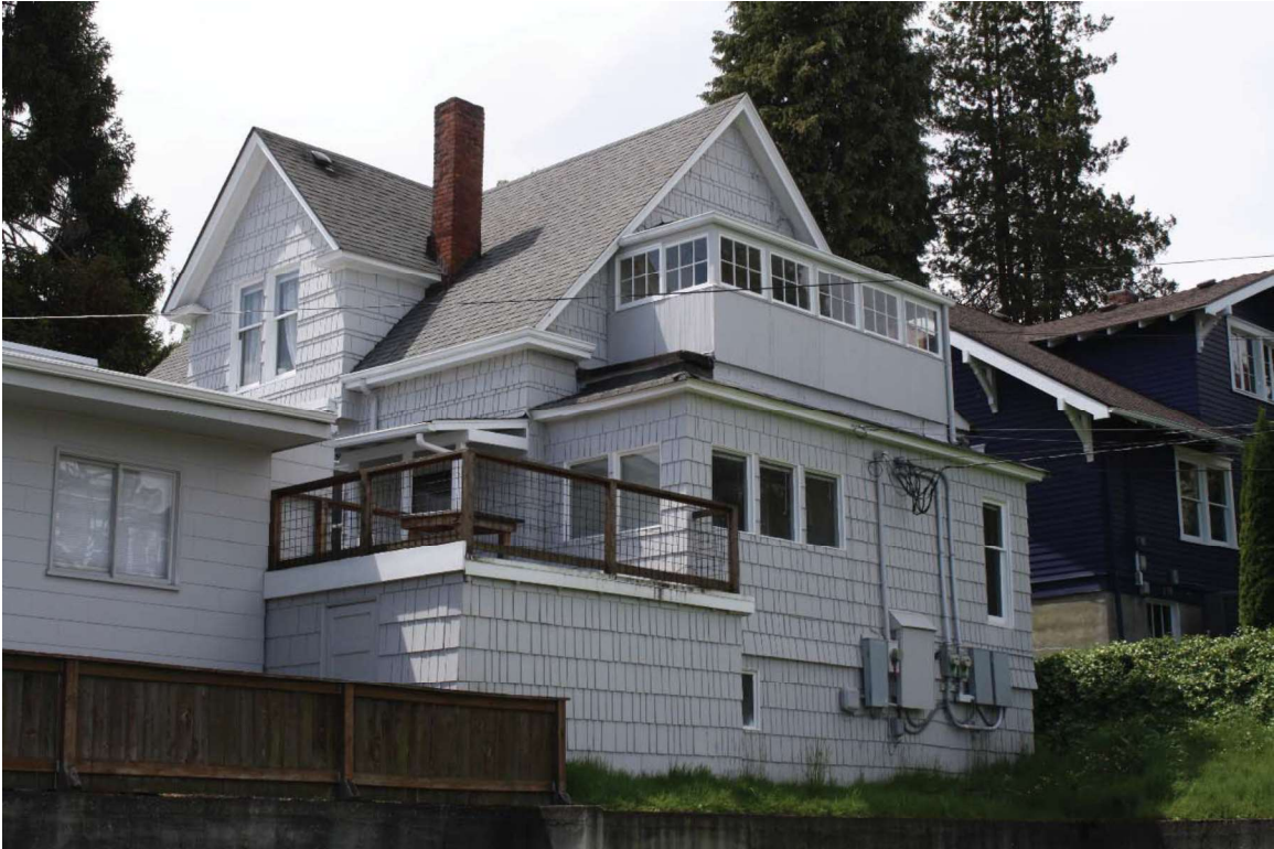
Figure 19. East and north elevations of 205 N. Yakima Avenue, view to west
