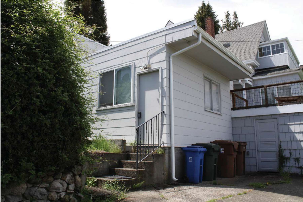
Figure 15. Rear addition of 201 N. Yakima Avenue, view west
