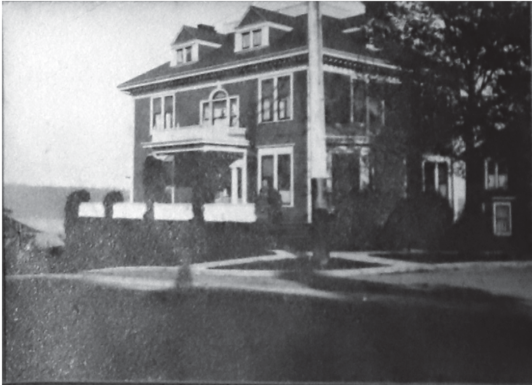
Figure 5. Undated historic photo of building's southwest corner.
