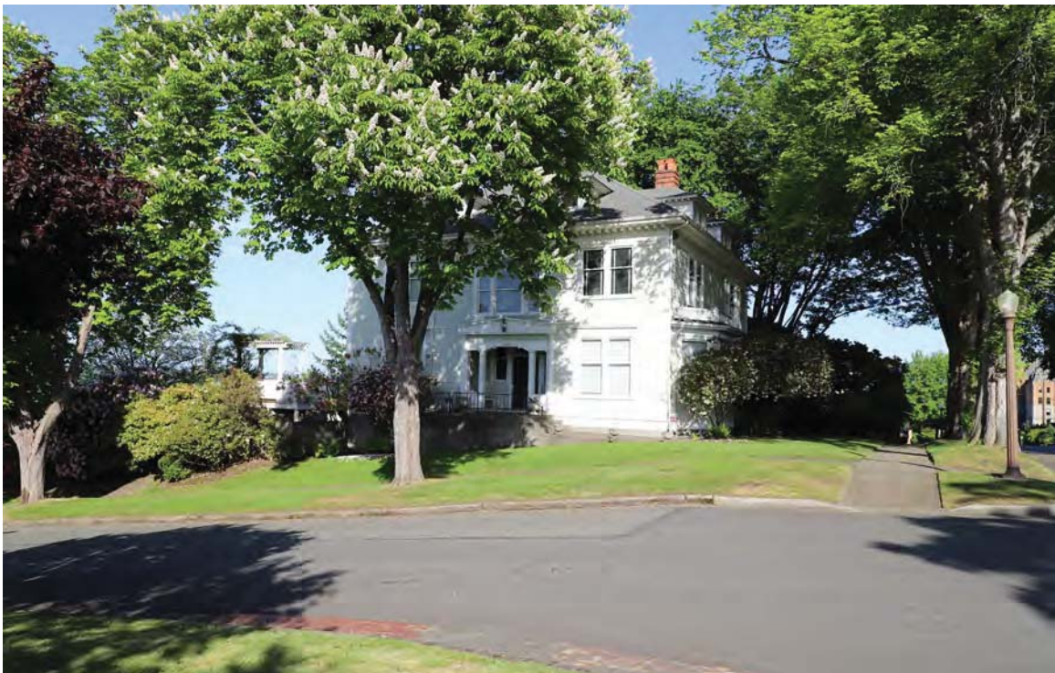
Figure 20. West and south elevations, 2019.
