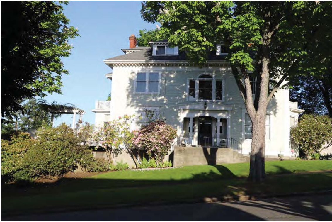
Figure 19. West (main) elevation, 2019.
