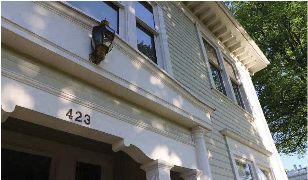
Figure 25. Main entry details, 2019.
