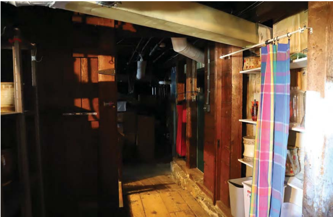
Figure 46. Basement view looking south, 2019.
