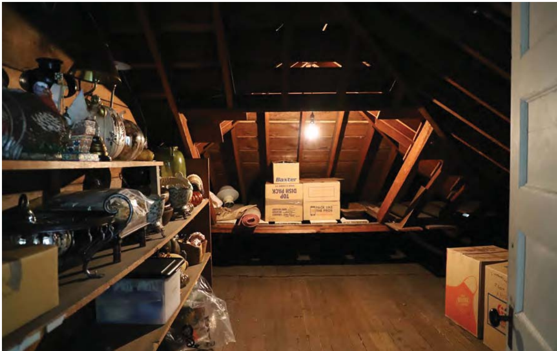
Figure 44. Unfinished attic space, 2019.
