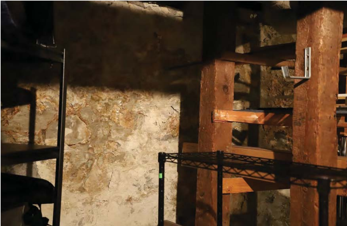
Figure 45. Basement view with stone foundation and timber support posts, 2019.
