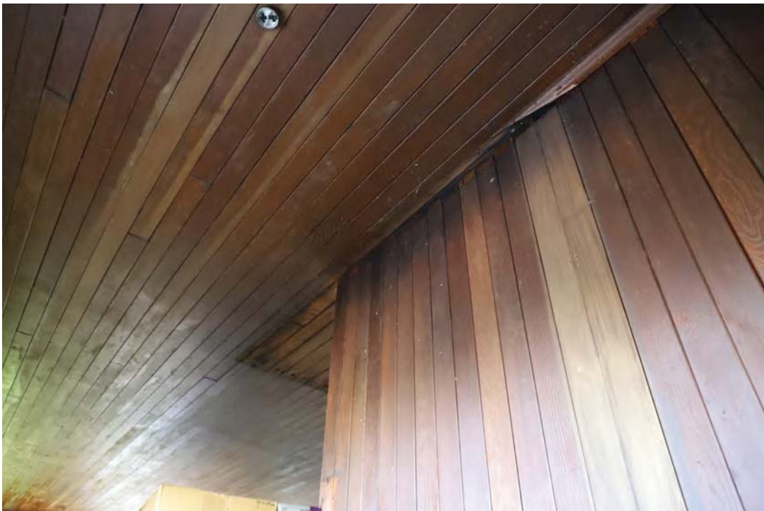
Figure 48. Garage interior finishes detail, 2019.
