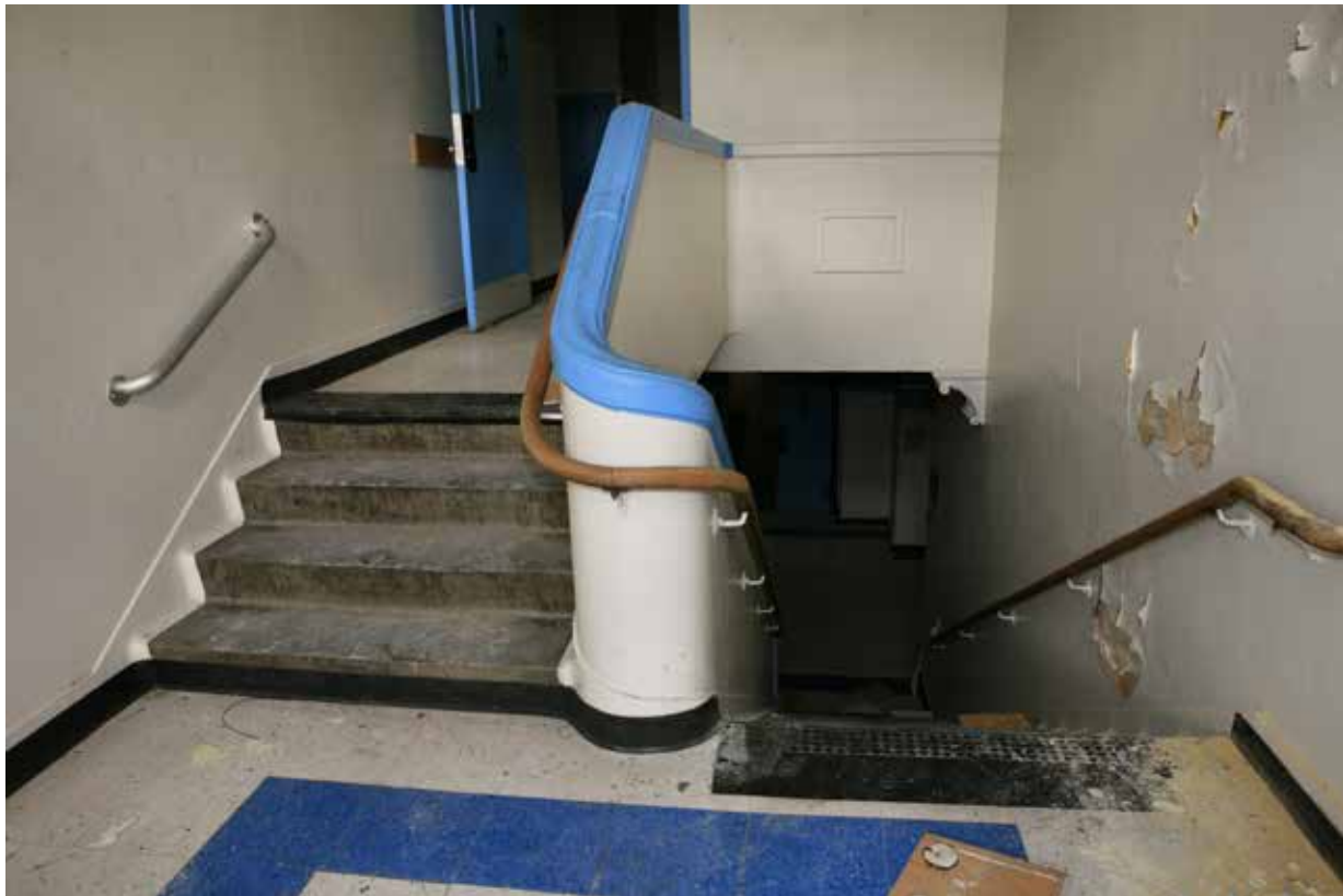
CP56. SE stairwell, landing between 1st and 2nd floors. Looking north.
