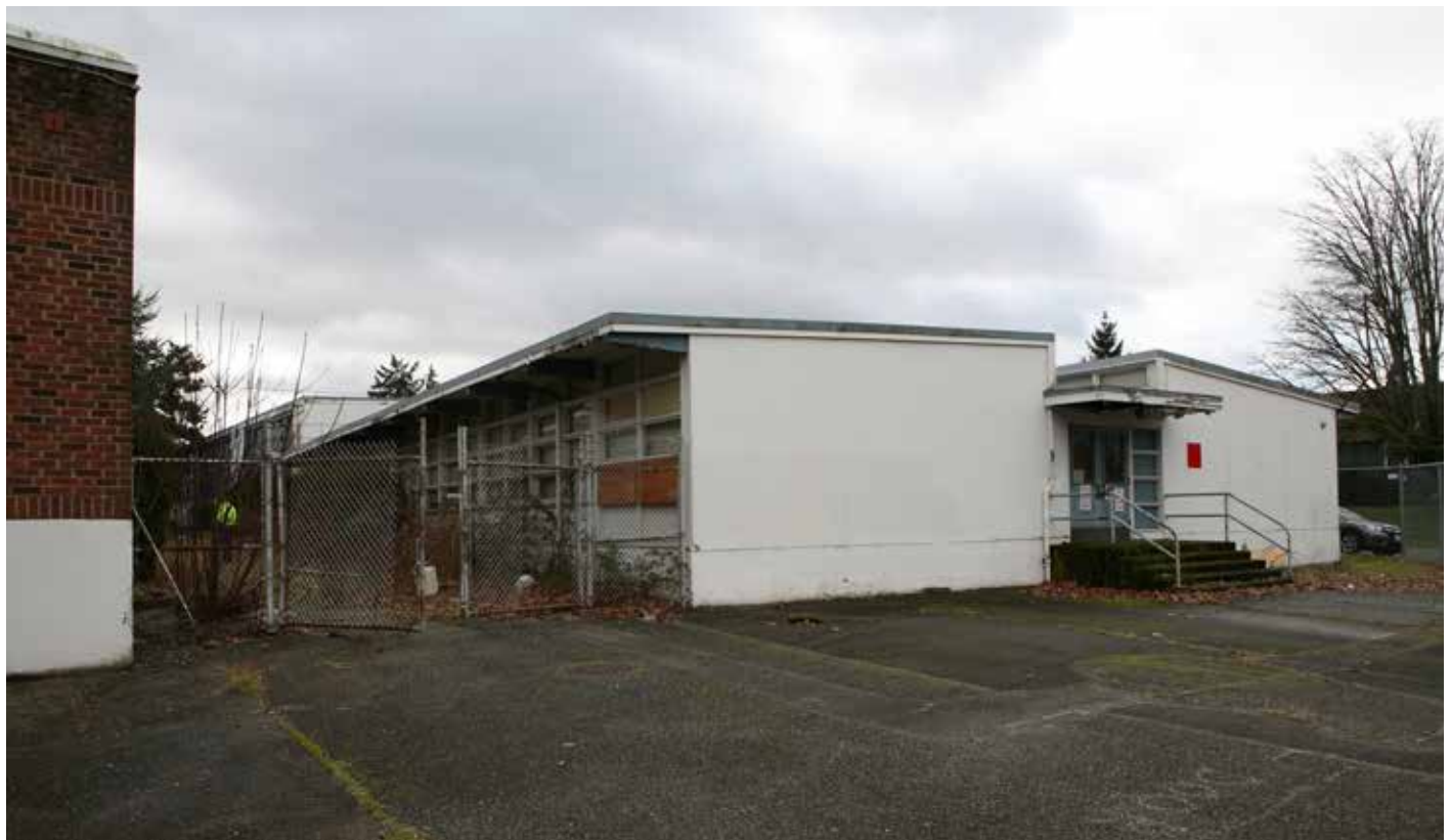
CP6. NE corner of '53 north annex, looking SW.
