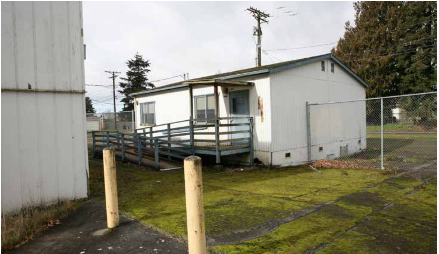
CP24. SE corner of detached (1990) portable classroom, looking NW at north edge of parcel.
