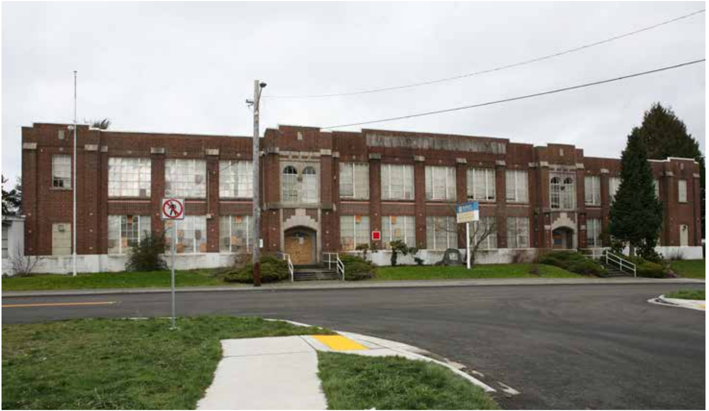
CP1. South facade of original building (1926) with divided main entries.
