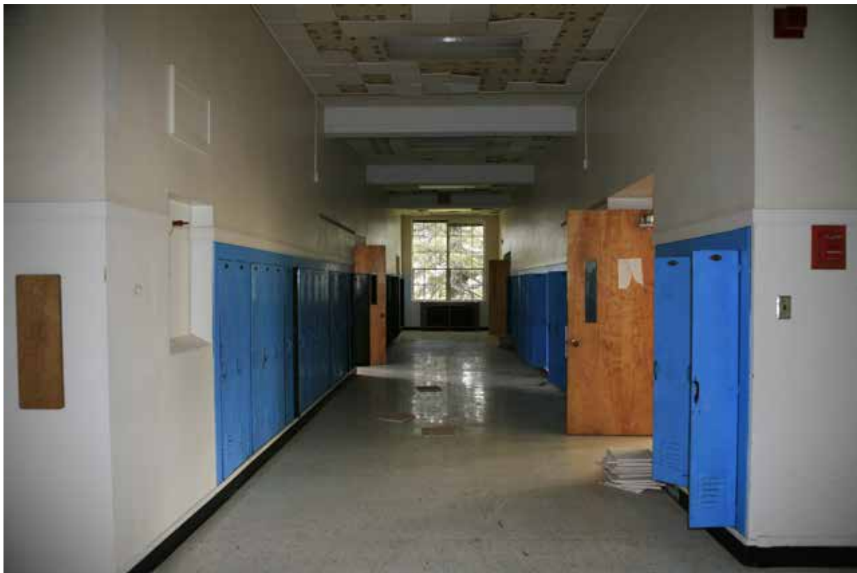
CP58. 2nd floor, main corridor looking east.
