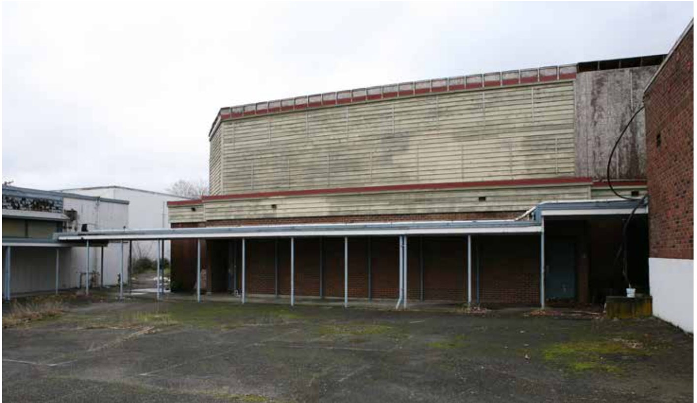
CP13. West facade of pool addition. Looking east.
