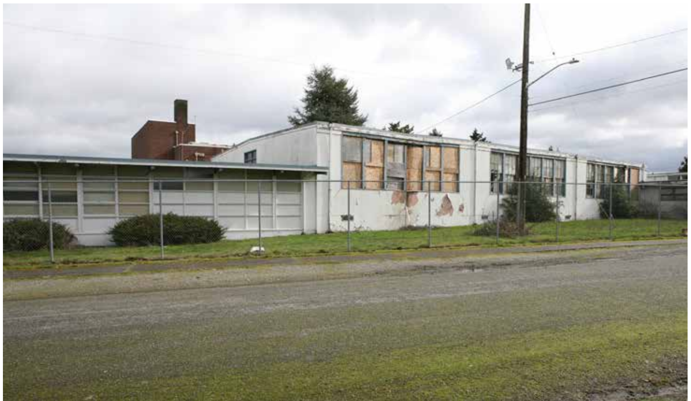
CP5. West facade, partial. '53 north annex (L), '43 annex (center).
