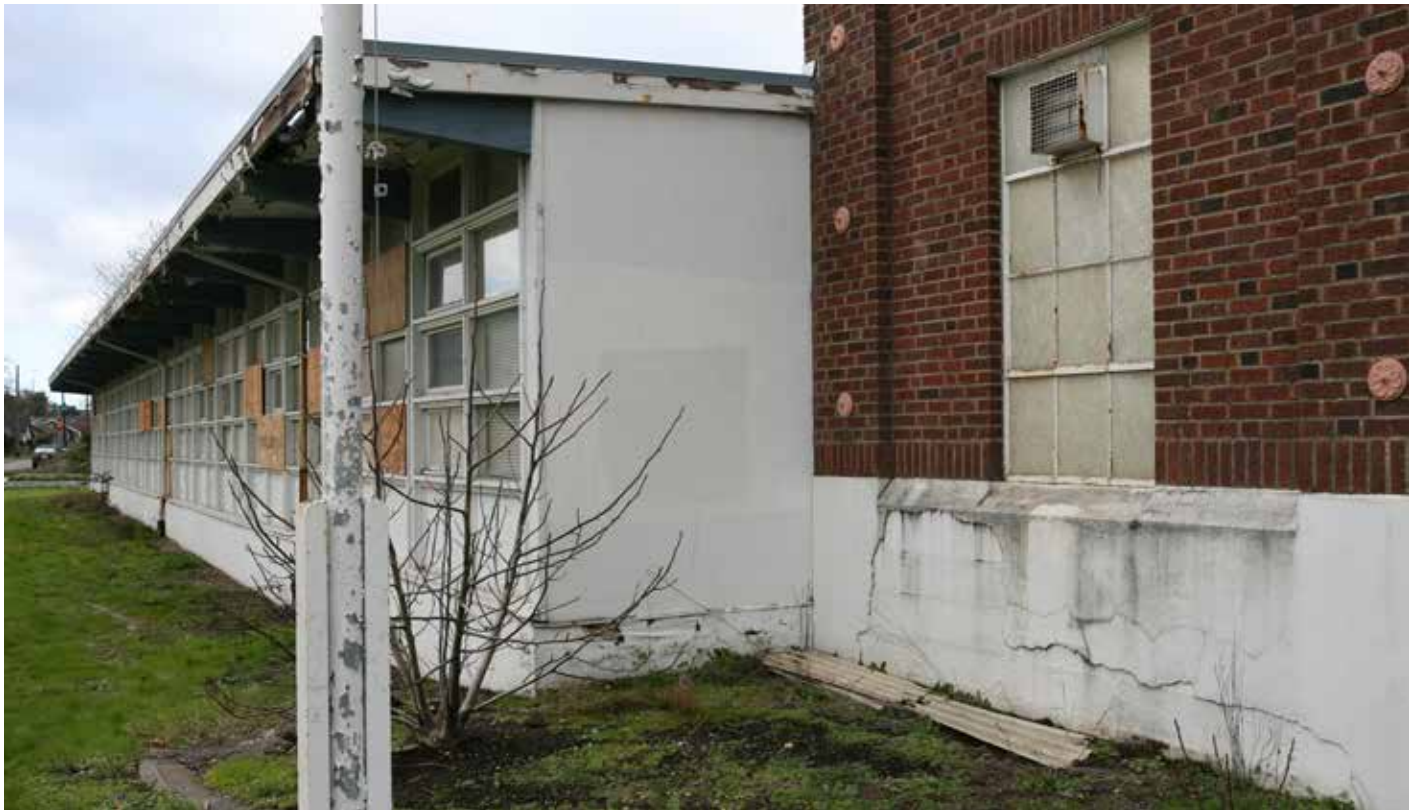
CP29. Detail, south facade. Looking NW.
