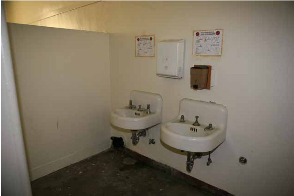
CP47. Restroom, first floor.
