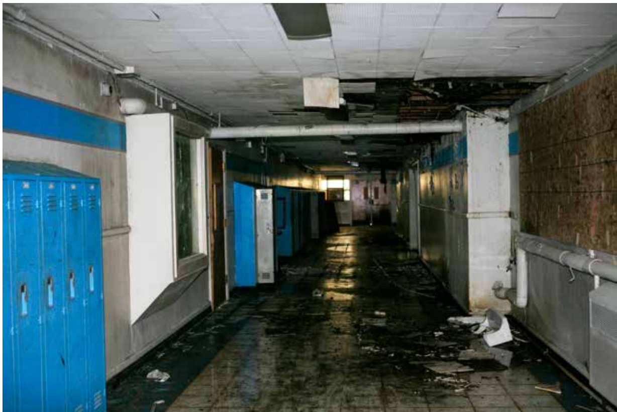
CP48. Looking west from original building into south 1953 annex.
