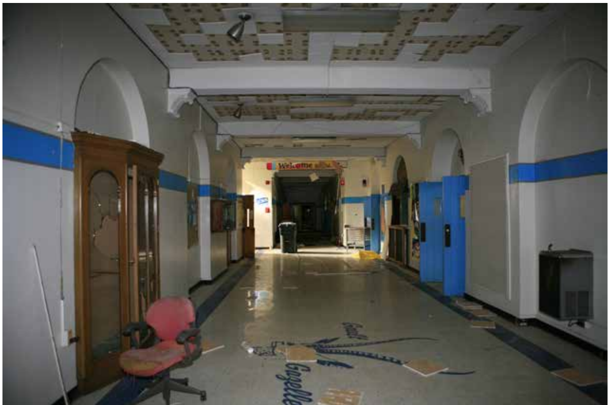
CP40. 1st floor main corridor, looking west. Auditorium is through doors to the right (north wall).
