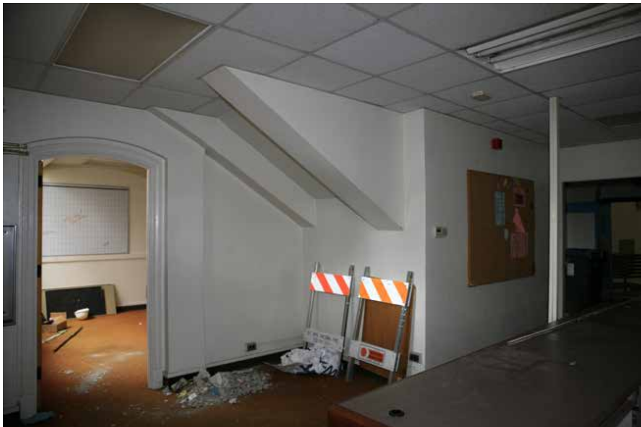
CP30. Looking NW from inside the westernmost main/south entry.
