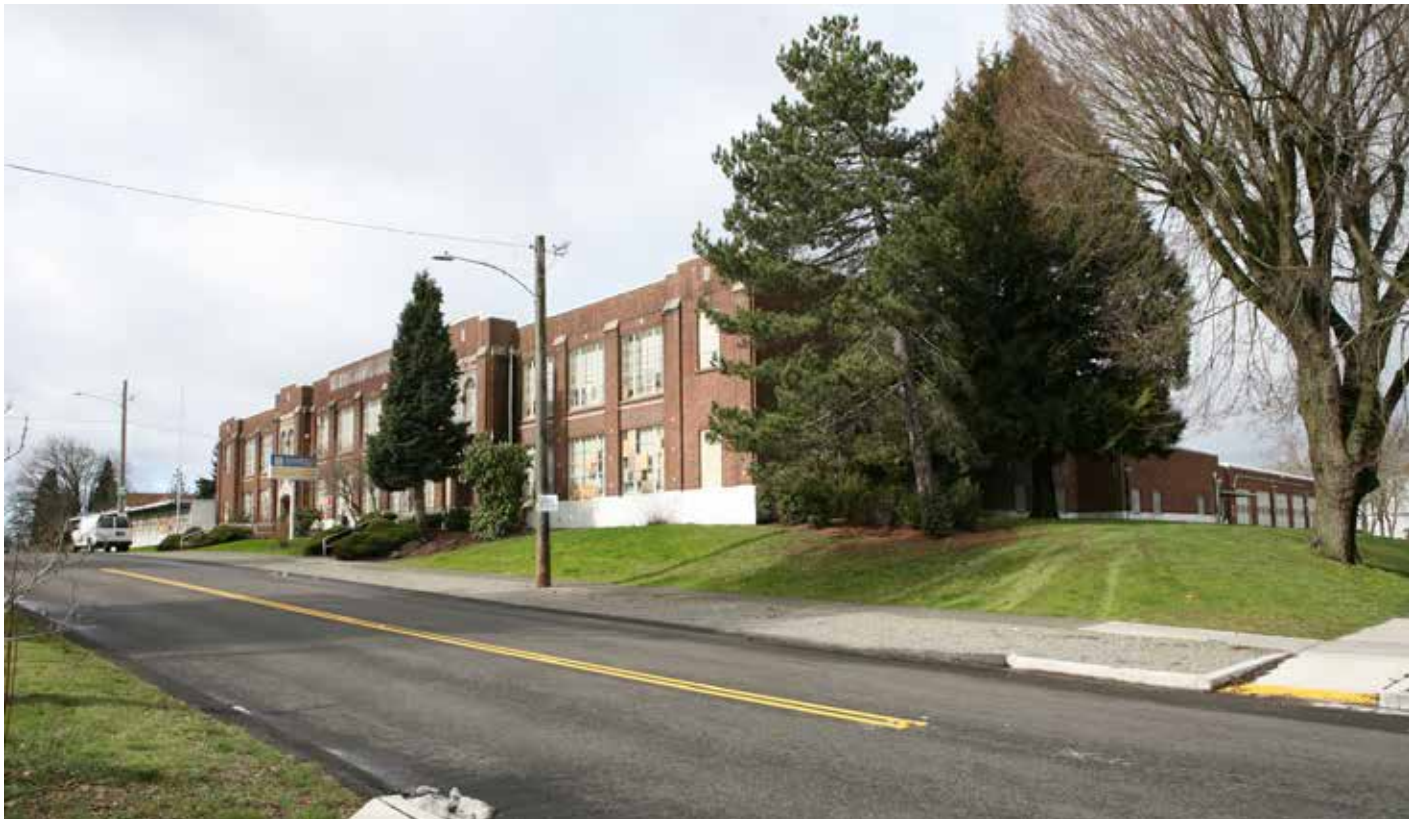
CP22. Southeast corner.
