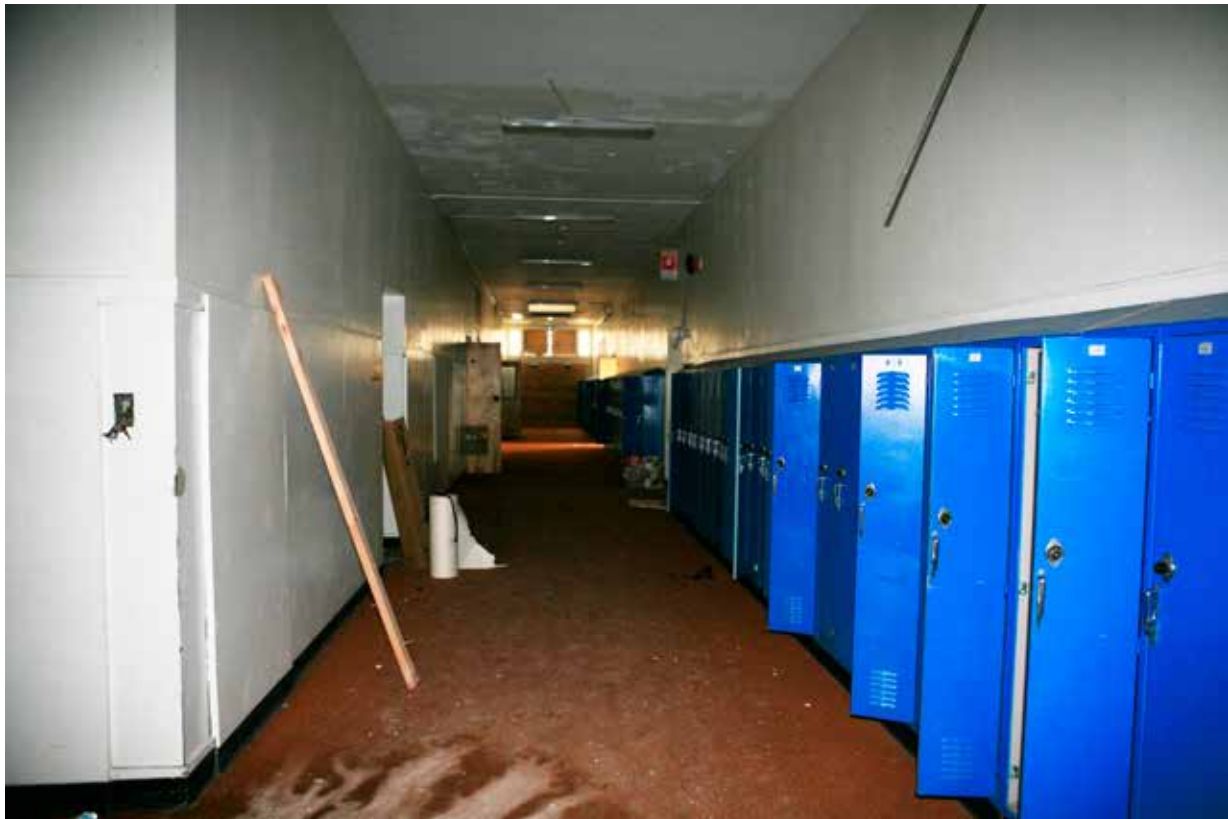
CP50. 1st floor, east corridor looking north.
