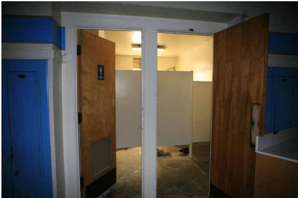
CP46. Restroom, first floor.
