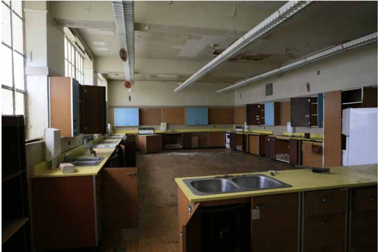
CP51. 1st floor. Cooking Room (Rm 106), looking south.
