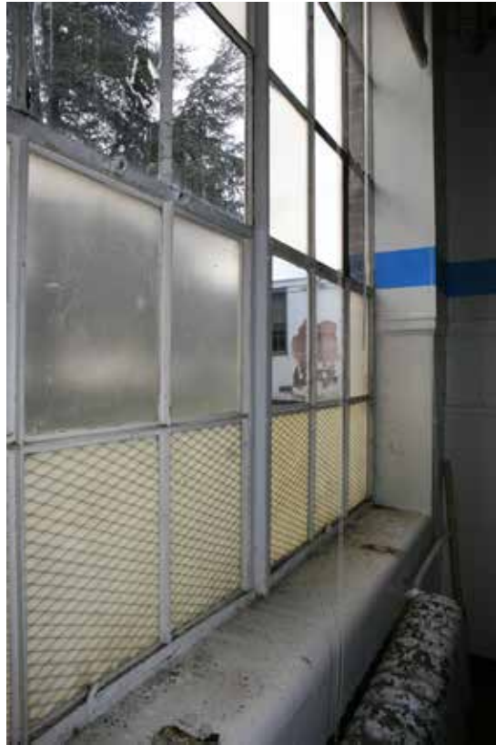
CP55. 1st floor, typical window. West side corridor.
