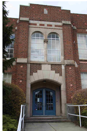
South Door Detail I
