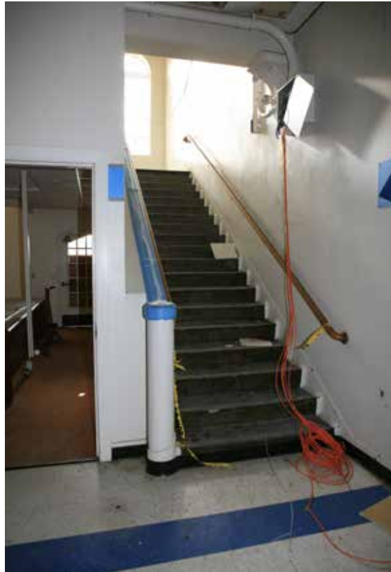
CP49. 1st floor, main corridor, looking S at SW stairwell. (Reflective twin of SE stairwell, previously shown.)
