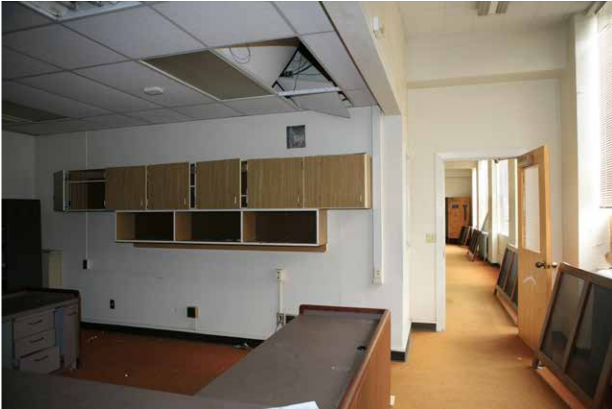
CP31. Looking east from inside the westernmost main/south entry.
