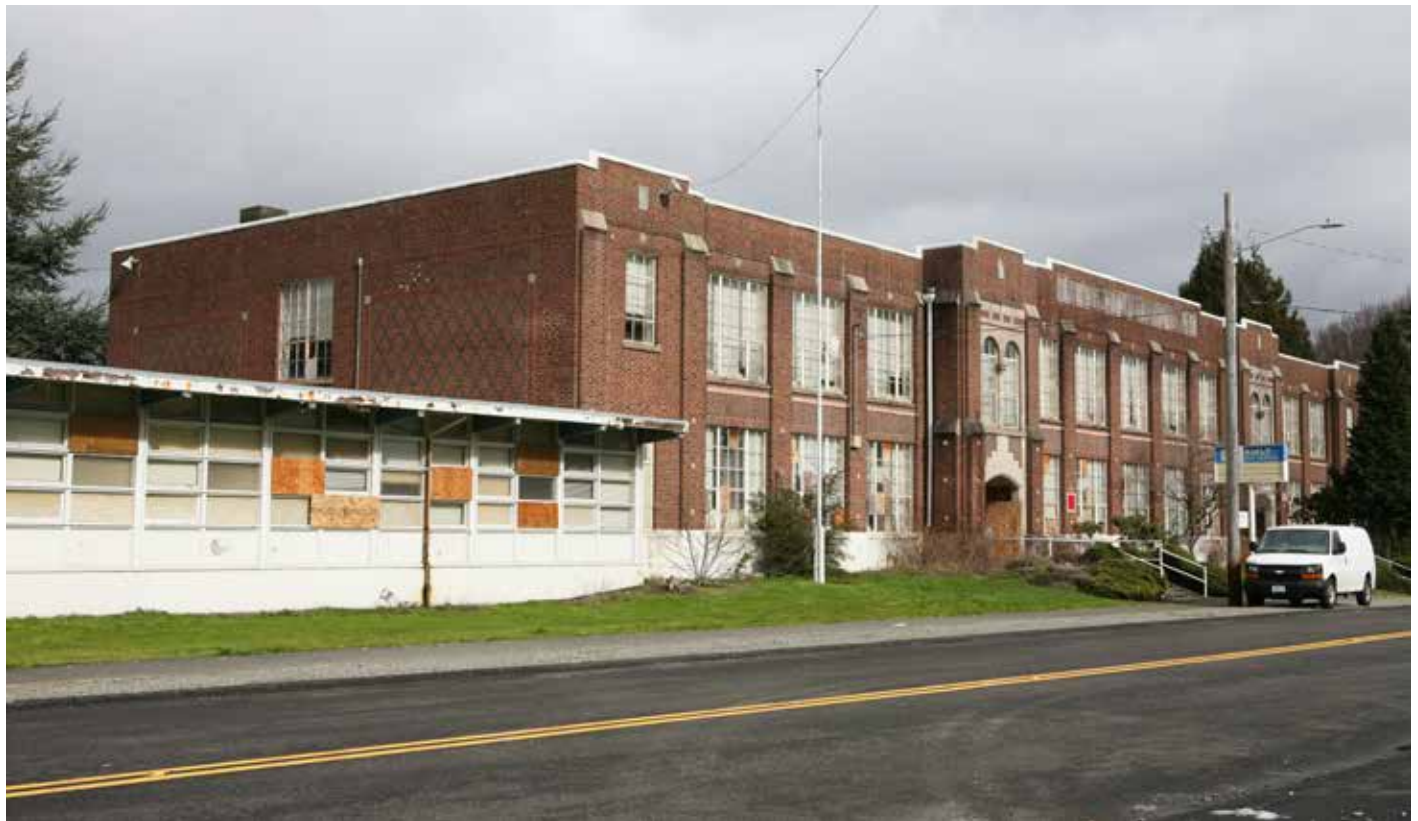
CP3. Southwest corner of original (1926) building with '53 south annex at left.
