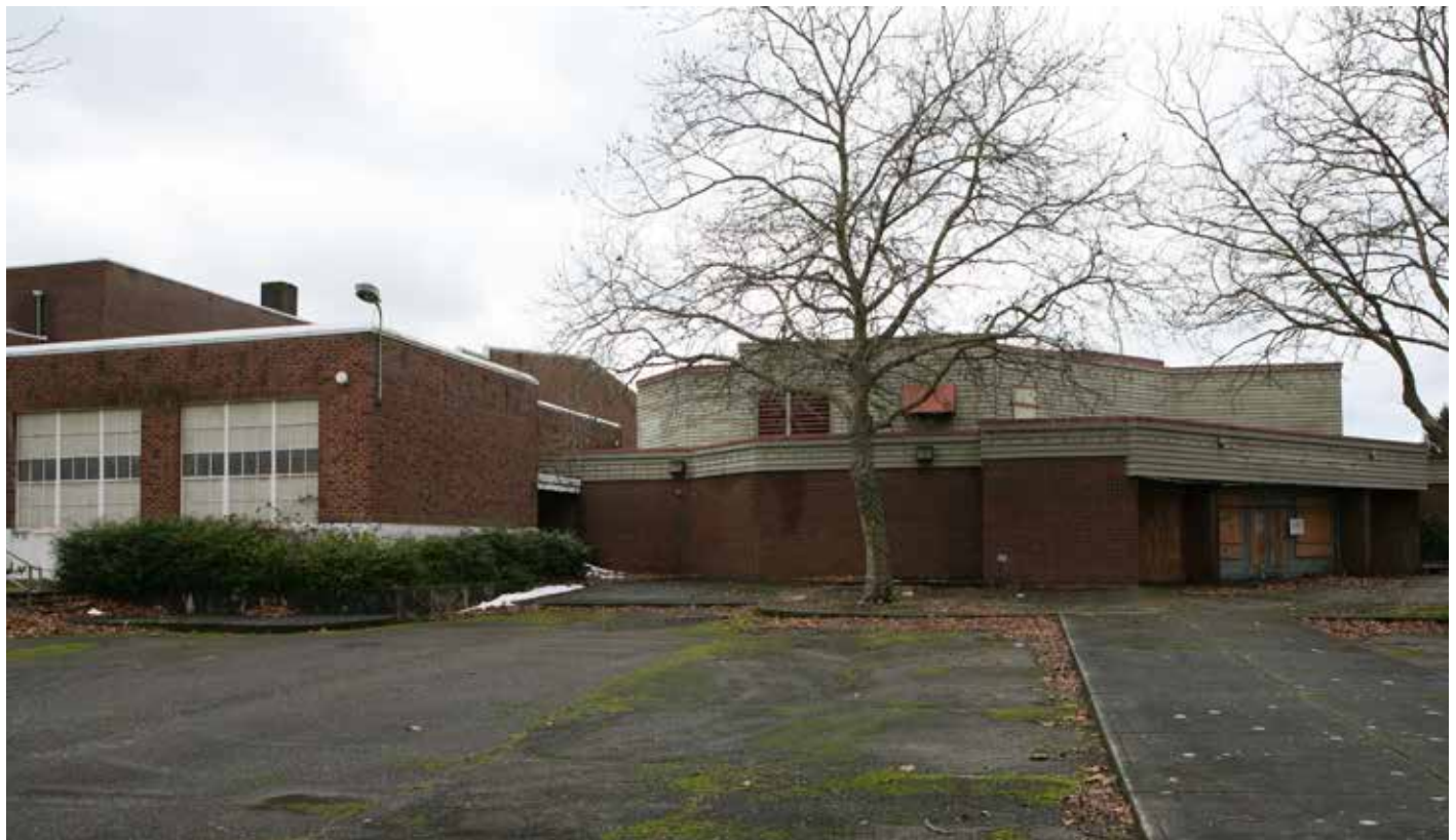
CP18. Looking west at junction between original building (L) & 1986 pool addition (R).
