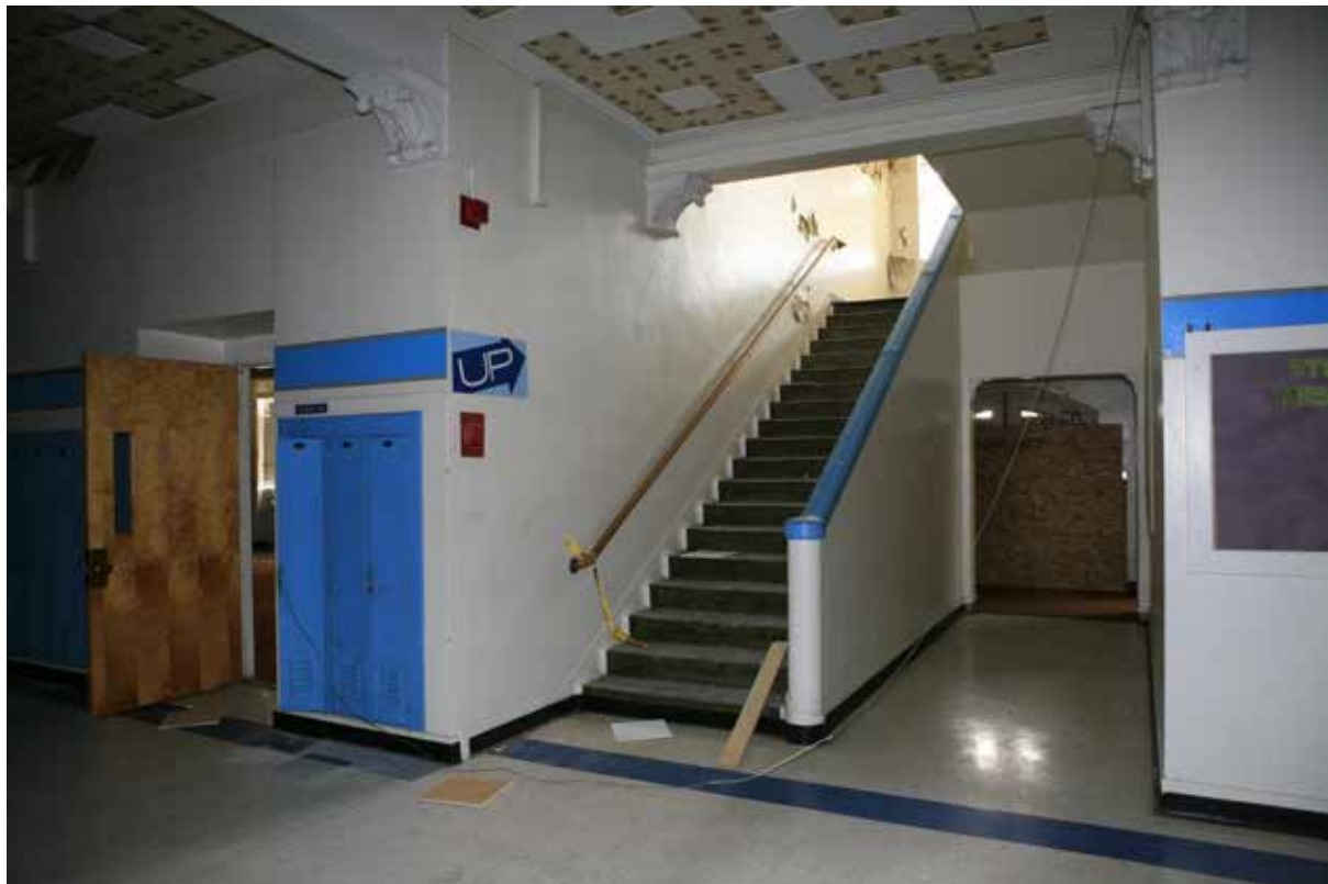
CP42. 1st floor, main corridor, looking SE at Classroom 104 and SE stairwell.
