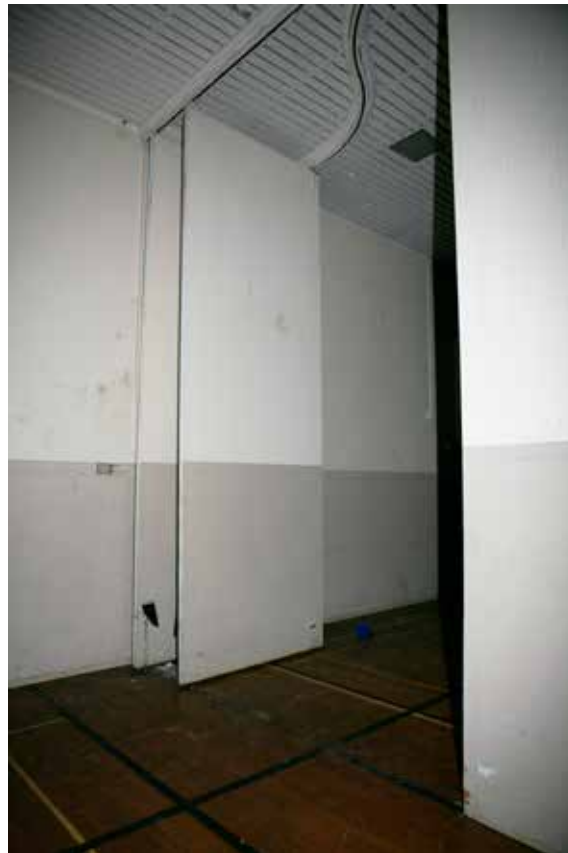
CP54. 1st floor. Former gymnasium, wooden panels dividing boys side from girls side. Note overhead track. Looking SW.
