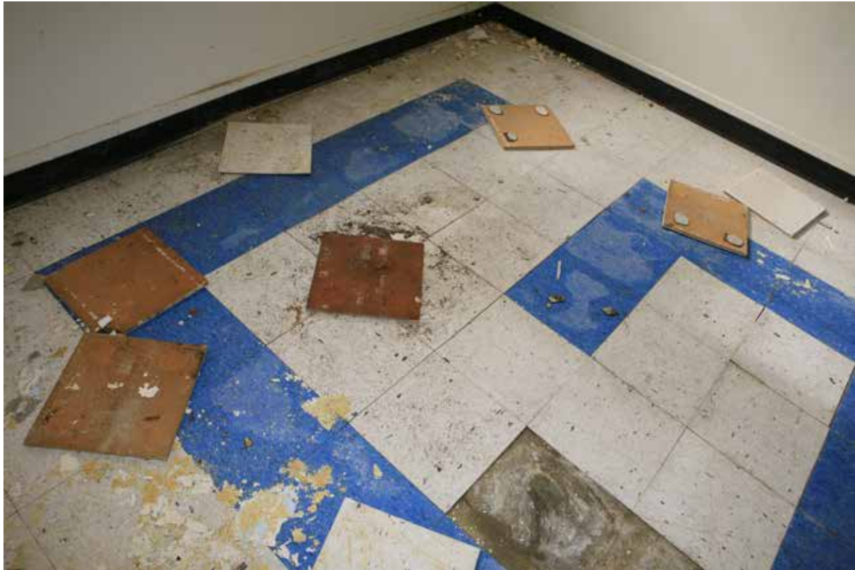
CP57. SE stairwell, landing between 1st and 2nd floors. Looking SW.
