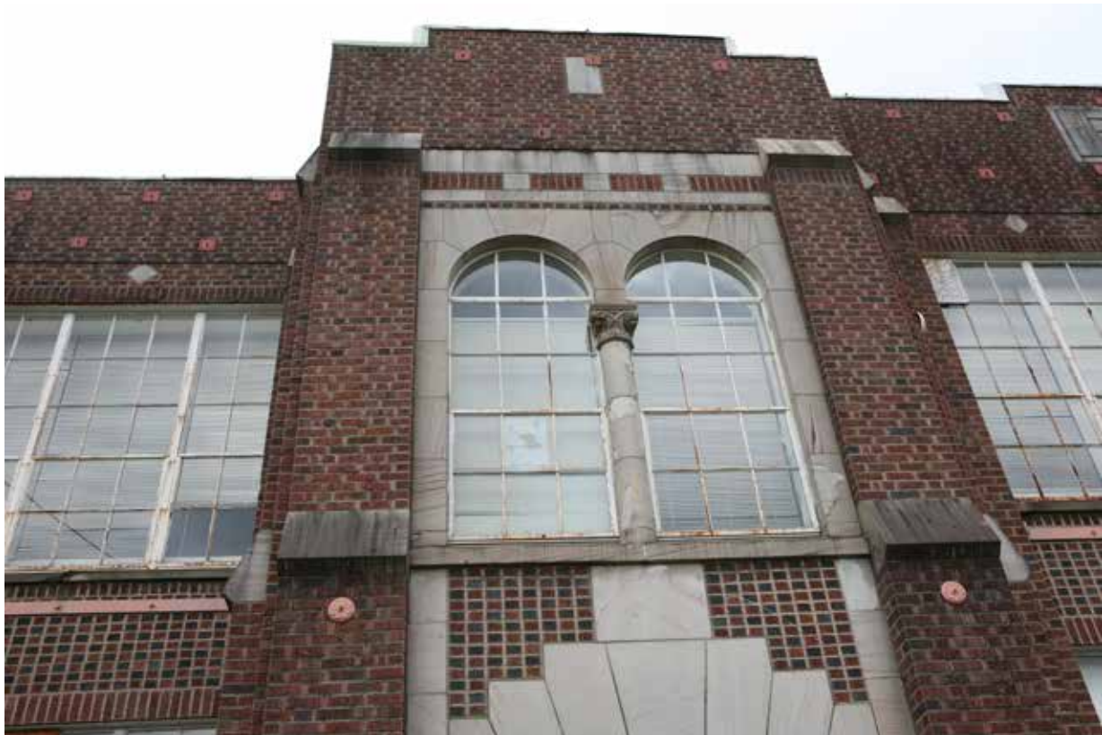
CP26. Detail, south facade, above westernmost entry.
