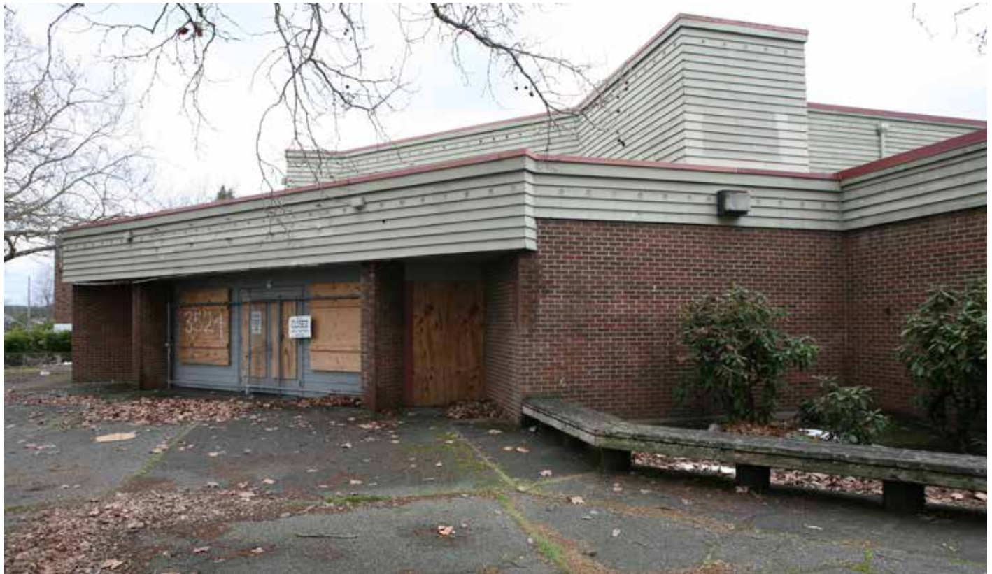
CP17. NE corner and main exterior entry to pool addition. Looking south.
