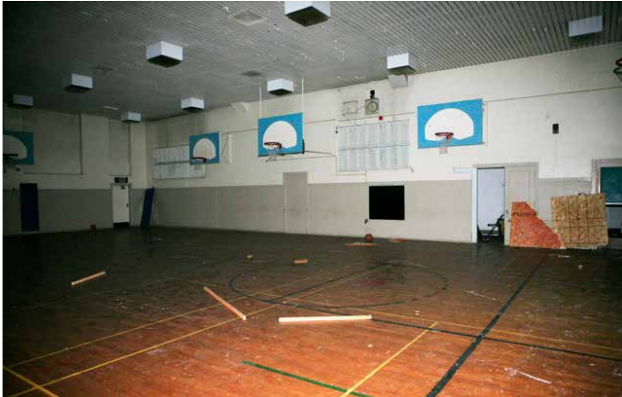
CP53. 1st floor. Former gymnasium, looking NE.
