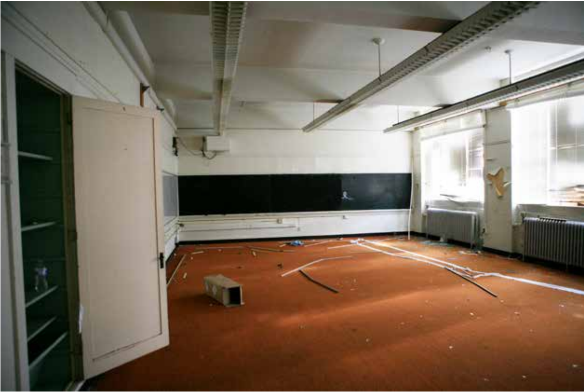
CP43. Typical classroom (Room 104).
