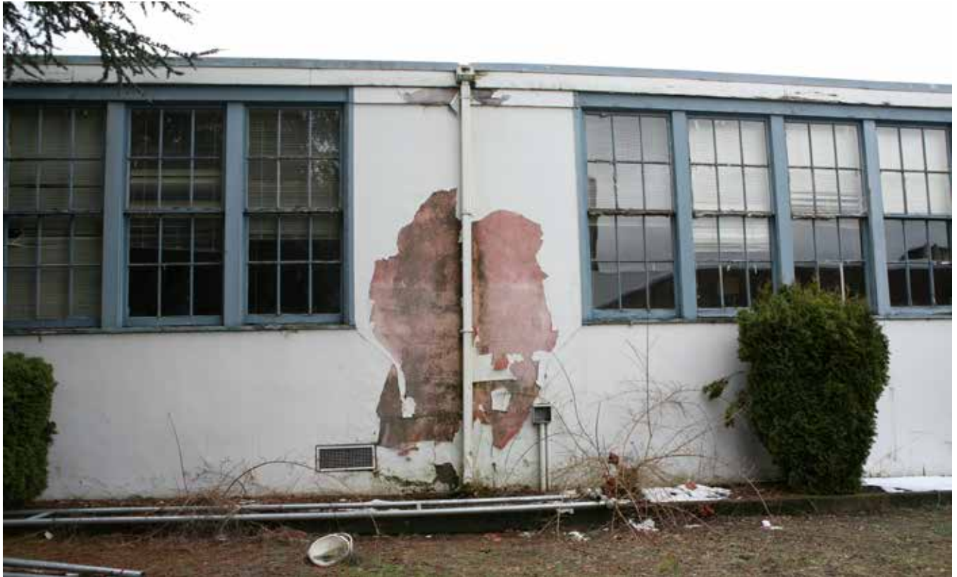
CP11. East facade (partial) of 1943 annex.
