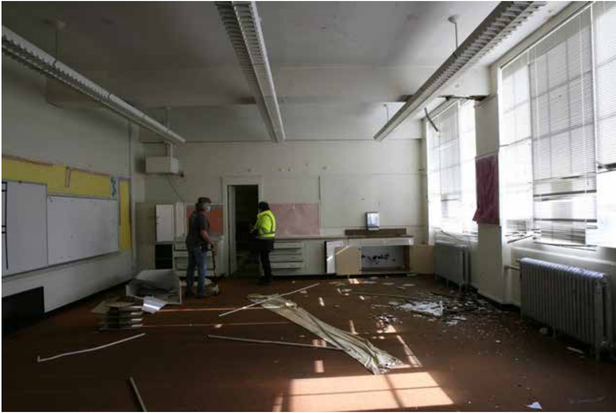
CP59. 2nd floor, Classroom 205. Looking east.
