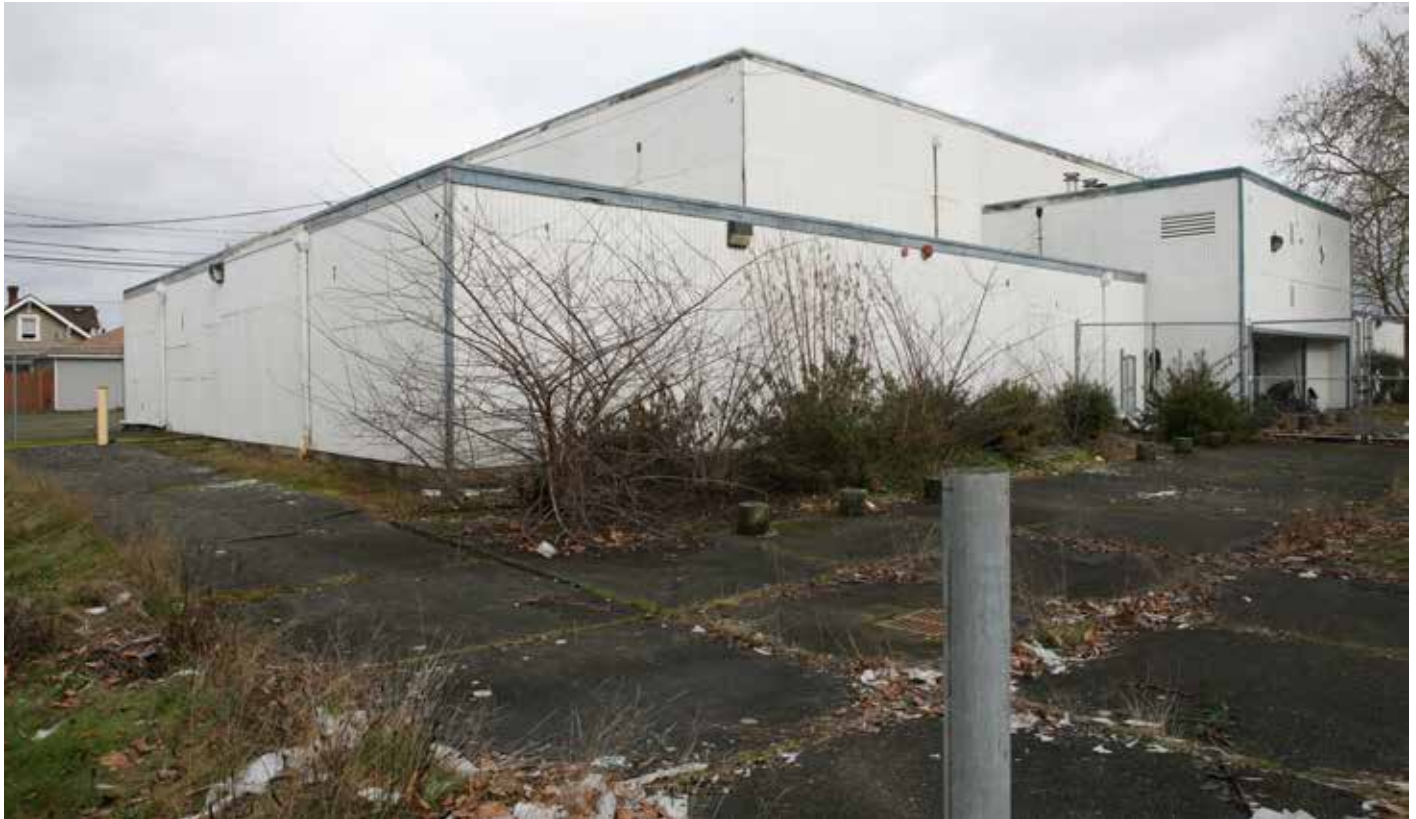
CP23. SW corner of Gym (1982), detached building on school parcel.
