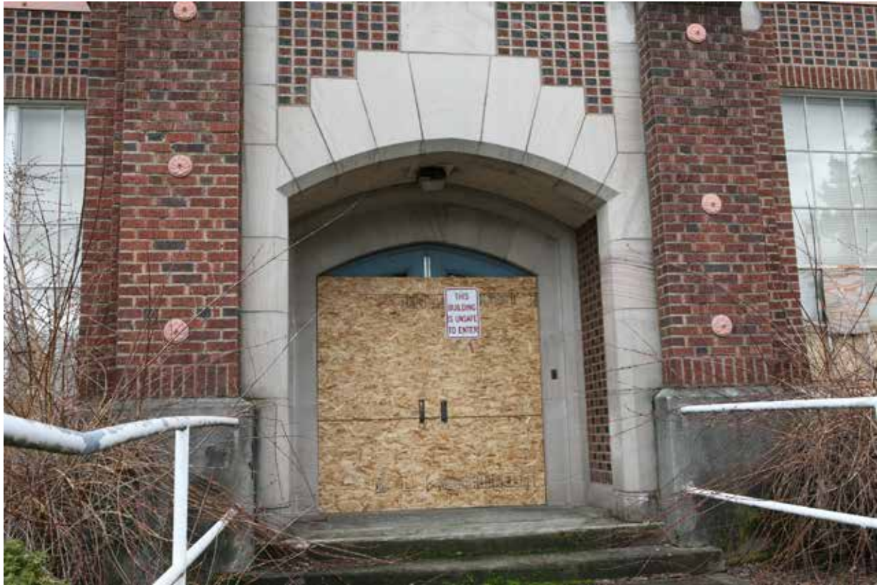
CP27. Detail, south facade, westernmost entry.
