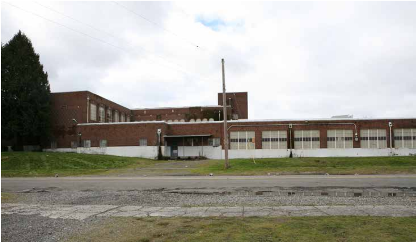
CP21. East facade of original building.
