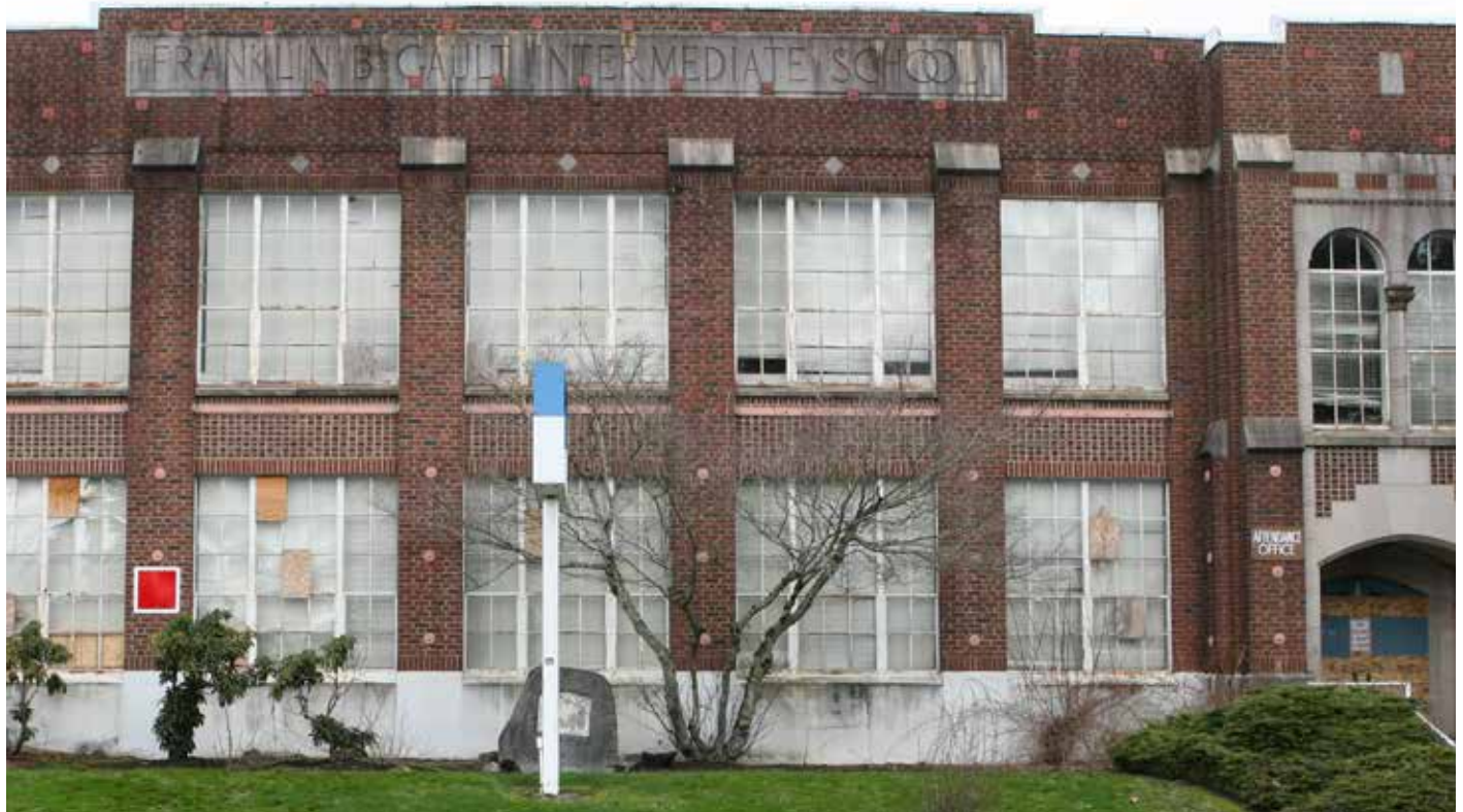
CP28. Detail, south facade. Note original signage/school name at top.
