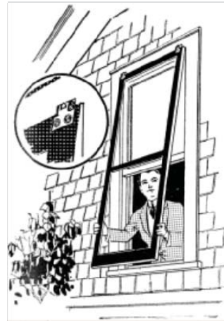
Above: Storm windows, held in place with a simple metal clip (still available at some hardware stores), maintenance of glazing compound and weatherstripping were the traditional way of improving thermal performance of windows. This is still a cost effective method in the Pacific Northwest climate.
