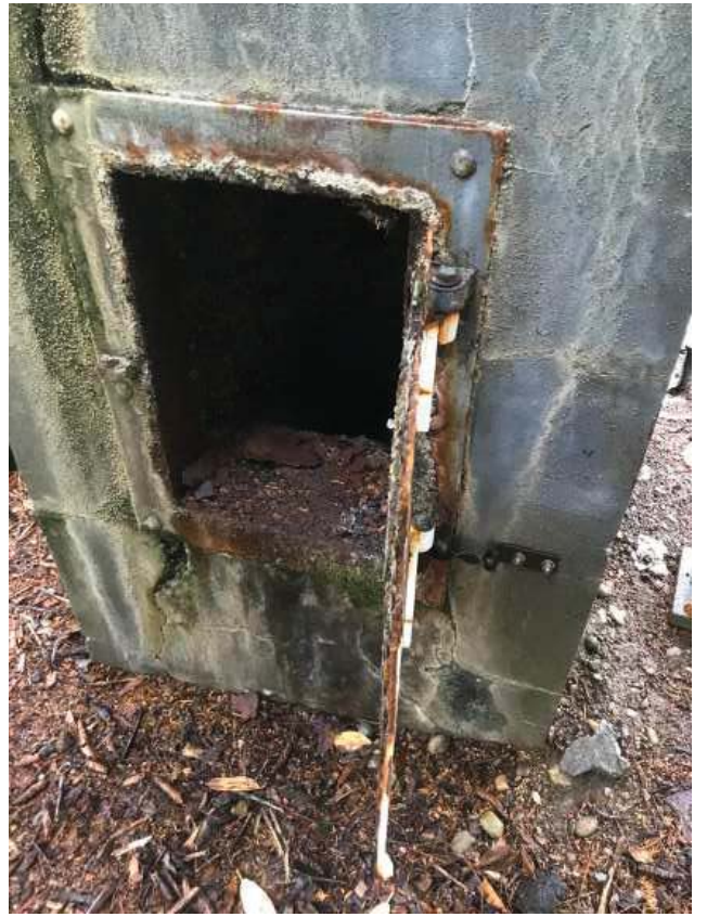
CHIMNEY AND DOOR
