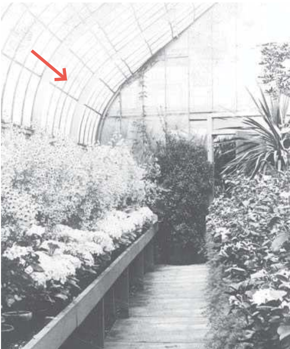
Historically, glass followed steel framing. Photo courtesy of Washington State Historical Society.
