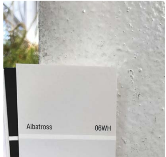
HIGH PERFORMANCE COATING (to match existing: used for all painted steel material during the restroom addition)
