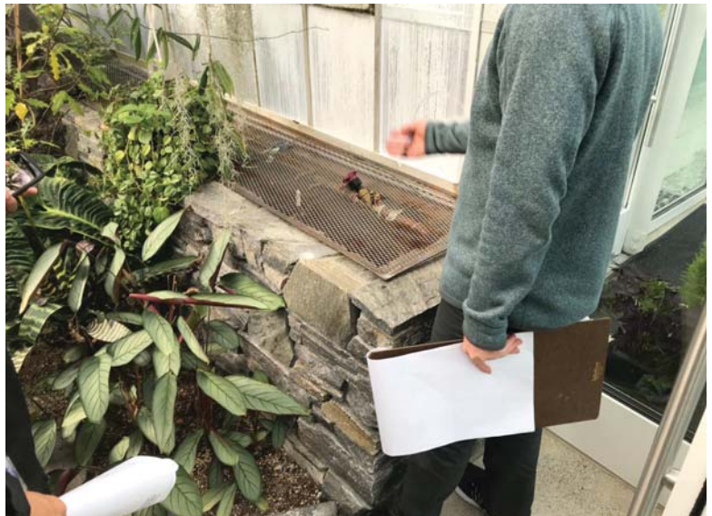
EXISTING STONE WALL (which replaced the slag walls, which contain hazardous/ heavy metals during the restroom addition)
