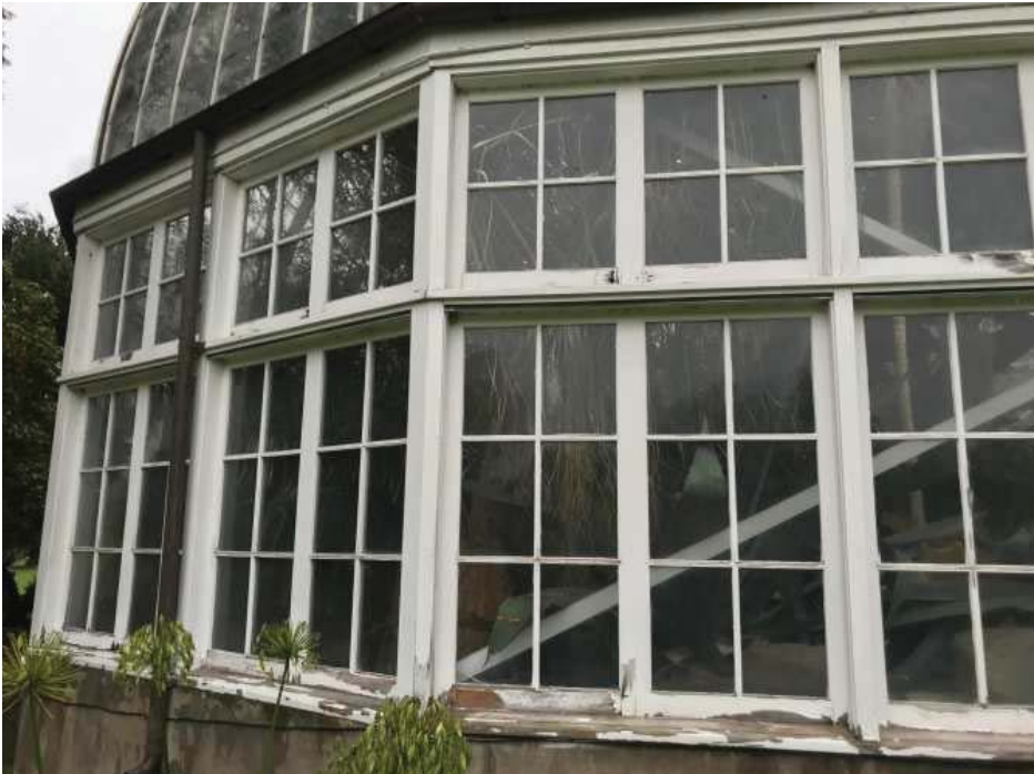
FIXED WOOD WINDOWS (west of the rotunda; previously replaced as part of the 1991 renovation)
