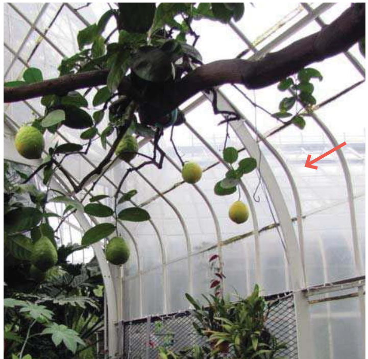
Today, glass curves away from the steel frame.
