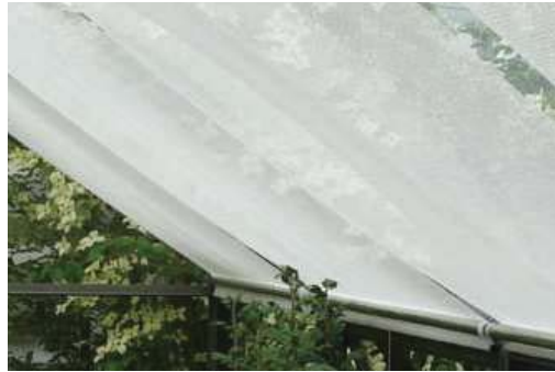
VINYL COATED POLYESTER SHADE FABRIC, WHITE (NOT SHOWN FOR CLARITY IN RENDERING BELOW, LOCATED AT ALL ROOF PLANES AT WINGS). FASTENED TO EXISTING STRUCTURAL WITH CLAMPS
