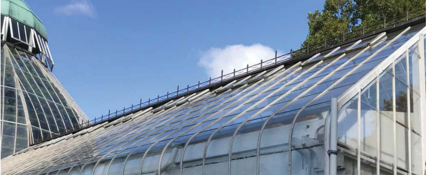
VENTILATOR WINDOWS (some, but not all, were replaced as part of the 2003 renovation)
