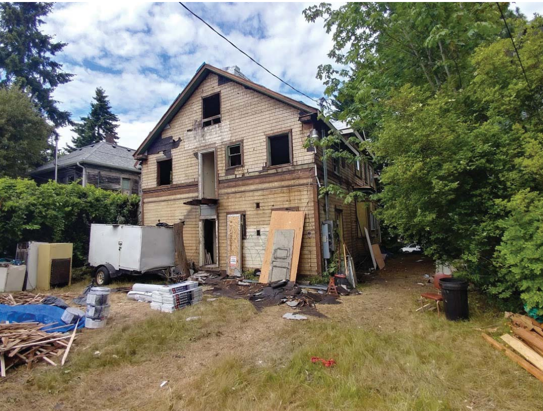
Front and rear of home after asphalt siding removed.
