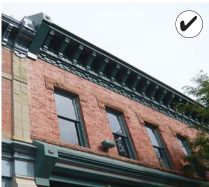
Maintain significant architectural details, including: projecting cornices, masonry patterns, decorative moldings, double-hung wood windows and other decorative features.
