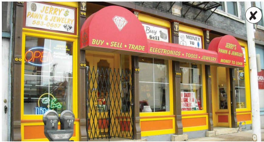
Do not design an awning to be of an odd shape that does not reference historic/traditional awnings, such as bullnose or bubble awnings.
