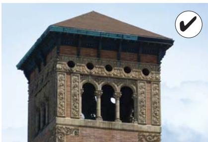
Maintain the traditional overhangs to preserve the shadows created, which contribute to the perception of the building's historic scale.
