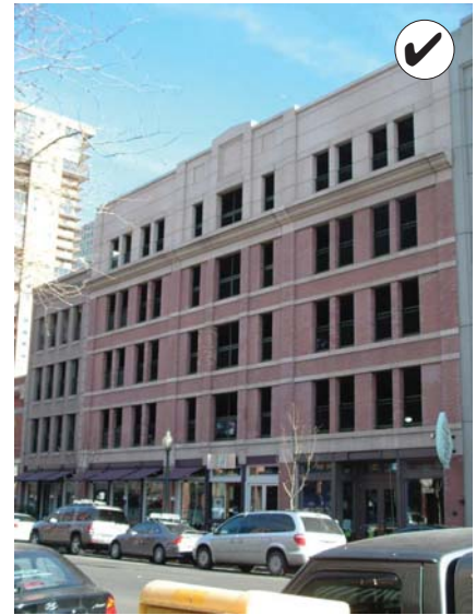
Design a parking structure to be compatible with the mass and scale of historic buildings in the District.
