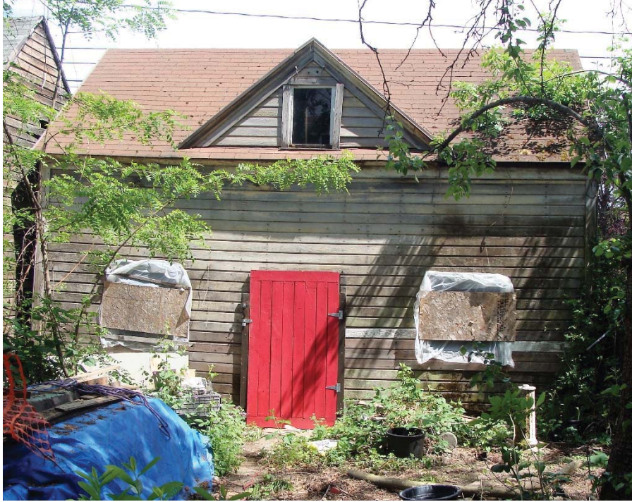
Figure 7. West façade of stable.
