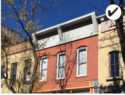
Design a simplified interpretation of a historic cornice if evidence of the original is missing.
