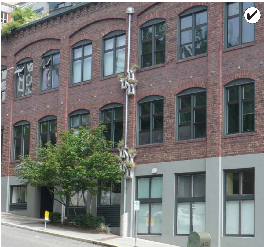
Step the first floor of a building along a sloped street to maintain a constant street presence.
