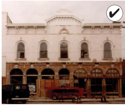
During rehabilitation (ca. 1982)
