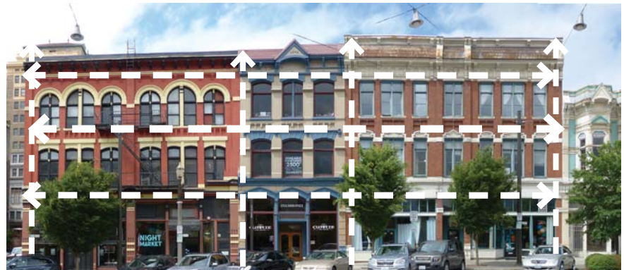
The Old City Hall Historic District context is defined by consistent patterns of building setbacks, alignments, fenestration and materials.
