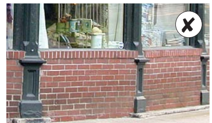
Do not cover or alter significant architectural details, such as kickplates.
