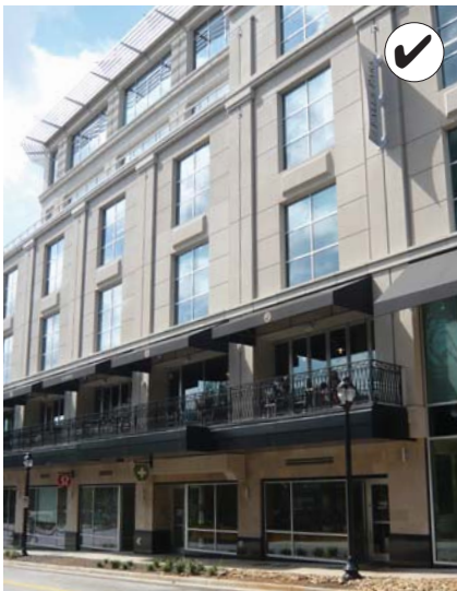
Align window moldings, tops of display windows, cornices, casings and parapets at the tops of buildings, where possible.
