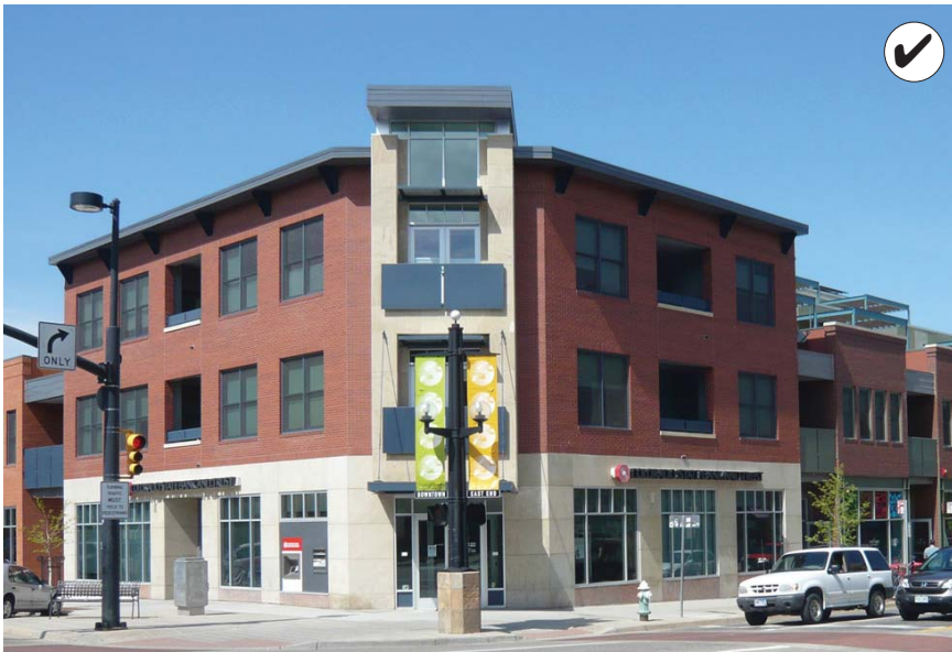
Use floor to floor heights which appear similar to those of traditional buildings.
