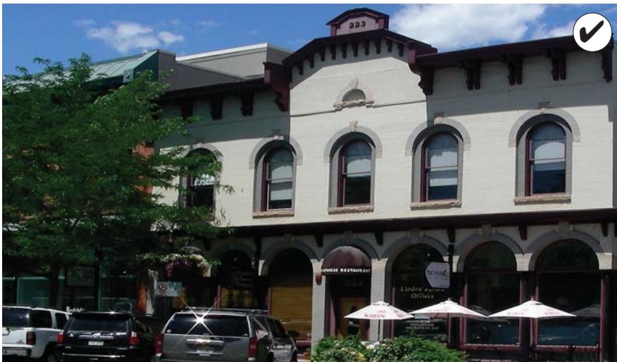
After rehabilitation. Using historic photographs, a cornice was constructed to match the original in character. An alternative material (wood) was used instead of the historic metal. (ca. 2013)
