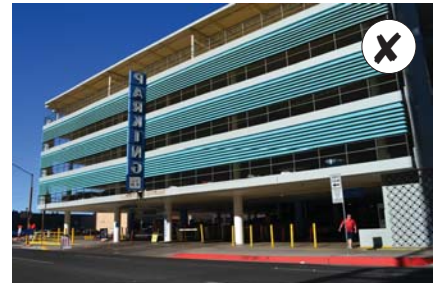
Screen the upper levels of a parking structure to minimize the visual impacts of parked cars on the street and sidewalk.
