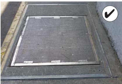
Retain and maintain historic grates and service doors in the District.
