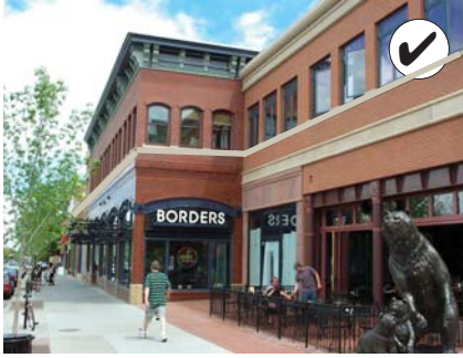
Align window moldings, tops of display windows, cornices, casings and parapets at the tops of buildings, where possible.
