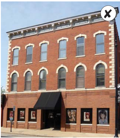
Do not alter the size and shape of a storefront opening, as seen above.
