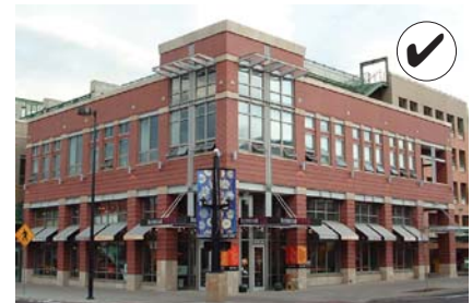
Use vertical and horizontal articulation techniques to reduce the apparent mass of a larger building and to create visual interest.
