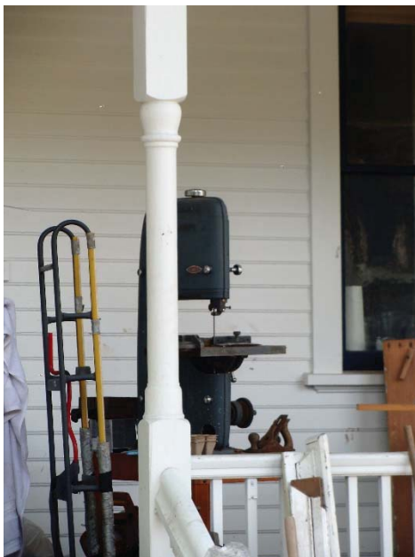
Figure 6. Detail of original porch post and balustrade
