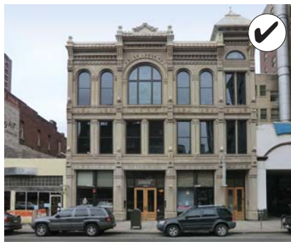
The rooftop addition shown above is set back from the primary façade to be minimally visible from the public street and sidewalk.
