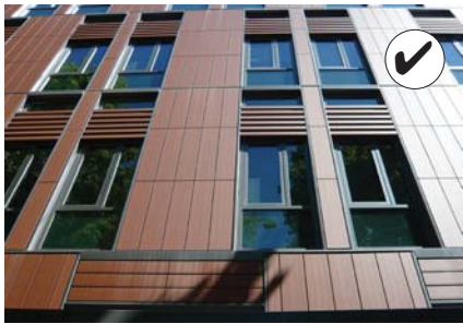
Use a ratio of solid-to-void (wall-to-window) that is similar to that found on traditional commercial structures.
