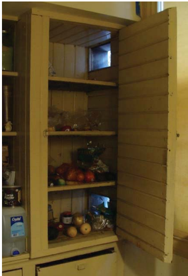
Figure 2. The cooling cabinet in the kitchen pantry. Note the exterior openings for ice delivery.
