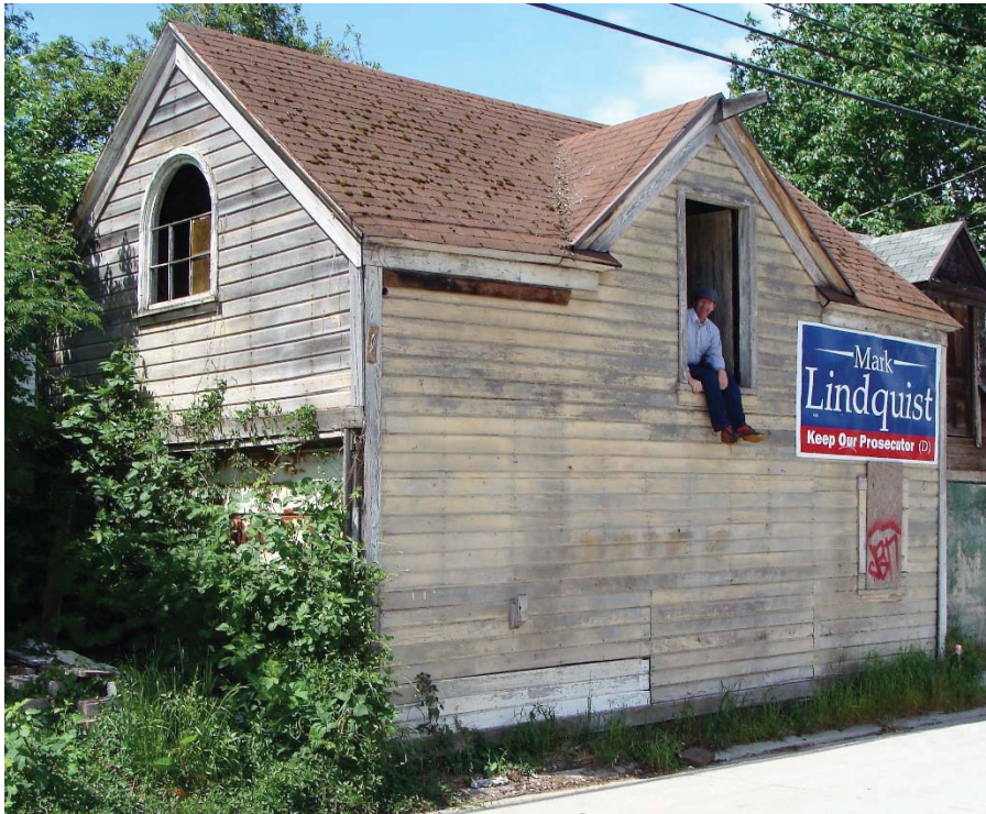
Figure 8. East (rear) and south facades of stable with current owner in loft. Note the barely discernible outline of the filled-in stable entrance below his feet. The auto entrance on the south façade is barely visible. The arched window was installed in the 1980s.
