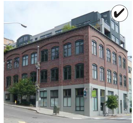
Incorporate a base, middle and a cap in the design of a new building to reinforce the visual continuity of the District.
