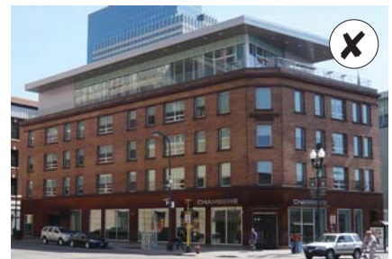
An addition to the rooftop of a building may be considered if it preserves the perception of the historic scale of the building.
